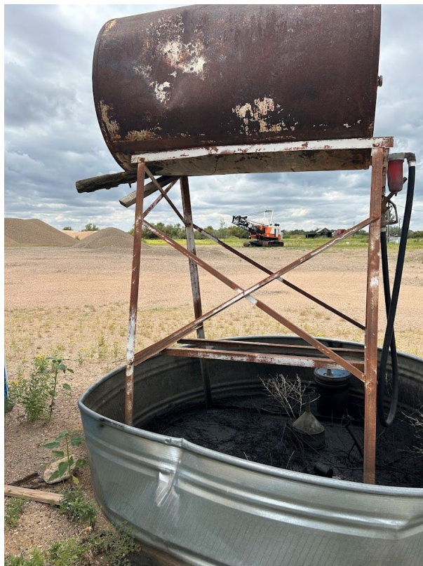
Photo 10: View of a storage tank within a horse trough, with observed hydrocarbon staining and odor, facing west.
