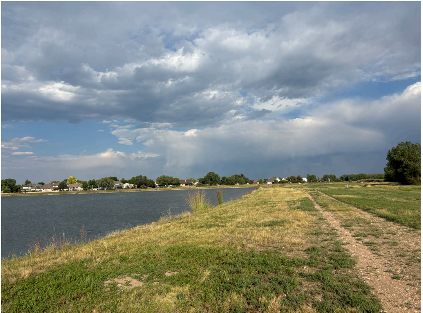
Below – dead weeds sprayed recently, north side of Pond 3 looking east
