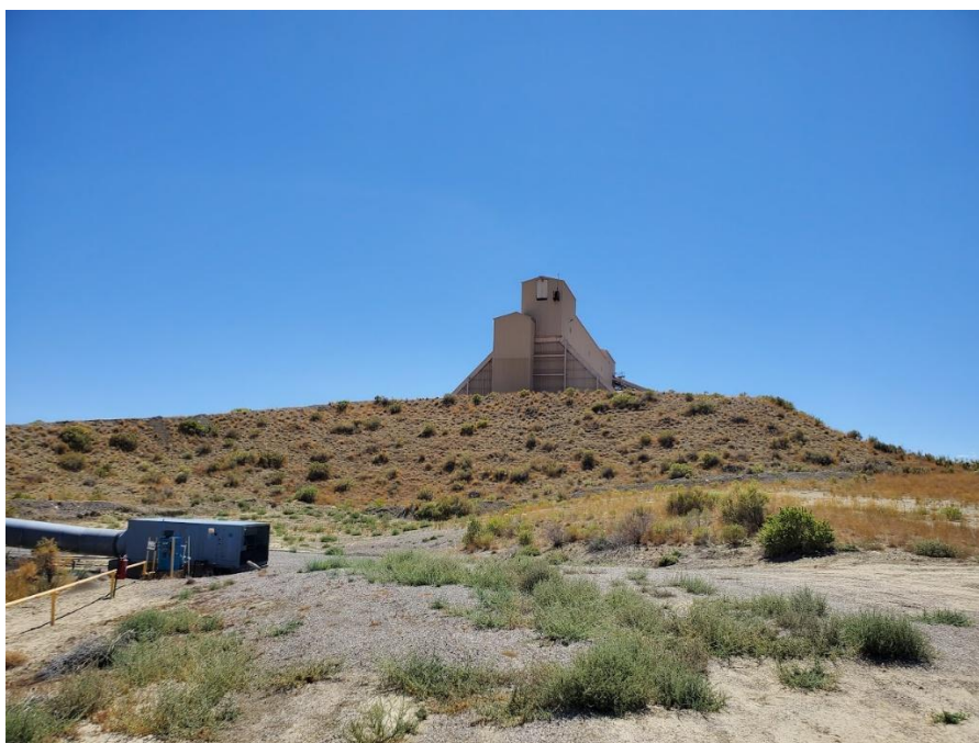
Photo 14: View to the north of animal burrow in the RP-5 embankment.
