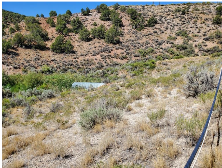
Photo 3: View to the southwest of the embankment
