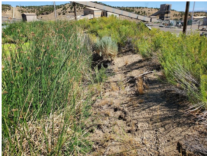
Photo 5: View to the north of the eastern embankment of the PP-2 Pond.
