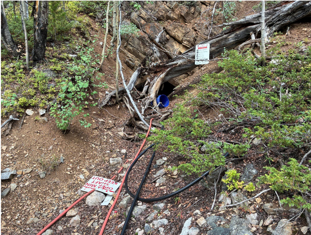
Photo 5- Portal located behind the tree stump. The mound of dirt in front keeps water in the mine.
