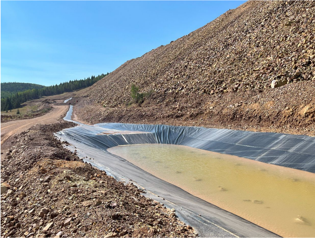
Photo 3: Seep 3/4. Note little to no process water from seepage appears to be contained within it at the time of inspection.
