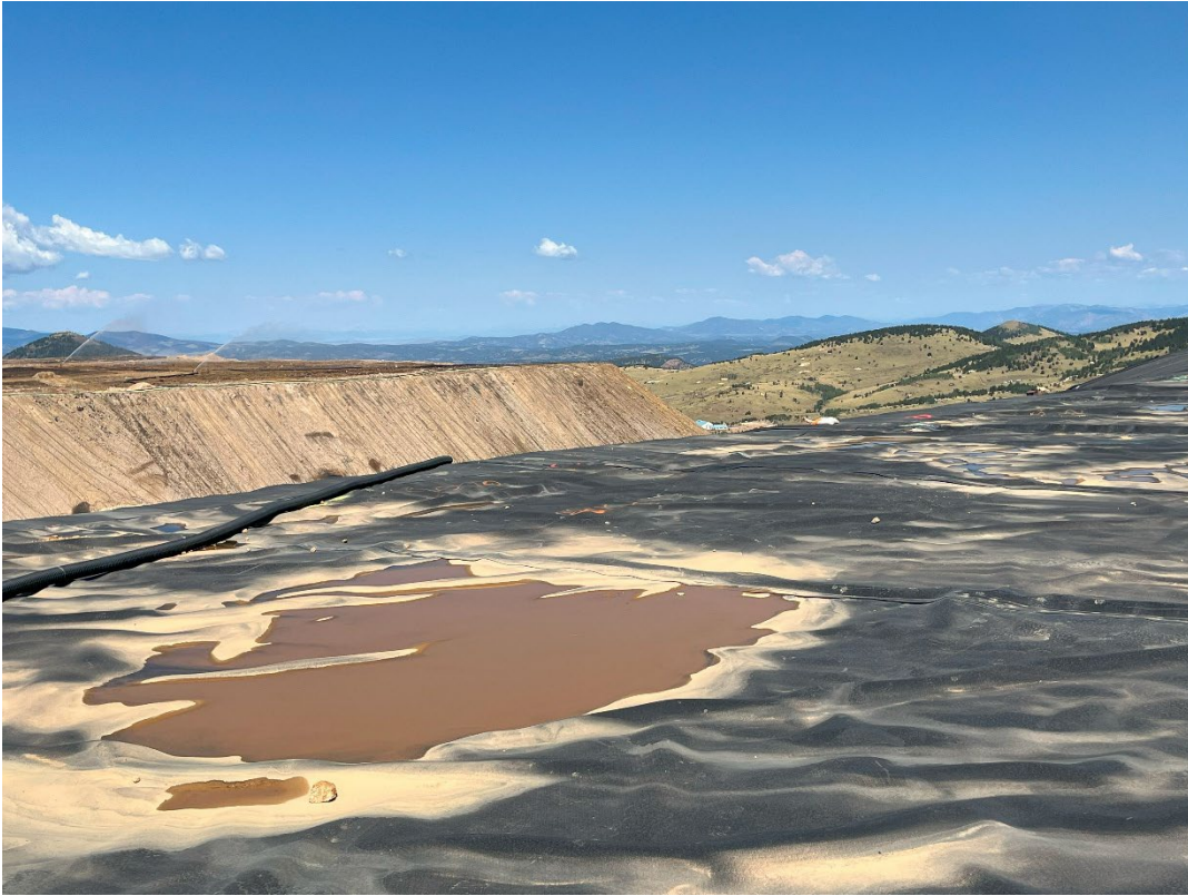
Photo 7: Recently installed liner area. Note minor ponding due to recent rainfall.
