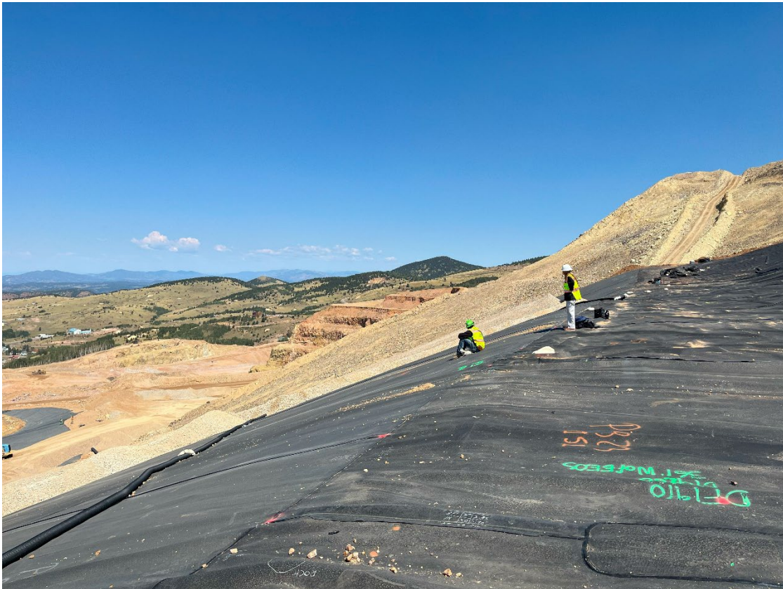
Photo 9: Newfields representatives performing QA monitoring of liner install.
