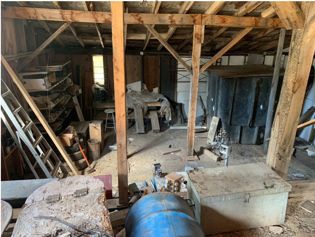
Photo 2 – Shop area inside Mill building.
