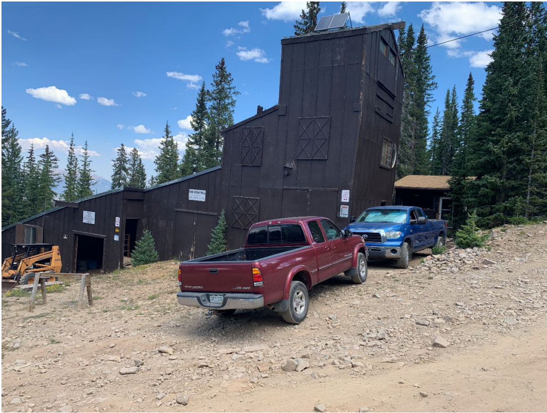
Photo 1 – Mill building adjacent to forest service road.
