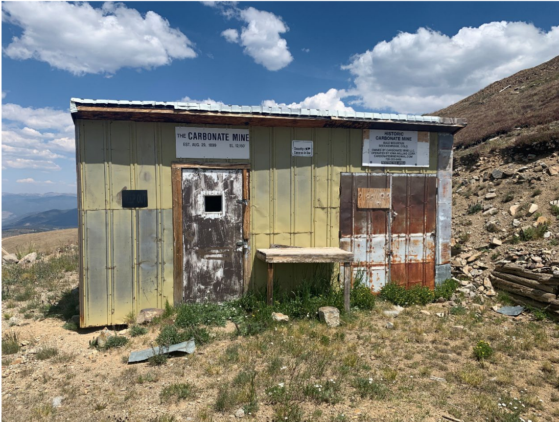
Photo 3 – Steel building and pad area at the Carbonate Mine.
