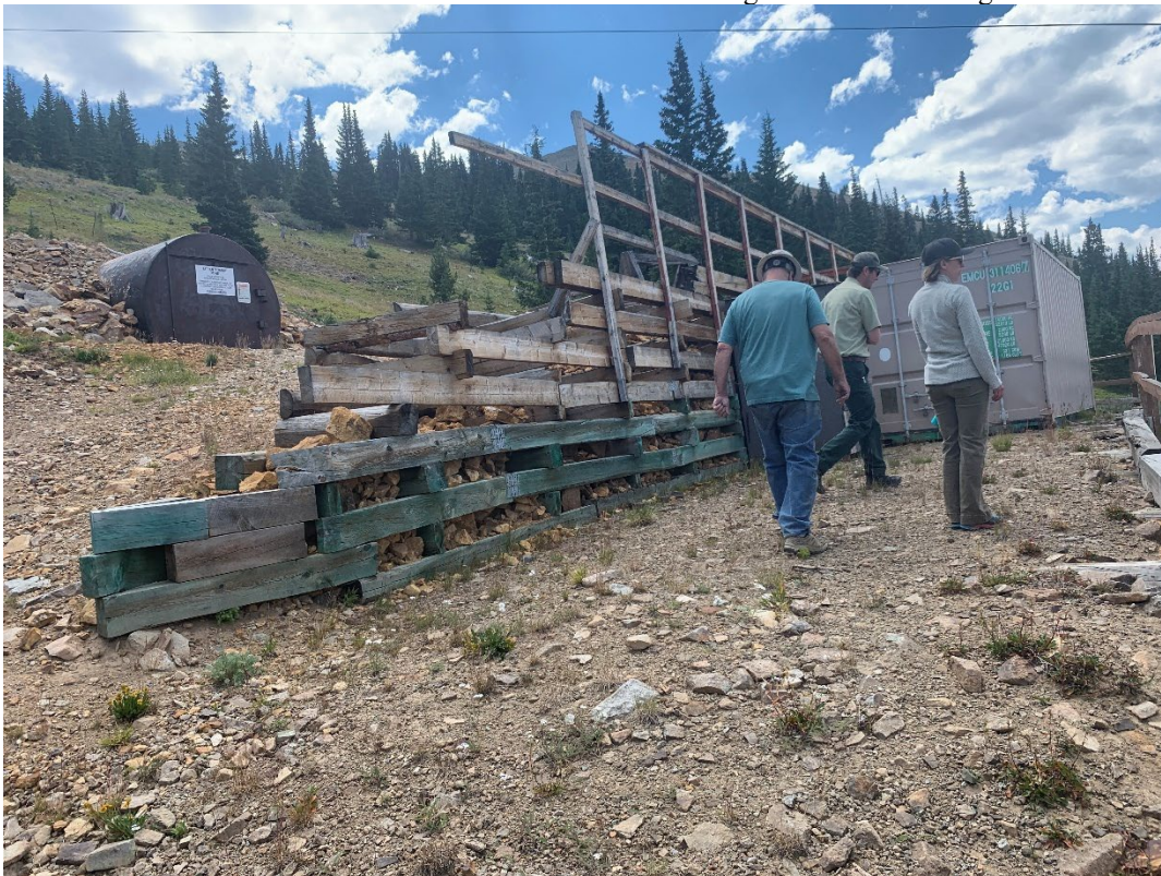
Photo 2- Cribbing structure below mine portal and Conex box.
