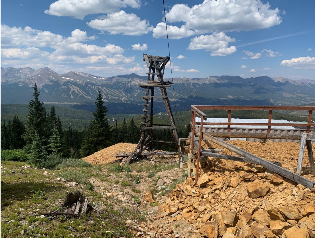
Photo 3- Historic tram tower with cable on south side of waste pile.
