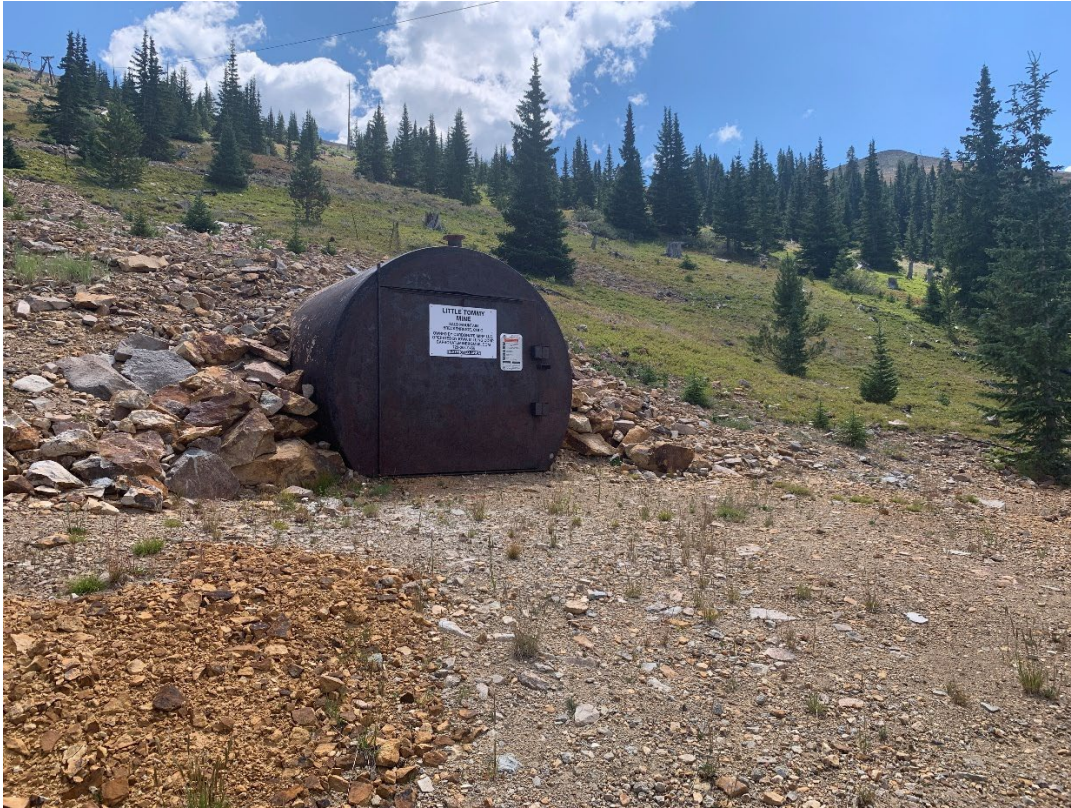
Photo 1- Portal entrance is well secured with no signs of water discharge.
