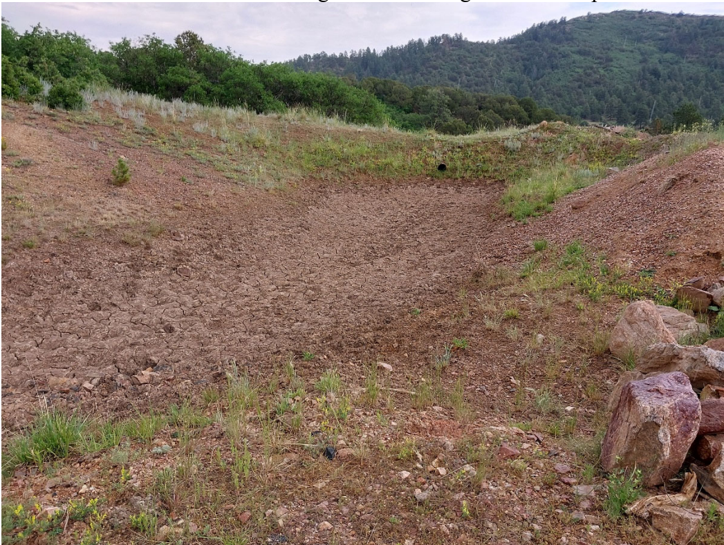
Photo #6: View of the settling pond and the culvert directing storm runoff to the natural drainage.
