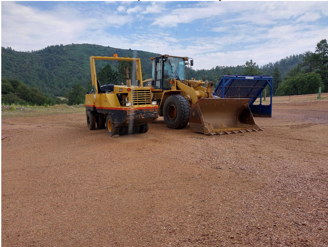
Photo #4: Stored equipment on site.
