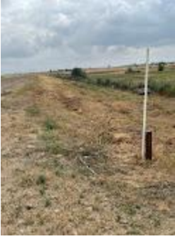
2025.08.25.Pit 29.near main gate for reservoirs.AFTER.jpg 116K
