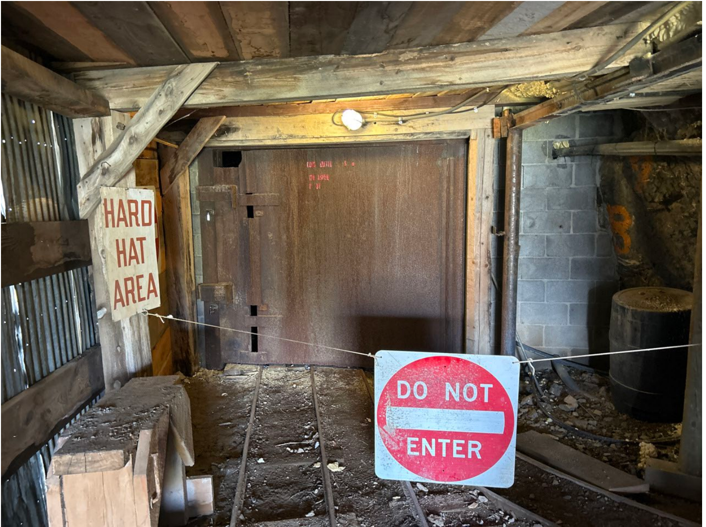
Figure 9: Portal entrance, secure.
