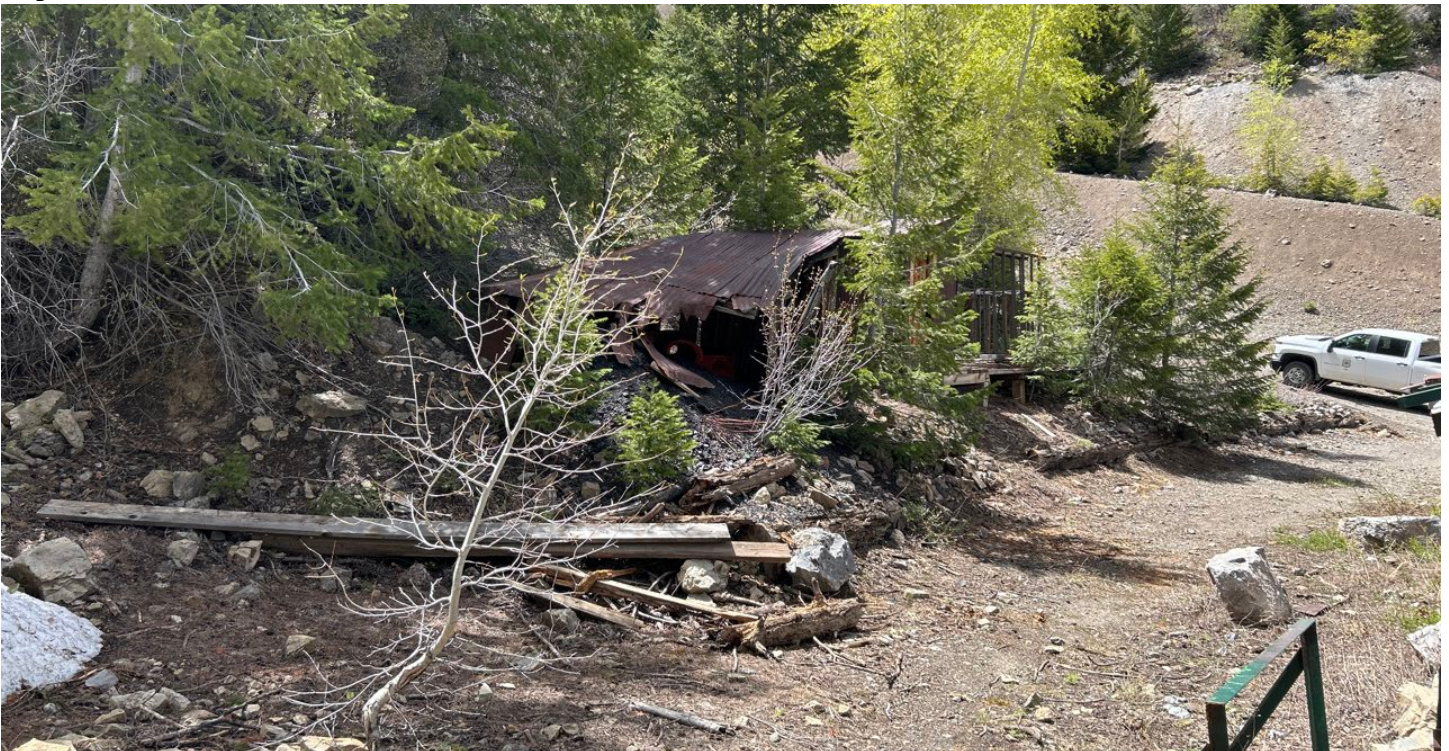
Figure 5: Outhouse area, maintenance work in progress
