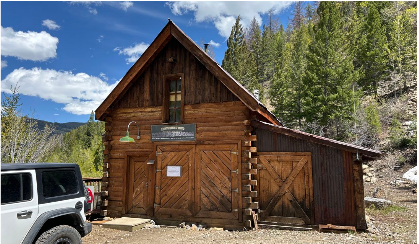
Figure 3: Locked cabin, front (west side)
