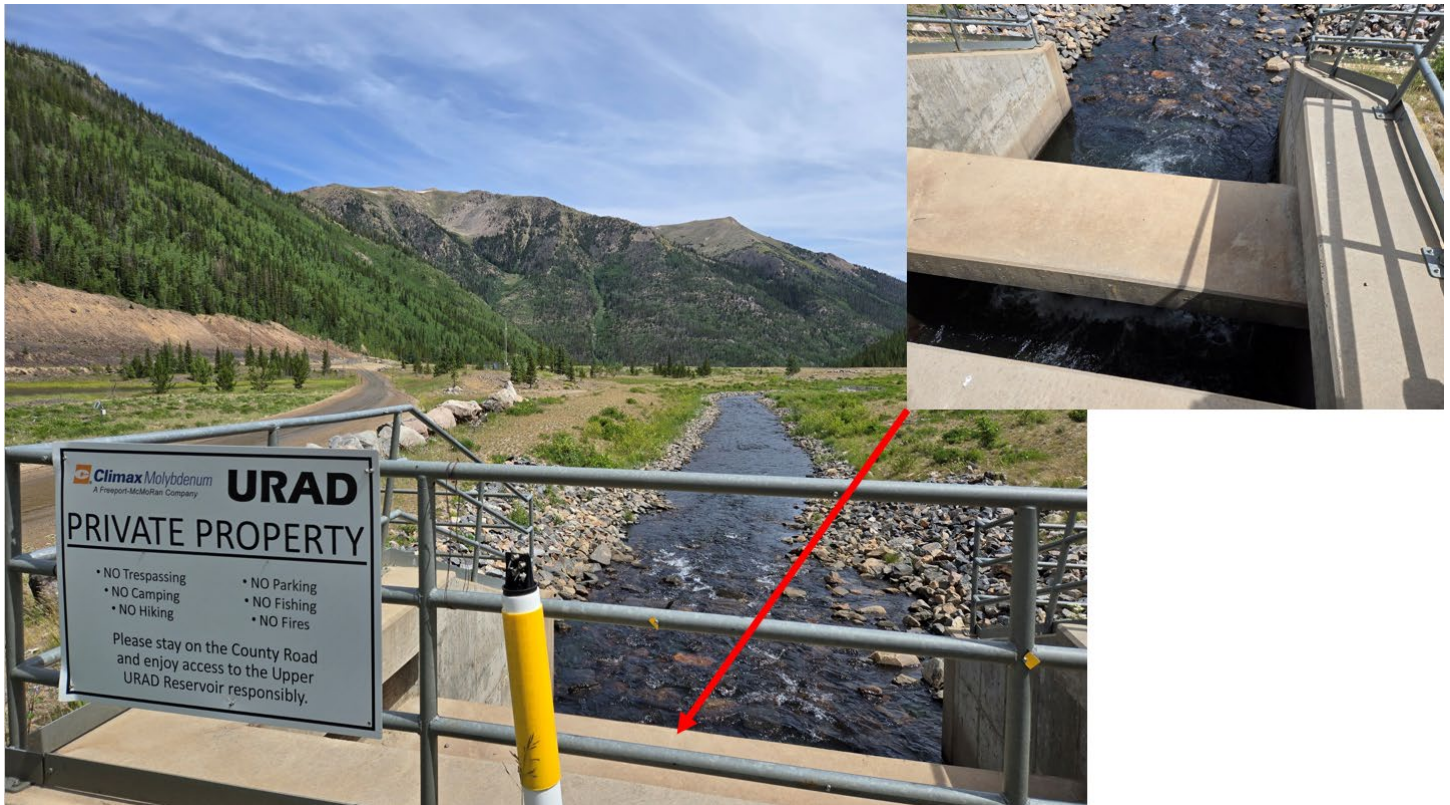
Photo 13: Point where the treated water from the URAD facility discharges into Woods Creek.
