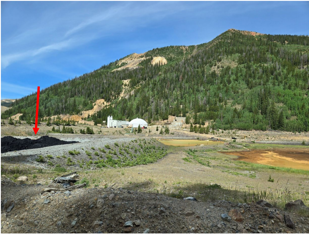
Photo 2: Looking west at external ponds at the URAD water treatment plant. The arrow points to Sludge Pond 2 where sludge was drying at the time of the inspection.
