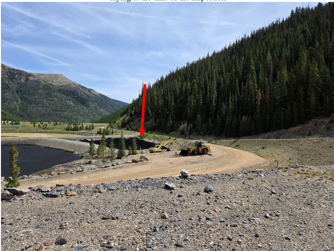
Photo 3: The red arrow points to Sludge Pond 2 where sludge was drying during the inspection. On the west side of Sludge Pond 2 is Sludge Pond 1, where sludge was being deposited during the inspection.
