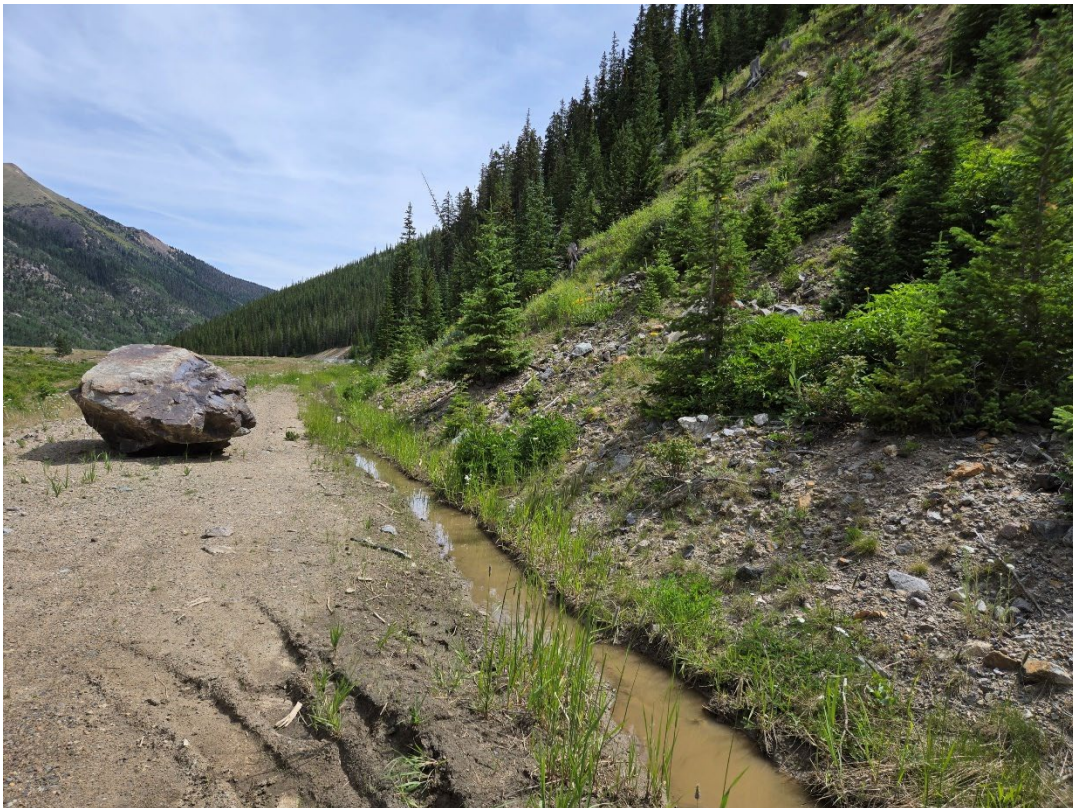
Photo 11: Looking north along the diversion ditch on the west side of the road leading to the URAD facilities.
