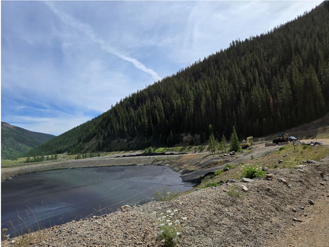
Photo 4: Looking east at Sludge Pond 1.
