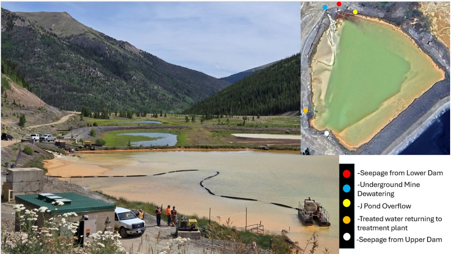
Photo 6: The color-coded circles, located on the image on the right, indicate inlet and outlet sources around Treatment Pond 1.
