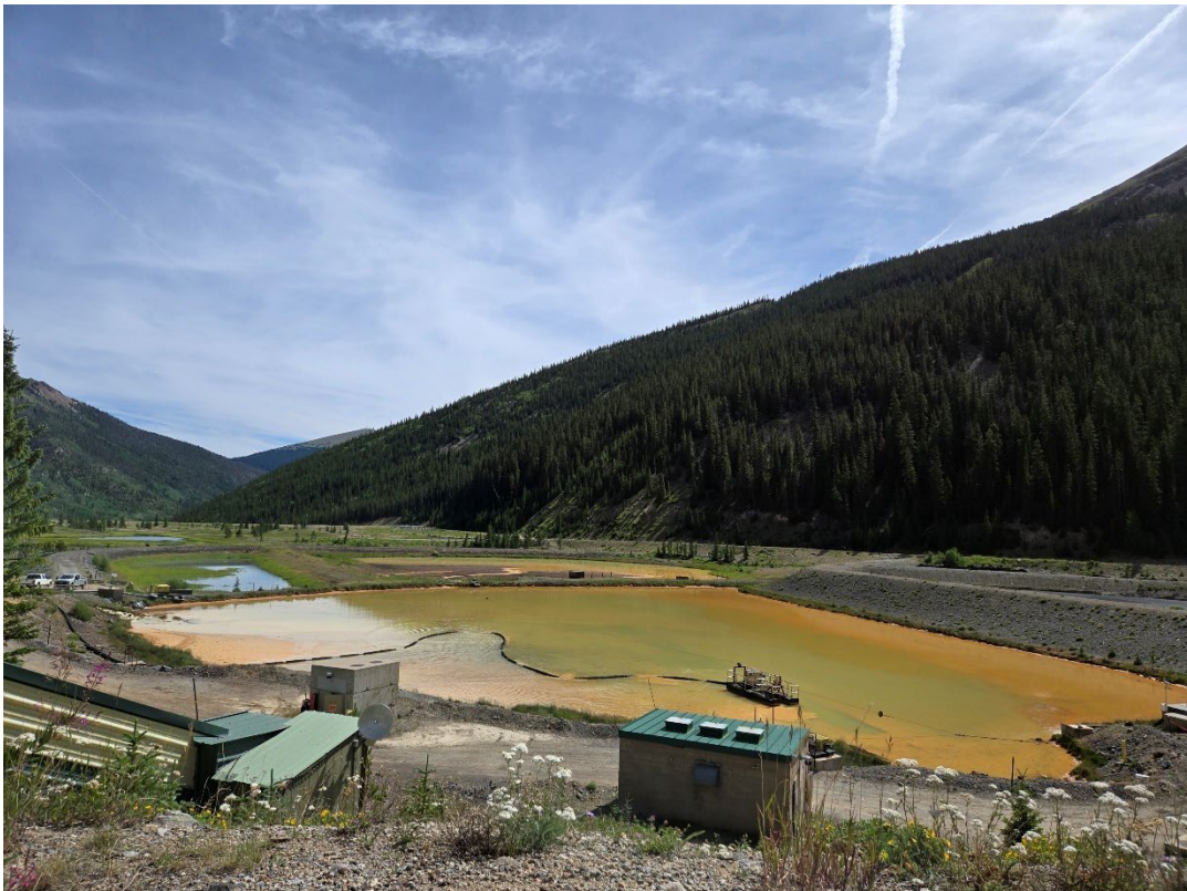
Photo 5: Looking east at the external Ponds at the URAD treatment plant. Treatment Pond 1 was being dredged at the time of the inspection.
