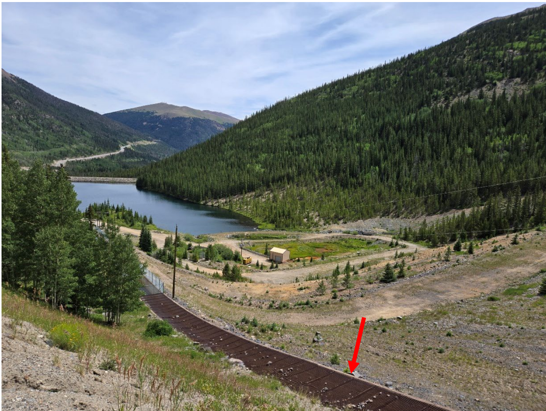
Photo 15: Looking north at the lower tailings dam and the Lower URAD Reservoir located on the north side of the URAD treatment facility. The arrow points to the channel connected to the box culvert within the berm on the southside of the URAD facilities, installed to divert emergency overflow.
