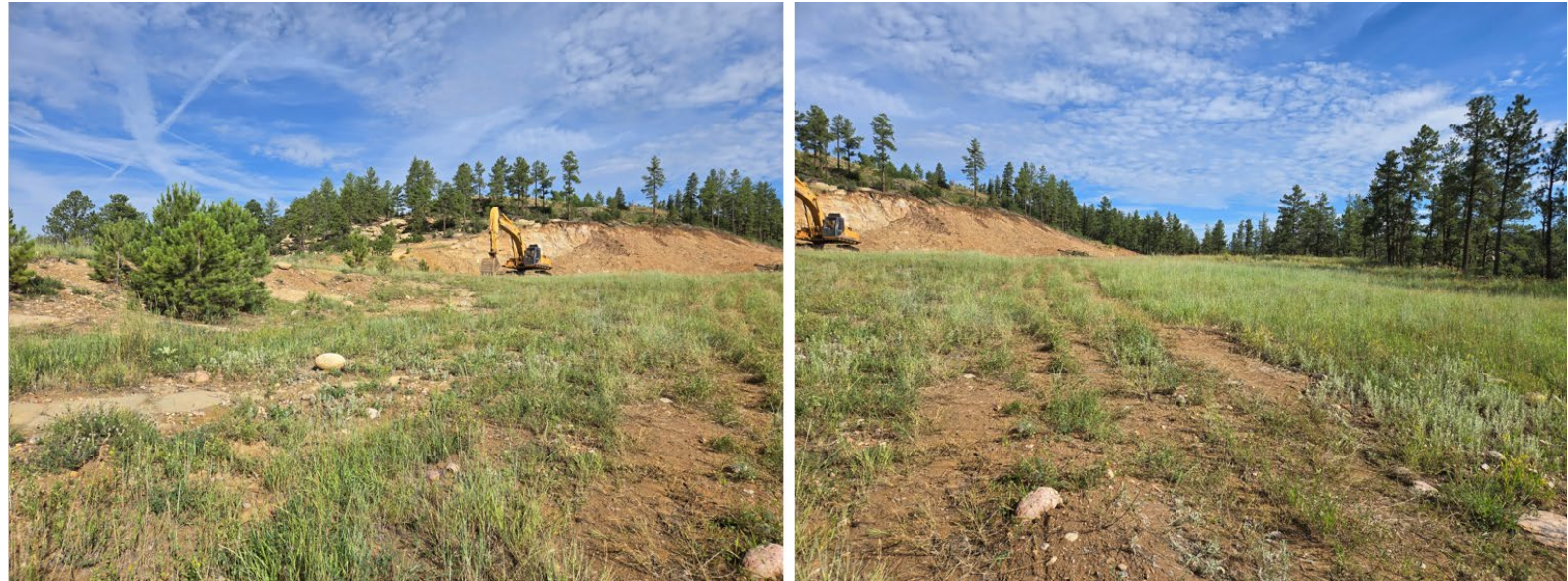
Photo 1: Looking northwest at the lower shelf area. The excavator highlights the recent backfilling and grading work done along the highwall separating the upper and lower shelves.
