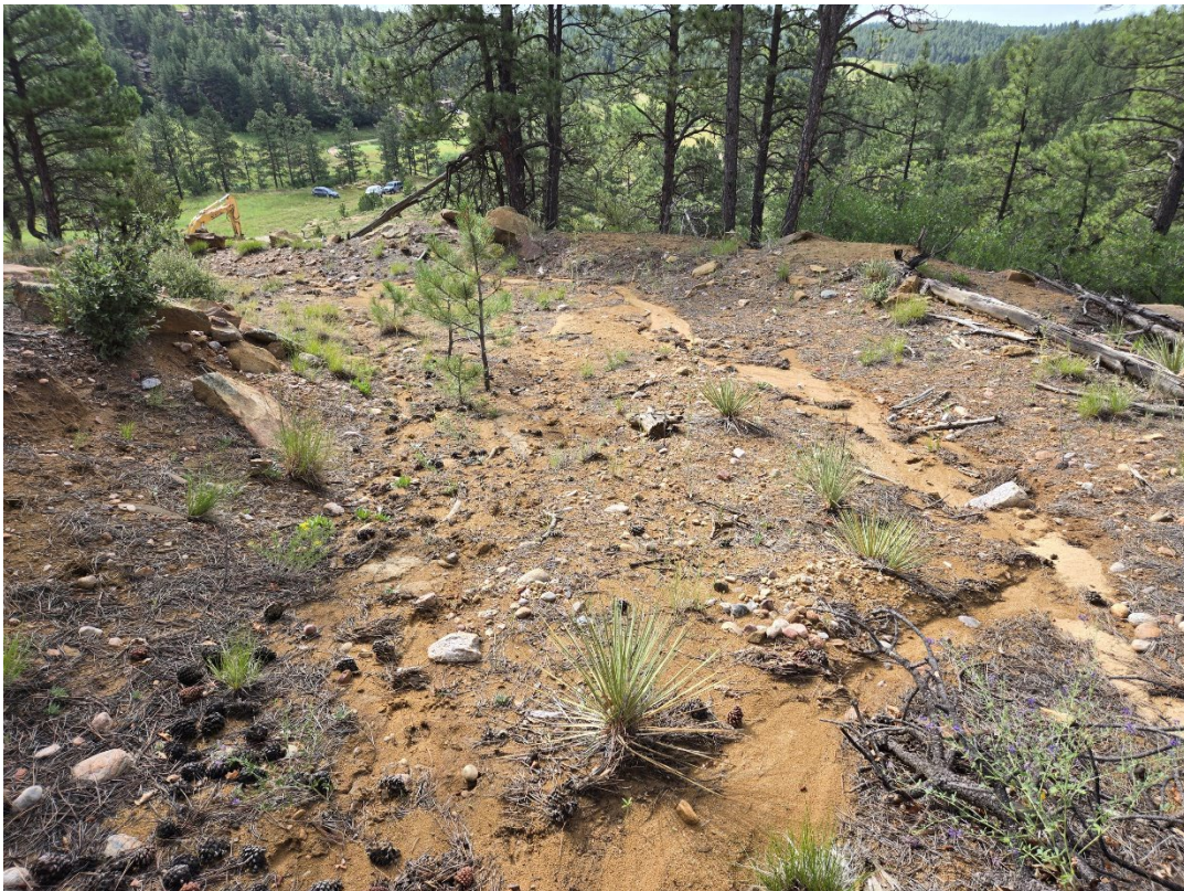
Photo 10: Looking at where sediment accumulation from stormwater runoff is contained onsite through the use of perimeter berms.
