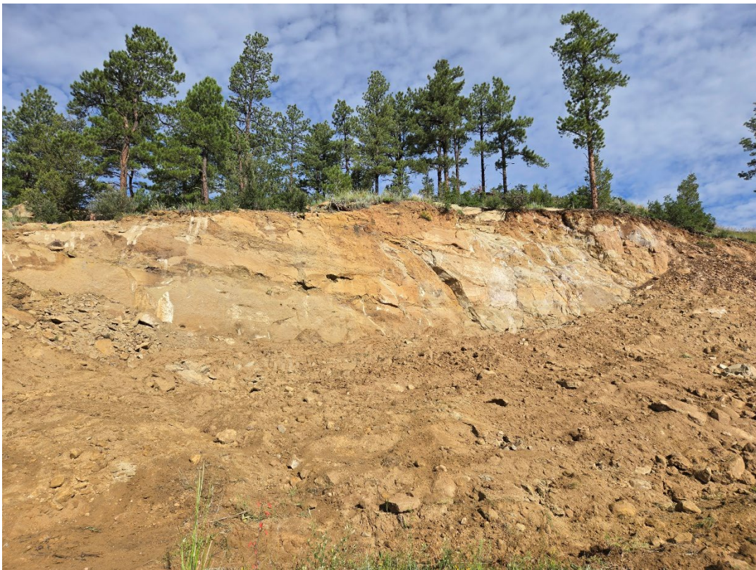
Photo 2: All that remains of the highwall that needs to be graded to a 3H:1V slope.
