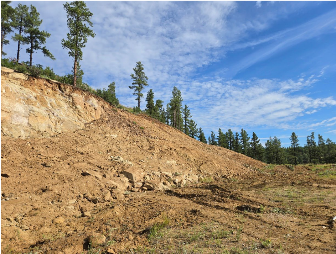
Photo 3: Looking north at a section of highwall that has been graded to a 3H:1V.
