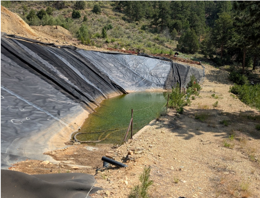
Photo 9: Looking at the out of compliance liner system in tailings storage impoundment. The liner is loose and damaged and will need to be repaired and re-certified before milling resumes.
