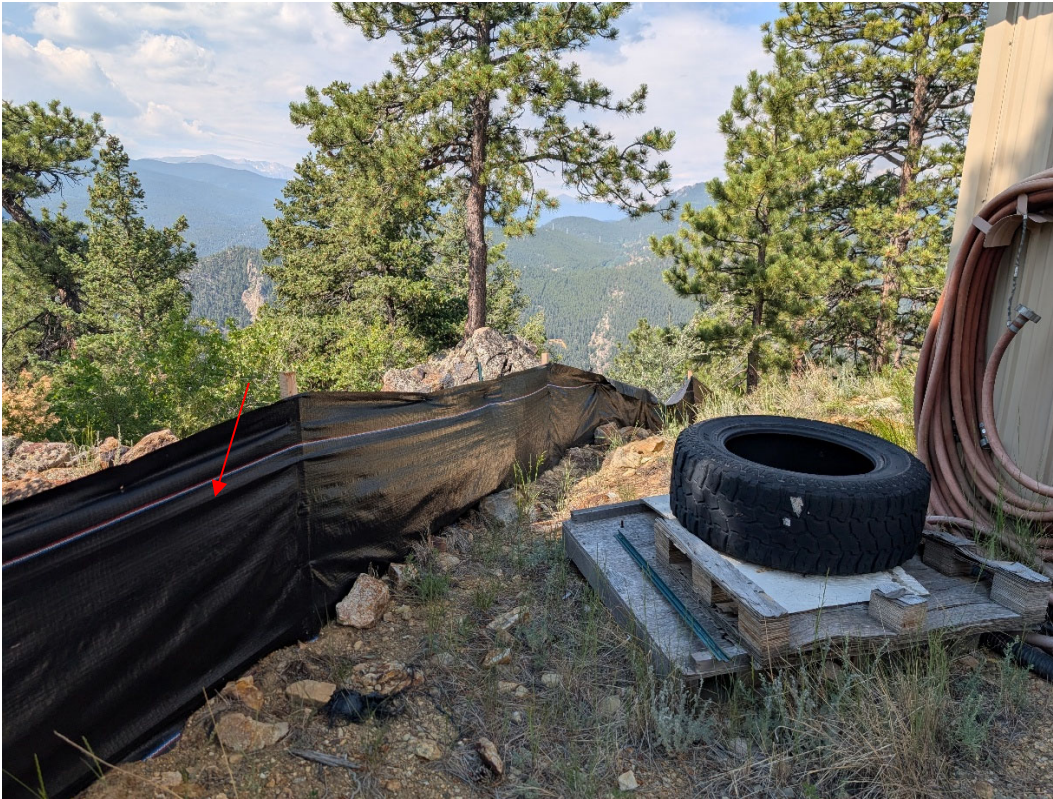
Photos 5 & 6: Silt fence reinstalled along the perimeter of the mill area.
