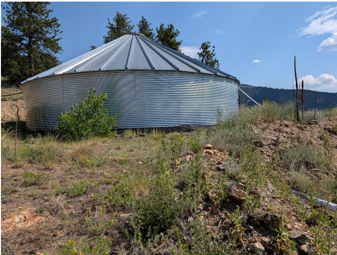
Photo 4: The 65,000 gallon water tank installed north and above of the mill.
