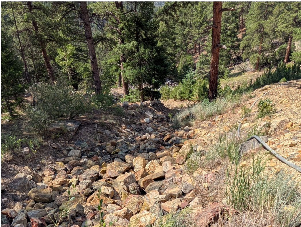
Photo 12: Looking at the stormwater diversion channel on the east side of the tailings impoundment area.
