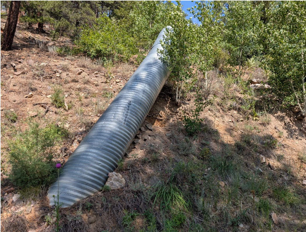
Photo 11: Looking at the stormwater diversion pipeline on the west side of the Tailings Impoundment Area.
