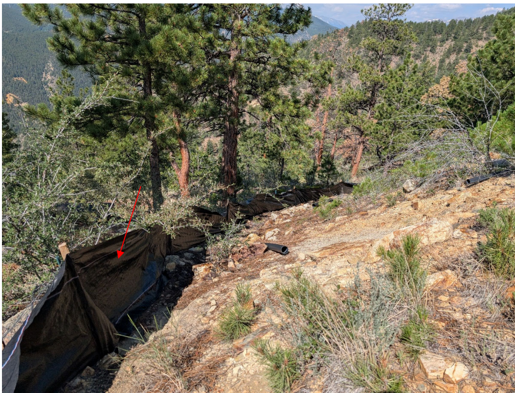
Photos 5 & 6: Silt fence reinstalled along the perimeter of the mill area.
