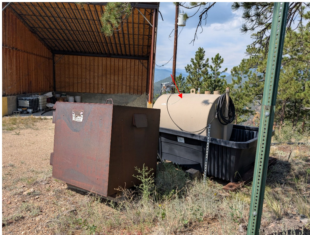
Photo 8: Fuel tank stored inside a containment vessel.
