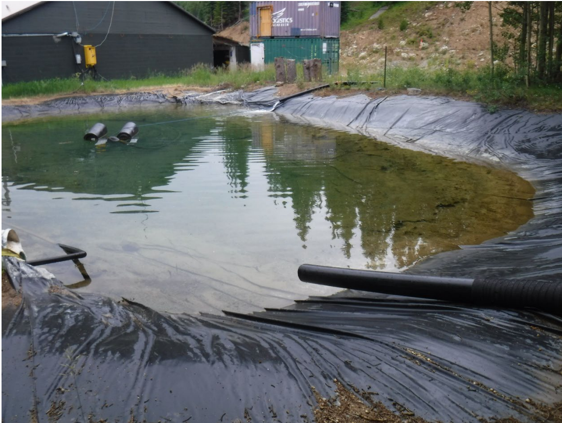
Photo 9: Pond 1, discharge in background is from the Joliet Raise and the pipe in the foreground is for Idaho Tunnel effluent direct discharge to pond
