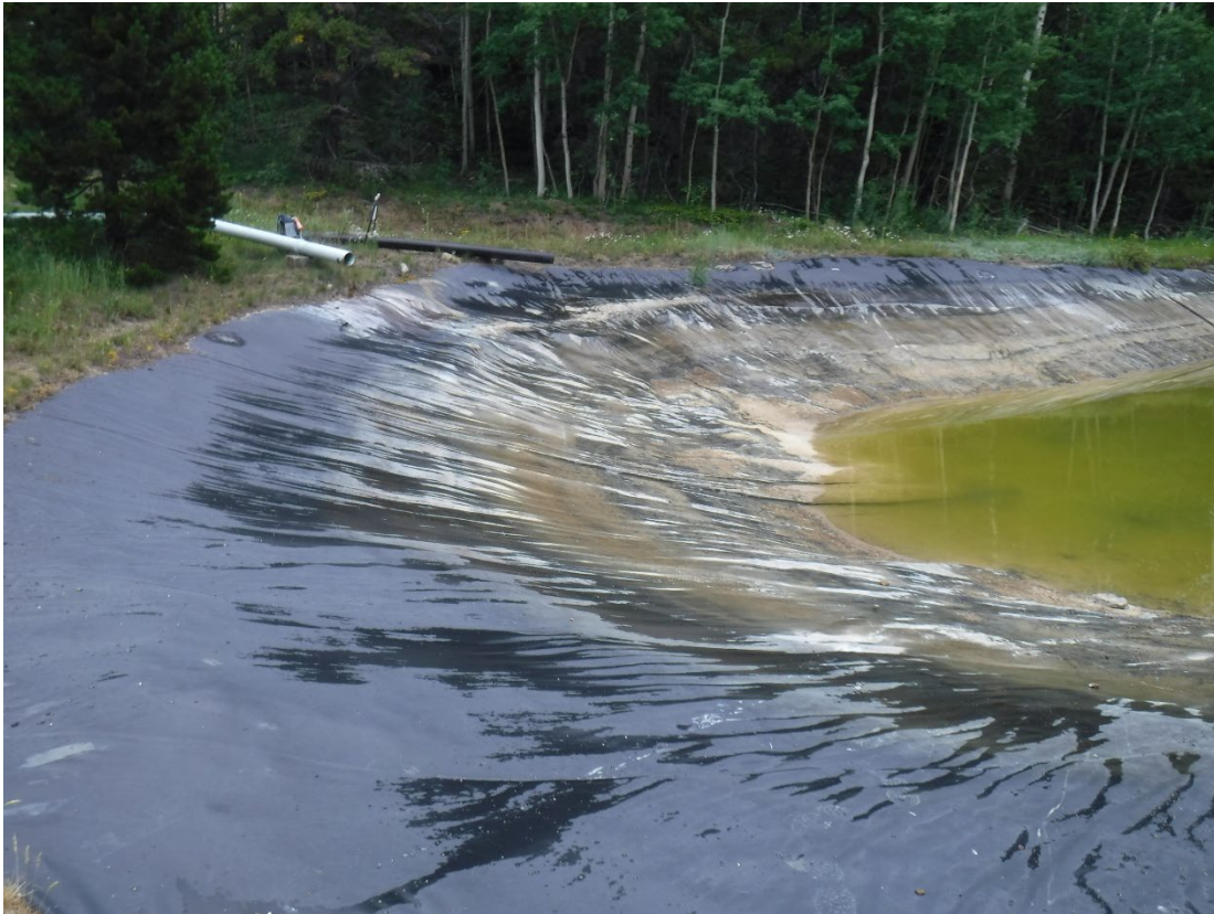
Photo 11: Back flushing discharge pipe from Pond 1 going to Pond 2, and black pipe from Idaho Tunnel
