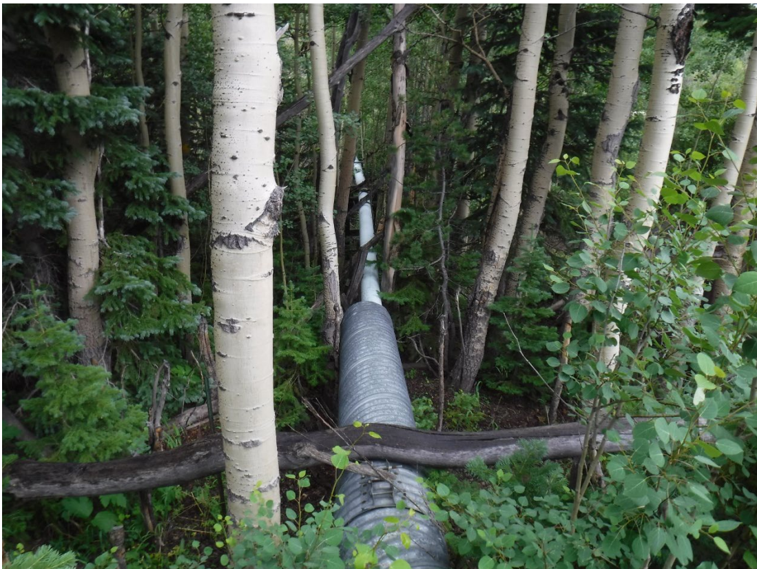
Photo 10: Back flushing discharge pipe from Pond 1 going to Pond 2
