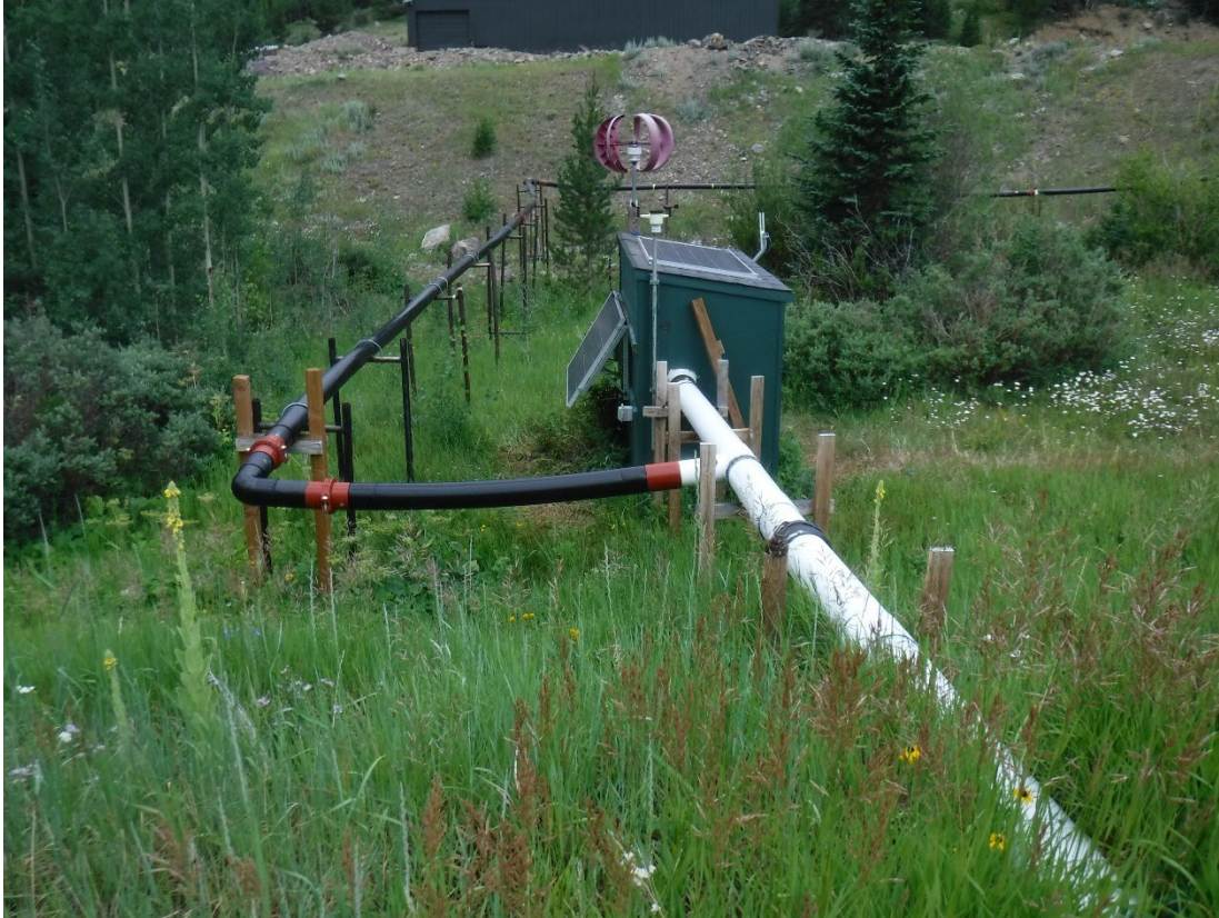
Photo 13: CDPHE approved discharge location, black pipe is from water treatment plant white pipe not used from Pond 2
