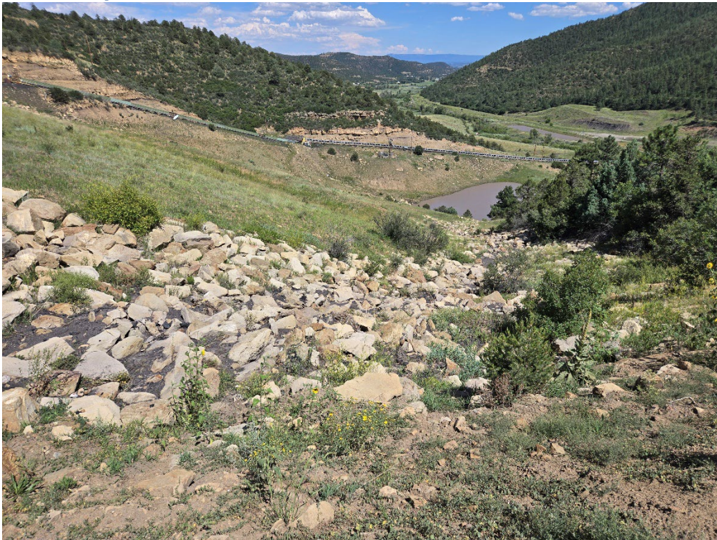
Photo 28: Sediment accumulation within the rock lined channels around the reclaimed portions of the RDA.
