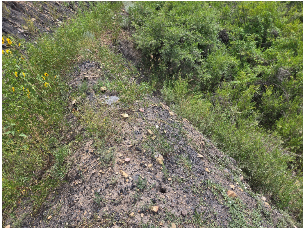
Photo 32: Standing on the berm dividing the clean diverted surface water (D7) from the water contacting disturbed areas (ditch that discharges into D6). The right side has bindweed growth.
