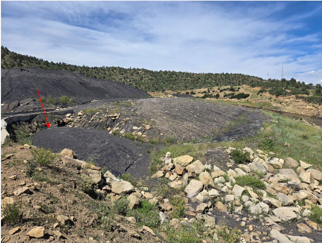
Photo 24: Looking east across where the un-reclaimed RDA benches meet the reclaimed benches. The arrow points to the outlet for C81.
