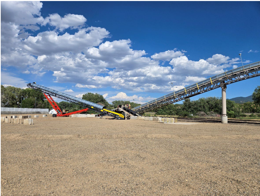
Photo 37: New/replaced conveyor equipment at the Jansen Loadout.
