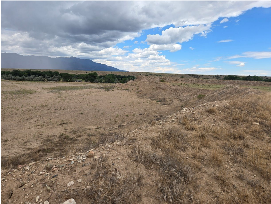
Photo 9: Looking north from the beginning of the highwall along the eastern border of the disturbed area at the 1.5-2H:1V current mining face.
