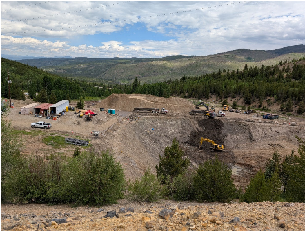
Photo 17: Looking at the progress of the excavation work for the foundation of the future Water Treatment Plant.
