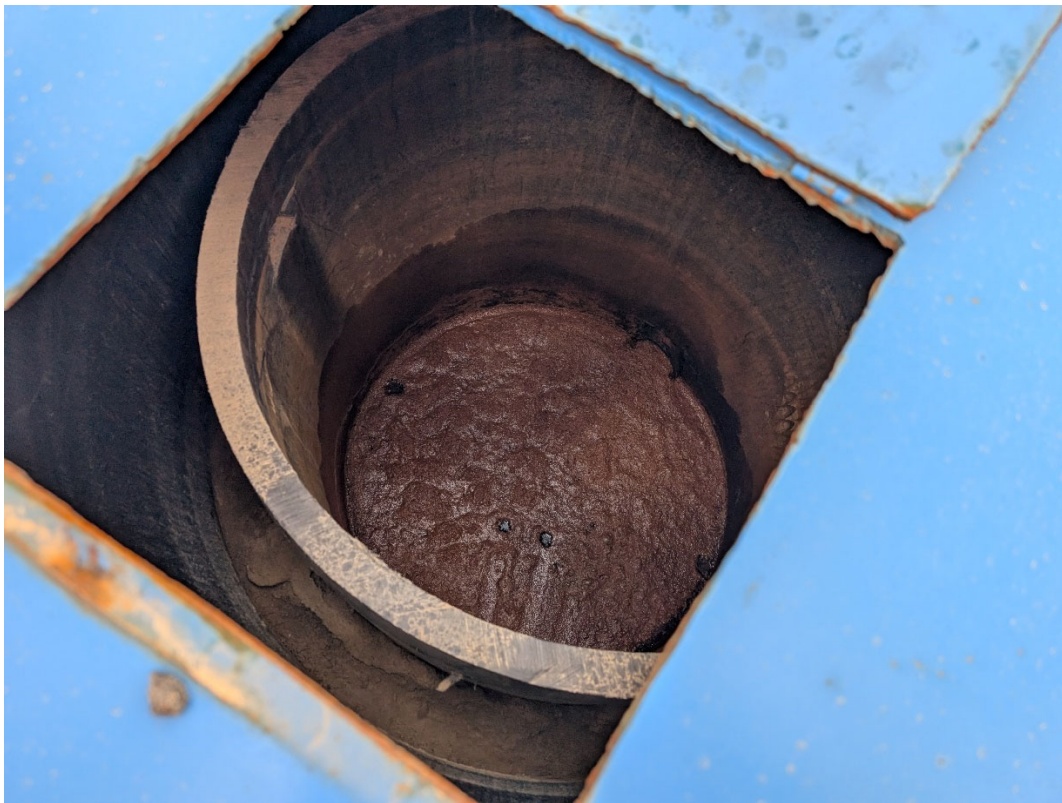
Photo 14: Looking inside the manhole on the Lower Subdrain below 1-Dam.
