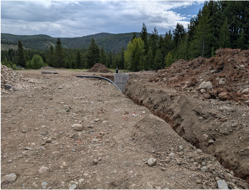
Photo 5: Looking at the excavated trench for the 6-inch pipeline for MLEX-7.
