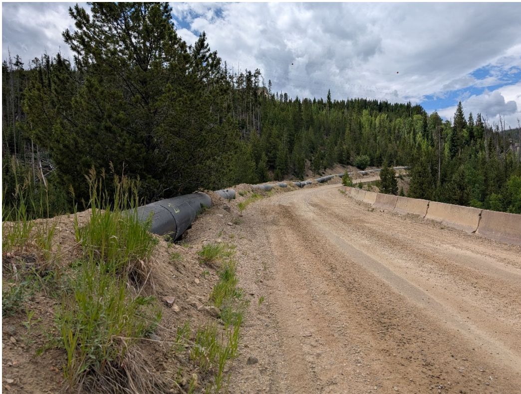
Photo 2: Looking at the TDL along the road, adjacent to the Bear Paw Pipeline.
