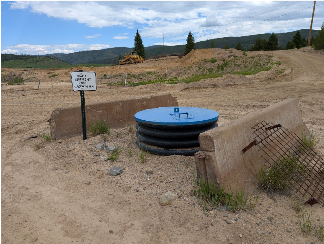
Photo 13: Looking at the Lower Subdrain manhole on the south end of Ute Park below 1-Dam.
