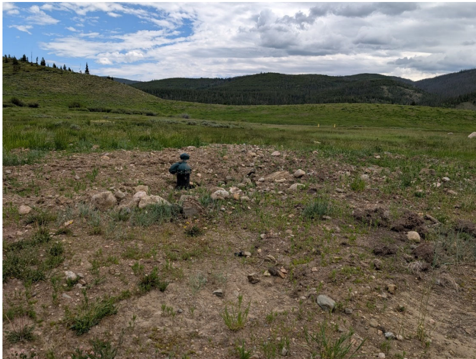
Photo 10: Replacement well drilled at MLEX-1 in Ute Park.
