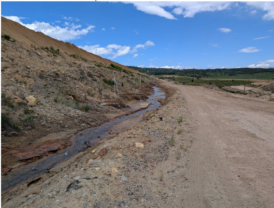
Photo 12: Observing the groundwater drains along the base of 1-Dam.
