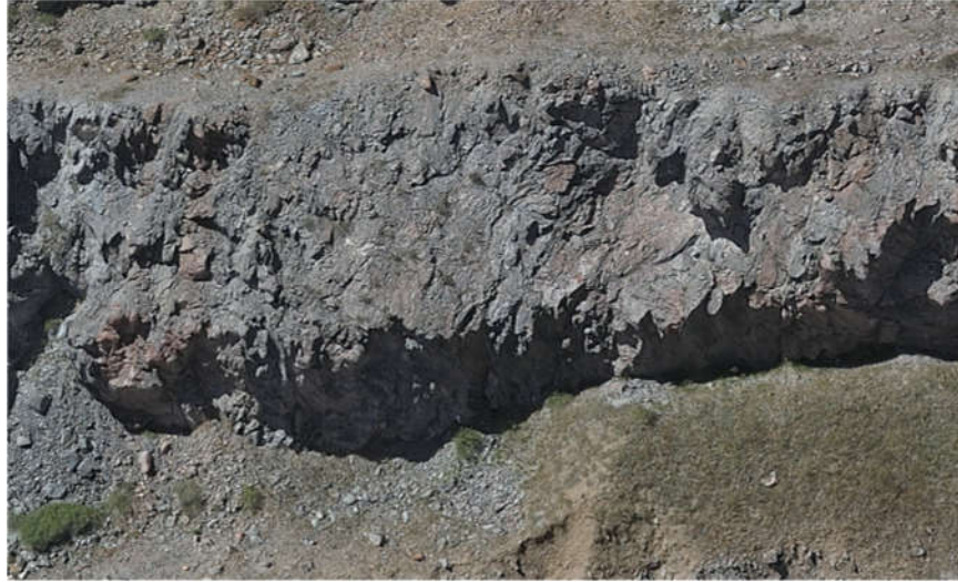
Figure 3: Eastern Facing Bench 6500 Showing Overhang
