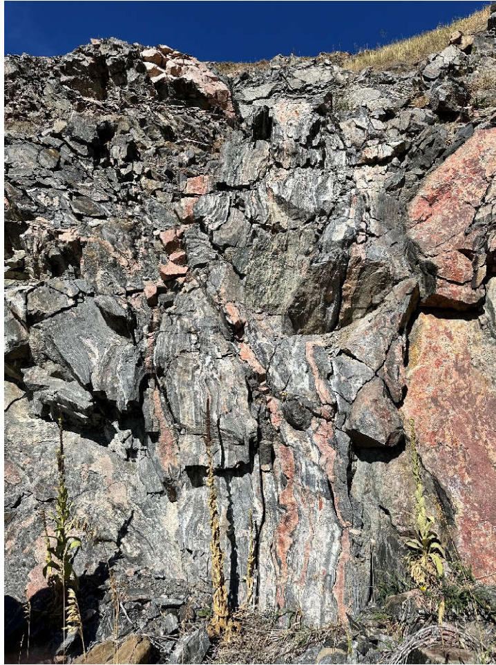
Figure 2: Central East-Facing Bench 6540 Showing Recent Raveling
