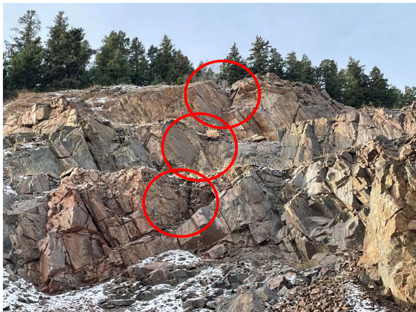
Figure 4: Southwest Corner, Photo taken from Bench 6460, Local Wedge Failure in Red.
