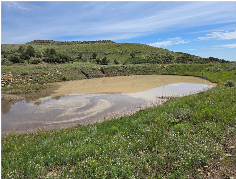
Photo 7: Looking at the erosion on the north side of the Pond 006a banks.
