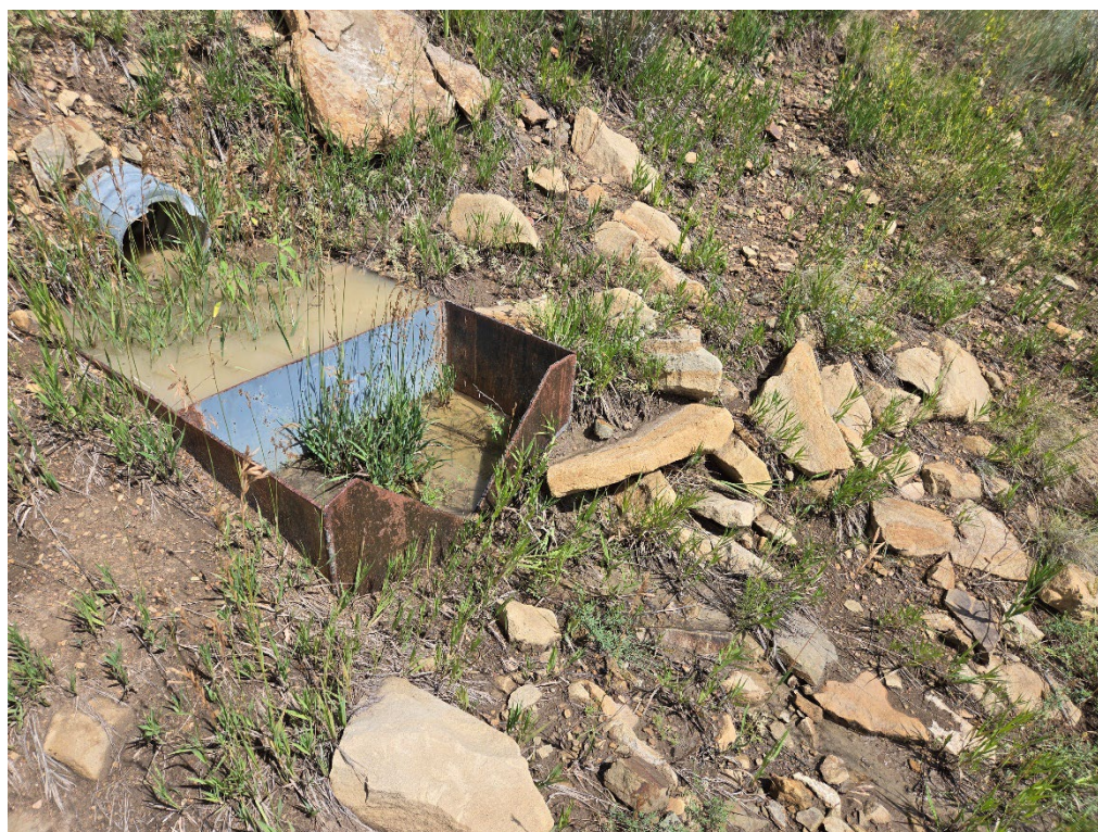
Photo 6: Discharging flume at Pond 006a. The top part of the flume has filled with sediment and vegetation, causing some of the discharge to escape from the sides of the top.
