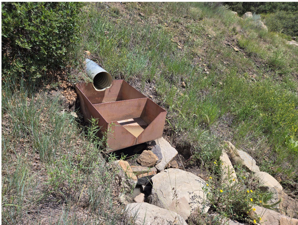
Photo 11: Flume for Pond 007a
