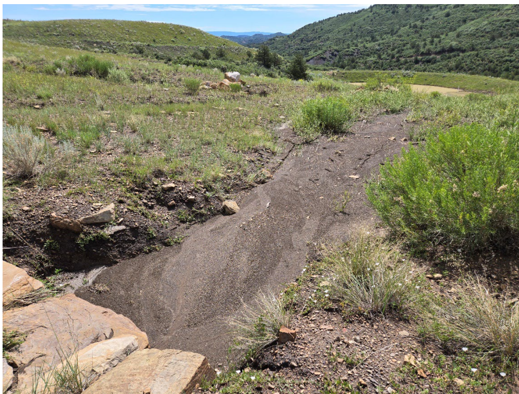
Photo 8: Check dam full of sediment leading down to Pond 006a
