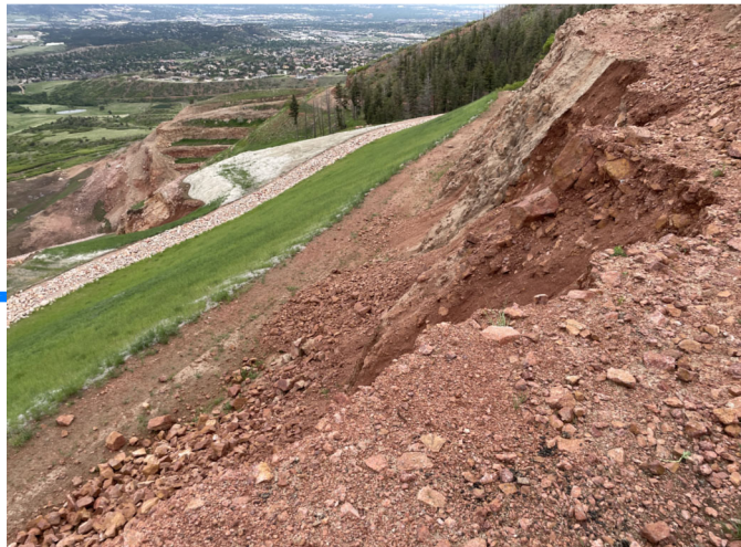
3. ROCK RAVELLING ON EXCAVATED BENCH. PHOTO TAKEN AT 3A. 3B SHOWED SIMILAR RAVELLING.
