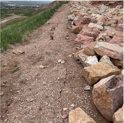
2. SETTLEMENT CRACKS ON EDGE OF BENCH.
