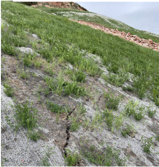
1. SETTLEMENT CRACK AT EDGE OF FILL.
