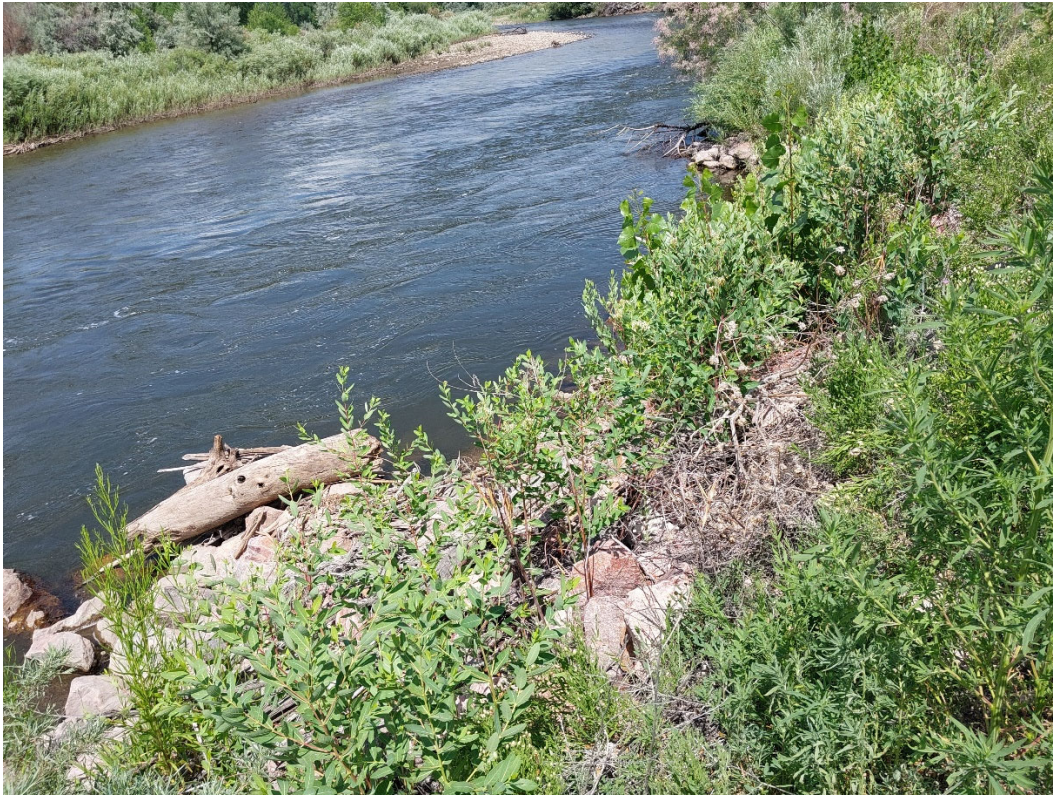
Photo #11: The armored north bank of the Arkansas River with voluntary vegetation established.
