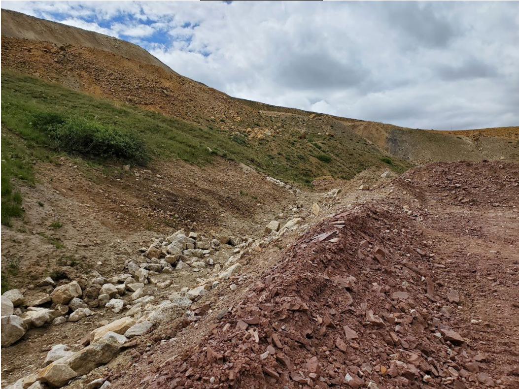
Photo 1: View to the south of the start of the East Interceptor above McNulty.
