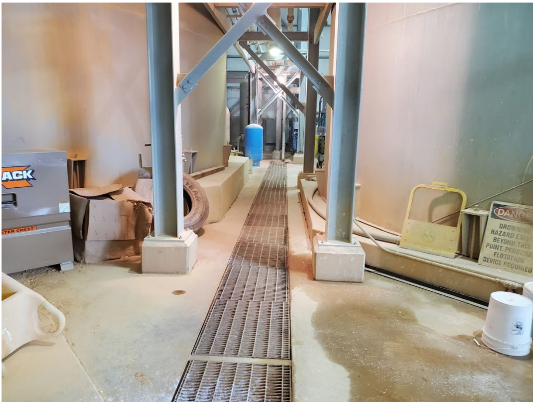
Photo 10: View to the south of containment in SDP.
