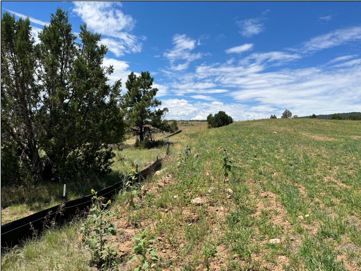
Photo 5: View south of the silt fence installed at the eastern end of the pit floor, towards the site's natural drainage.
