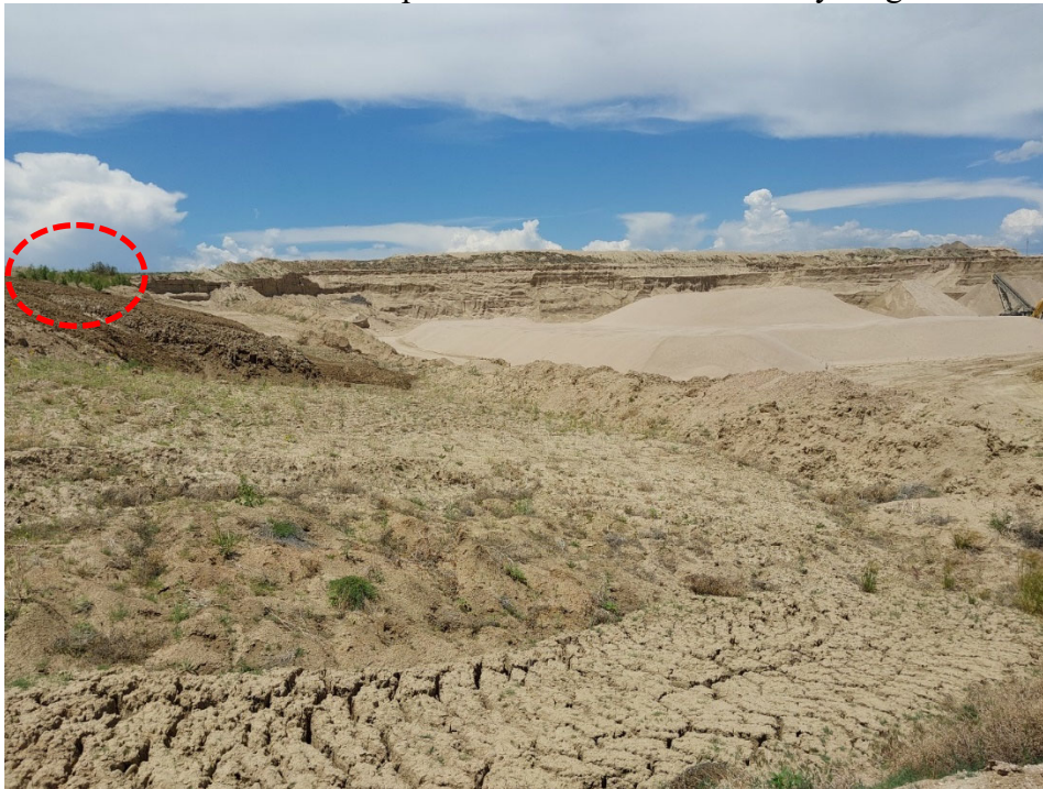
Photo #7: The slope on the left side of the photo is the area that has been backfilled and graded. Salt cedar can be seen on the top of the slope, circled in red. The western highwall can be seen in the background and a large product stockpile is seen on the pit floor.
