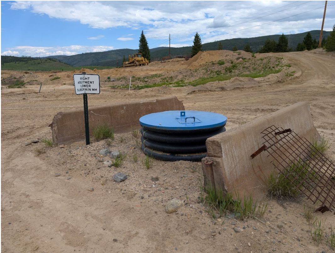
Photo 13: Looking at the lower subdrain manhole on the south end of Ute Park.
