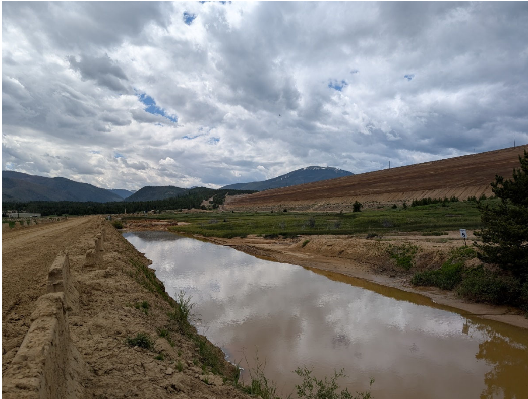
Photo 15: Looking at the north end of the seep water canal below 1-Dam.
