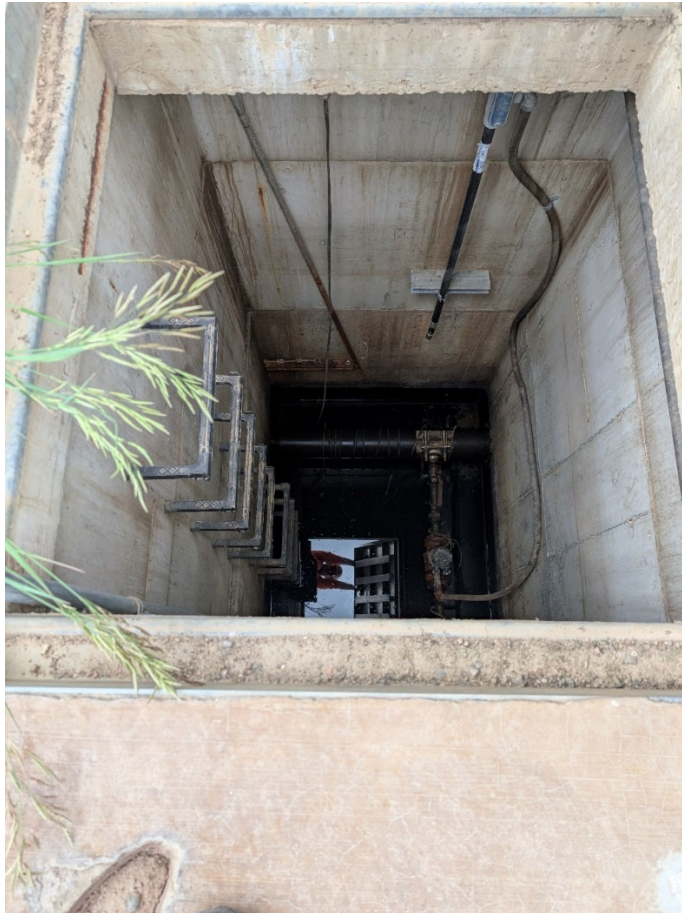
Photo 9: Looking down into the vault at MLEX-1.
