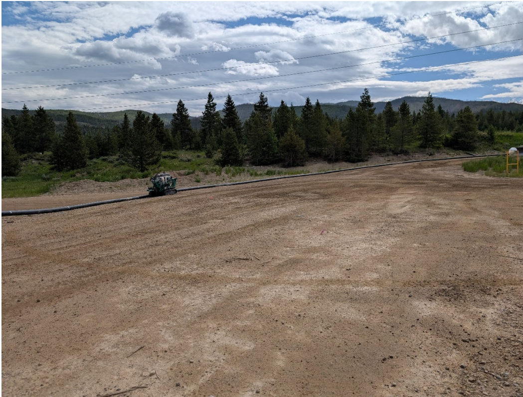
Photo 7: Pipeline laying on the ground that will be installed to discharge water from MLEX-7 into seep collection channel adjacent to the Ute Park Pump Station.
