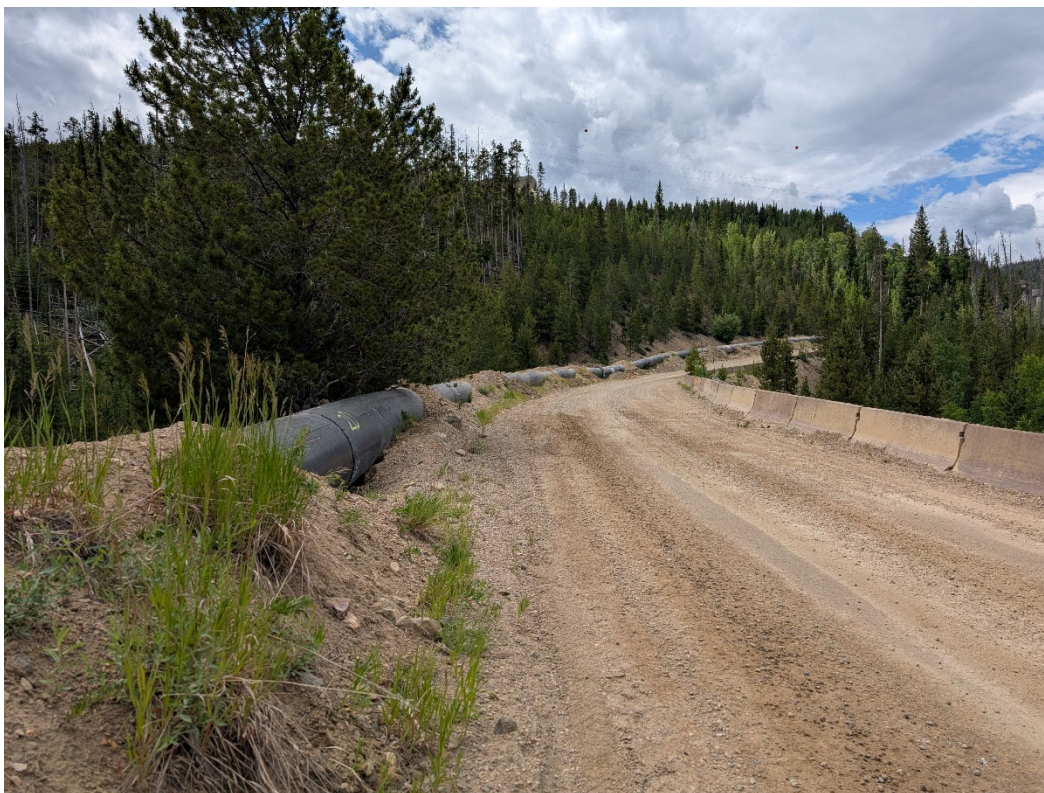
Photo 2: Looking at the TDL along the road, adjacent to the Bear Paw Pipeline.
