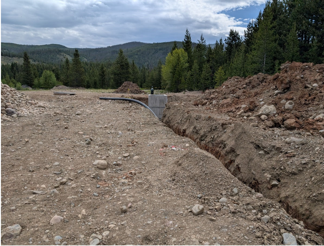
Photo 5: Looking at the excavated trench for the 6-inch pipeline for MLEX-7.
