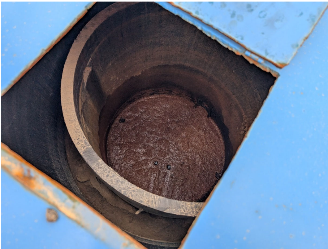
Photo 14: Looking inside the manhole on the lower subdrain.
