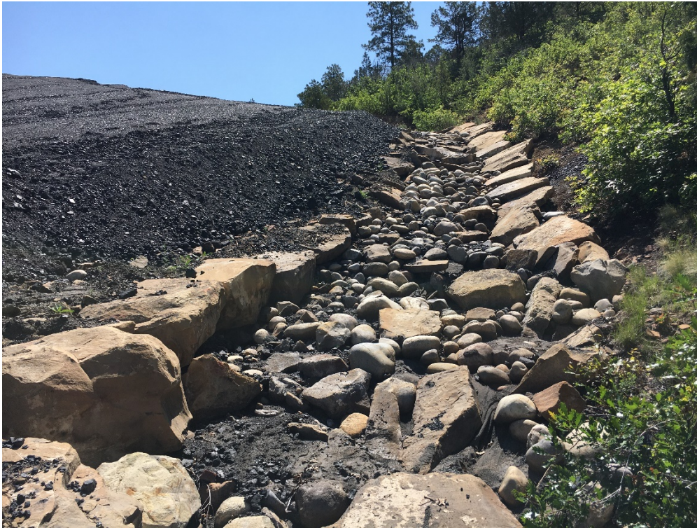
Pic. 7 – Reach 10, armored section between lower and upper waste piles.
