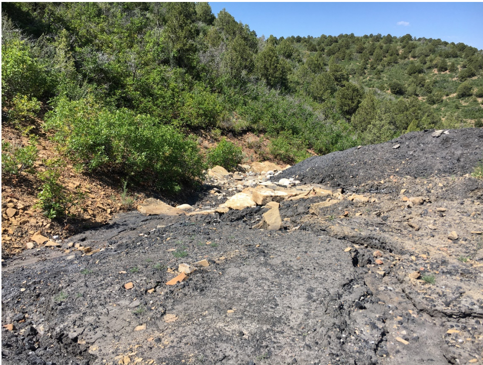
Pic. 8 – Minor erosion evident at the discharge from the upper waste pile to Reach 10. Monitor and maintain so larger, erosional channels do not start forming.
