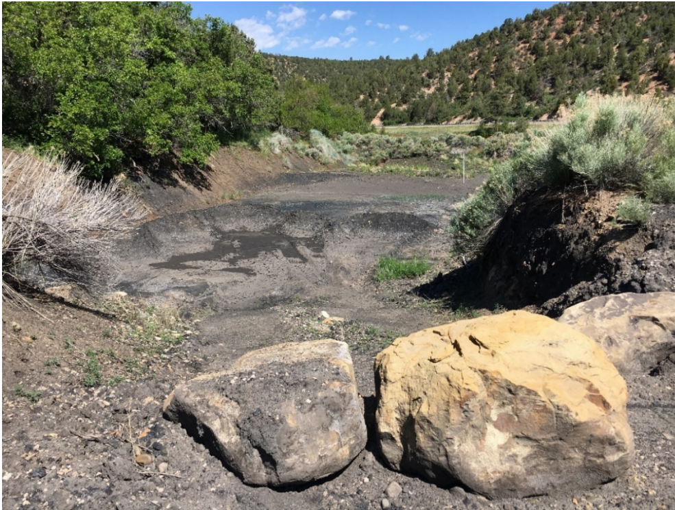
Pic. 3 – View into west pond. Evidence of sediment removal initiated but not complete due to muddy conditions just below the surface.
