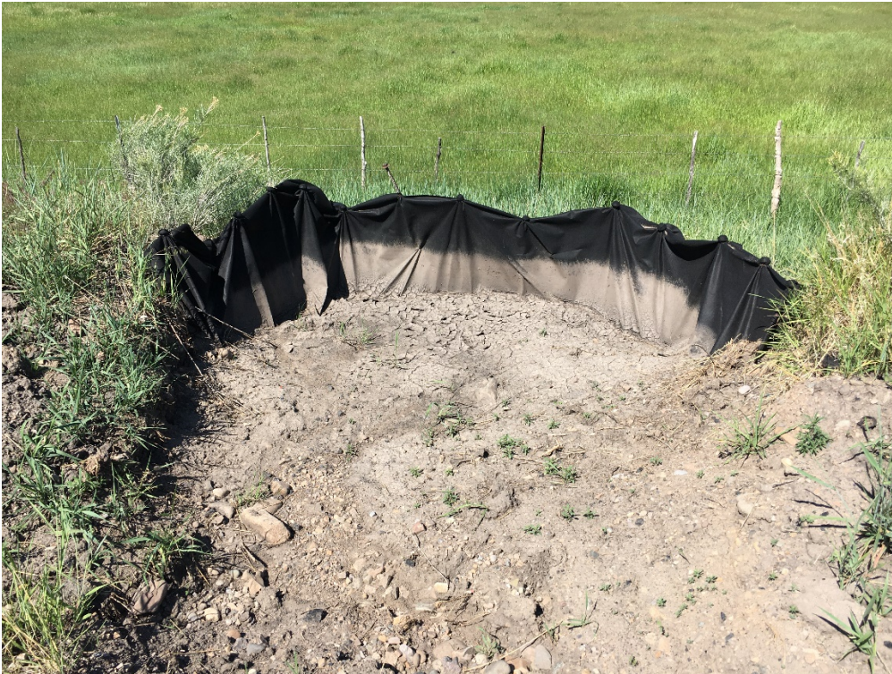
Pic. 1 – Sedimentation trap anchored and catching sediment.
