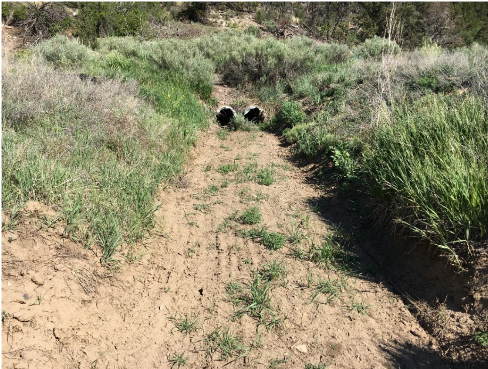
Pic. 4 – Culvert outfalls where the West Clear Water Ditch drains towards the Main Drainage Ditch.
