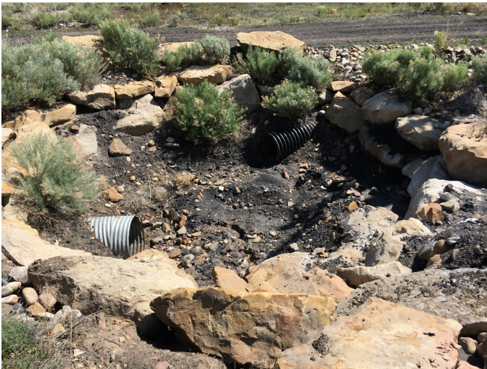
Pic. 4 – View of culverts which receive flows from Reach 9 and from below the lower waste pile.
