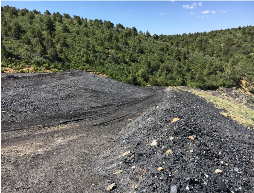
Pic. 11 – Bank stabilization and grading, and berming placed along edges of the upper waste pile.
