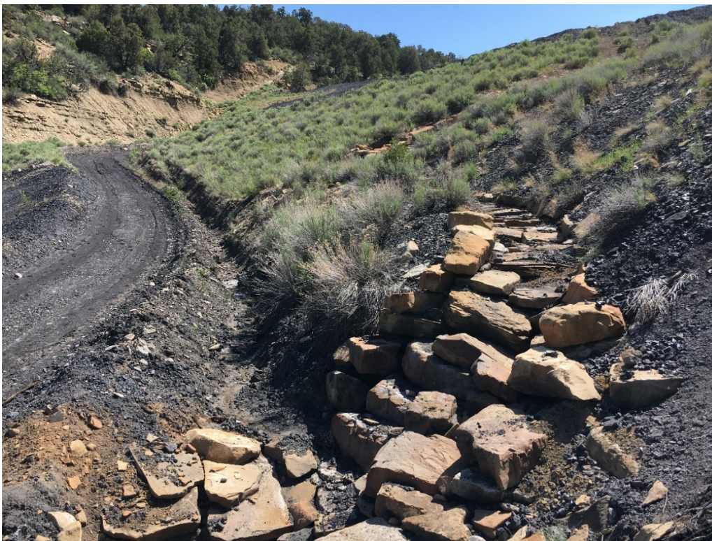
Pic. 6 – Haul road ditch and lower portion of Reach 10 prior to draining towards the lower waste pile area.
