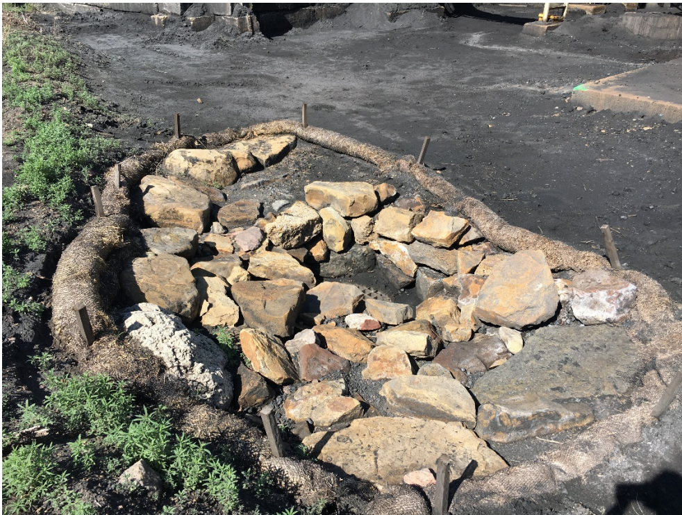
Pic. 6 – Straw wattles and rock armor near the vibratory processing area.
