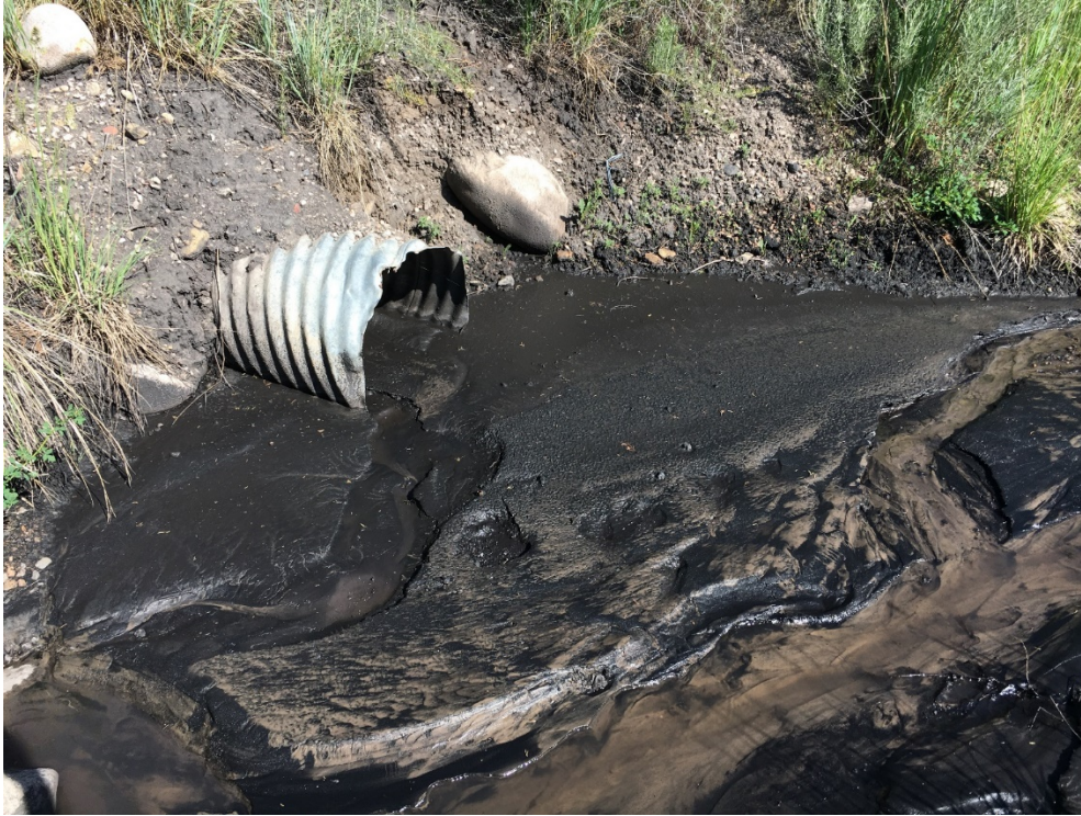
Pic. 9 – Some sediment accumulation at the culvert outlet that ultimately drains to the detention pond (south of scale house).
