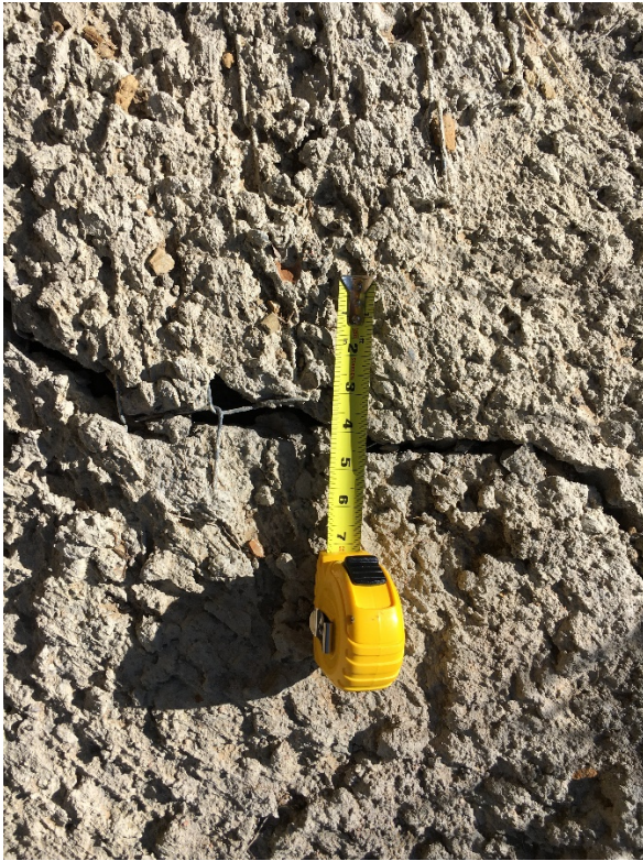
Pic. 9 – Crack along the armored section of Reach 1.
