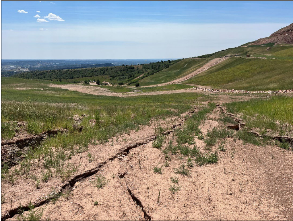
Photo 13: Erosional issues on old haul road, source of erosion shown in Photo 12.
