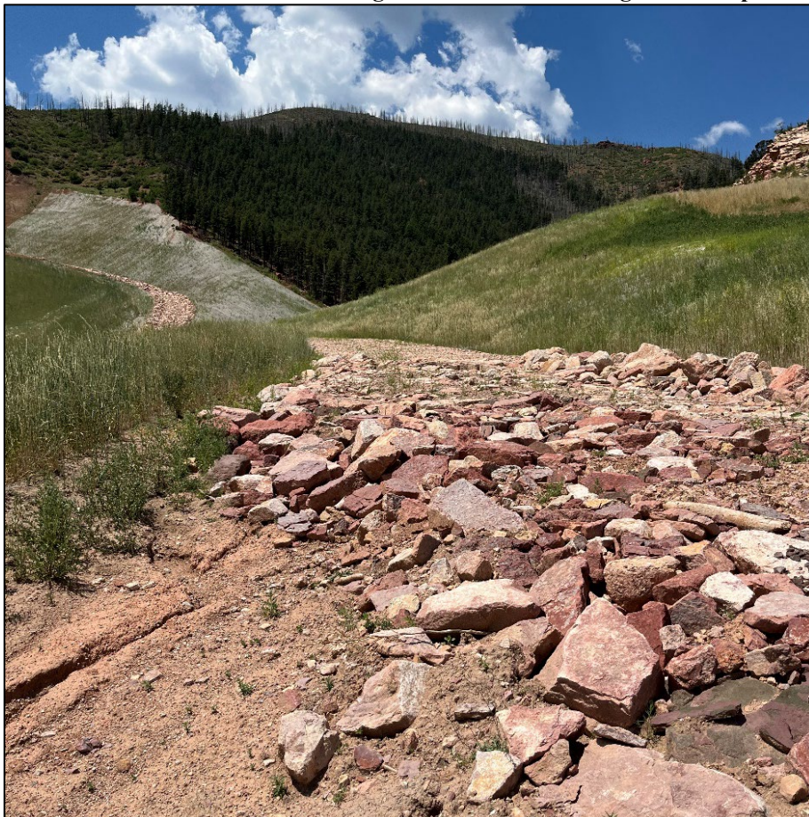
Photo 12: View east of the north channel, this area was observed to be the source of a few downslope erosional issues shown in
