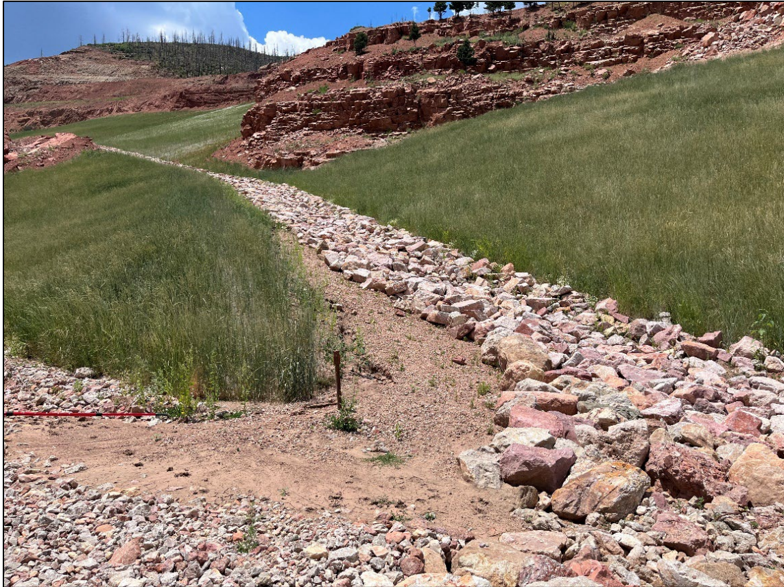
Photo 15: Sedimentation observed at the tie in on Channels T7 and T8.
