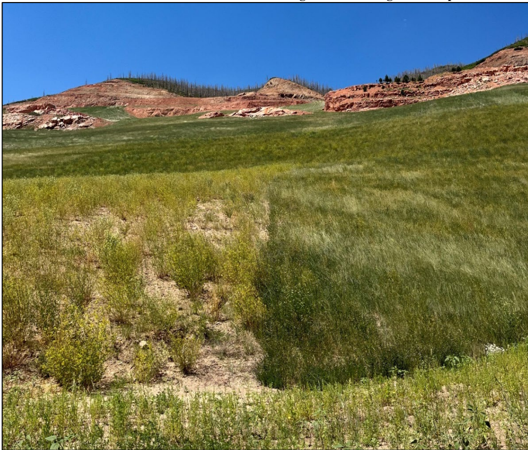
Photo 10: View west, depicts difference between hillslopes revegetated with matting versus drill seeding alone.
