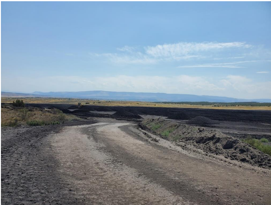
Photo 10: View to the east of Refuse Pile RP-A and the windrows being spread.
