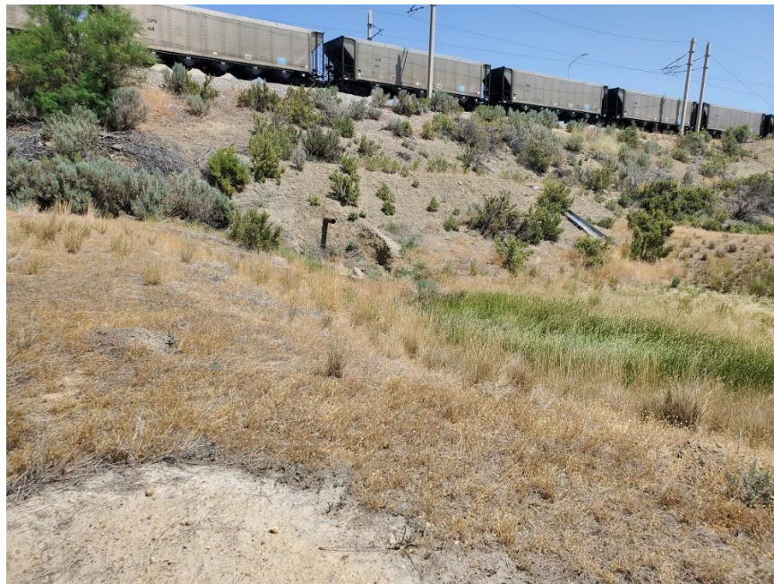
Photo 6: View to the north of erosion scar on RR-1 pond.
