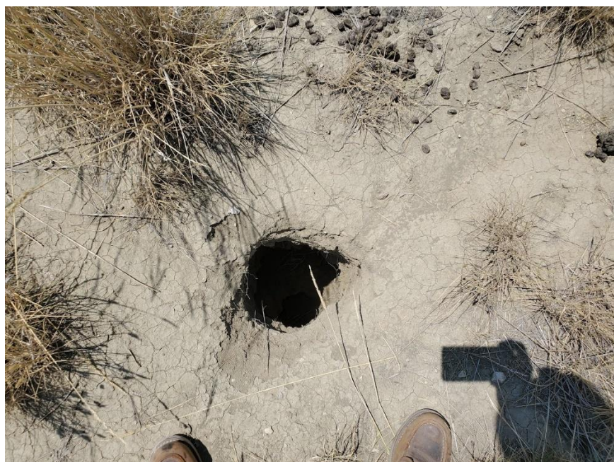
Photo 8: View to the north of animal burrow that was filled on RP-4 Pond embankment.
