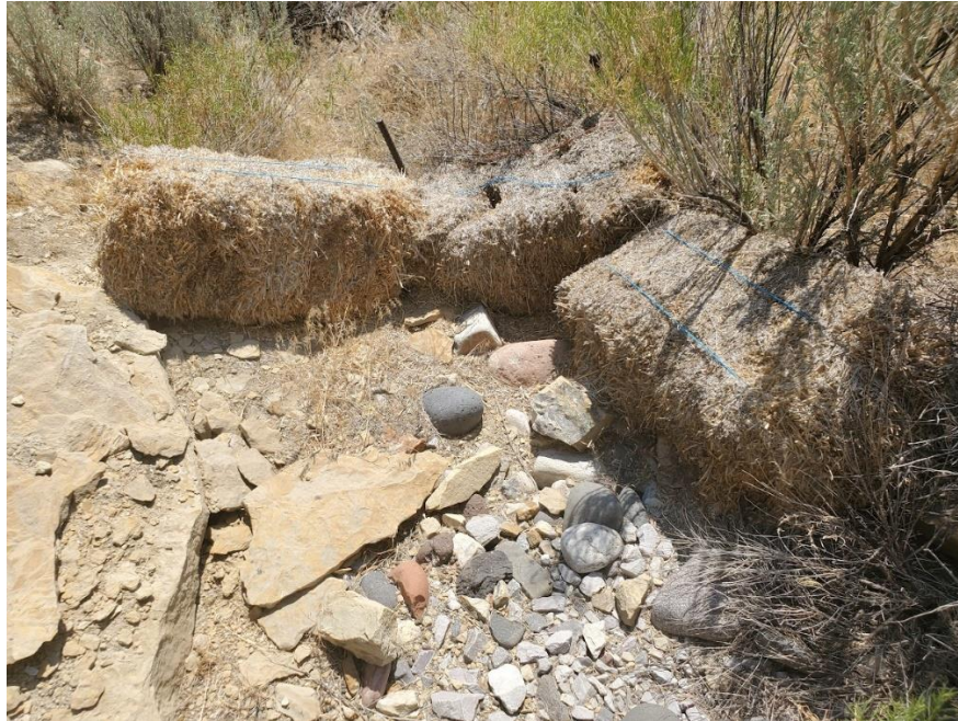
Photo 1: View to the east of straw bales at explosive pad drainage.
