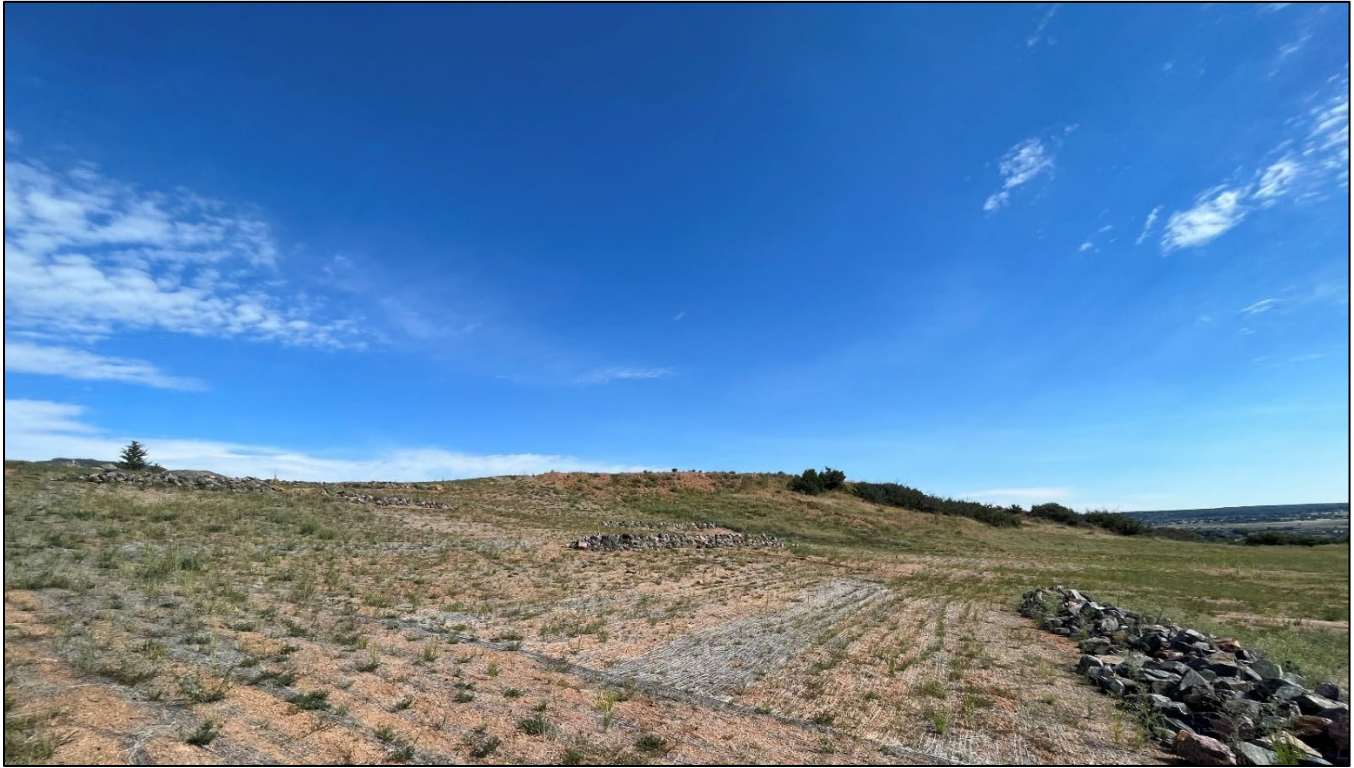
Photo 2: View north of the reclaimed slope between the upper and lower mine areas, rock check dams are in place.
