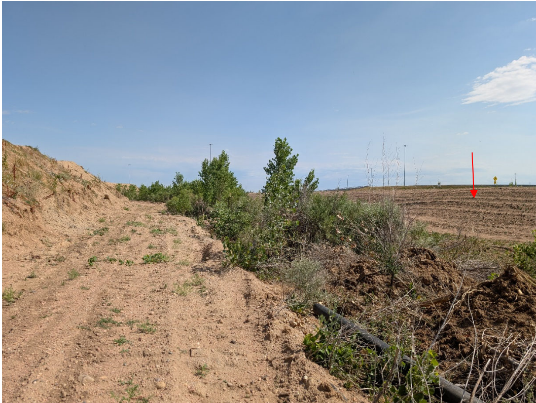
Photo 6: Looking north at a low spot on the eastern side of the large stockpile in Mining Area III. Topsoil berm was observed in a berm on the right (red arrow).
