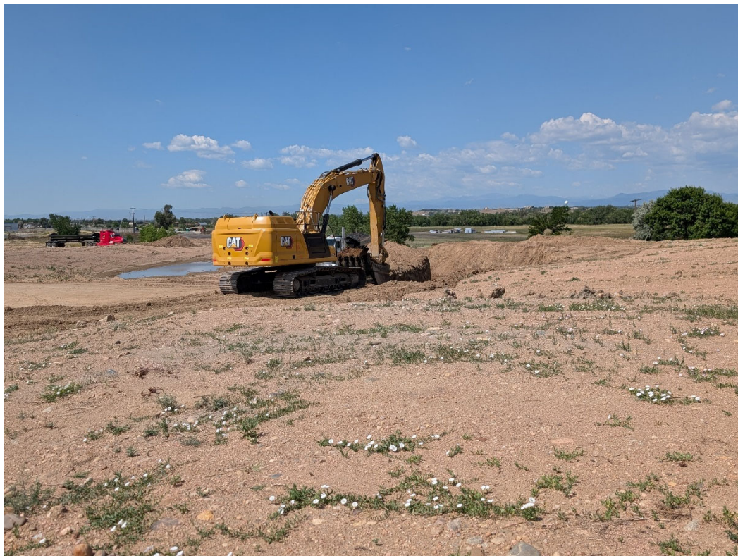
Photo 2: Excavator working at the south end of the large stockpile in Mining Area III.
