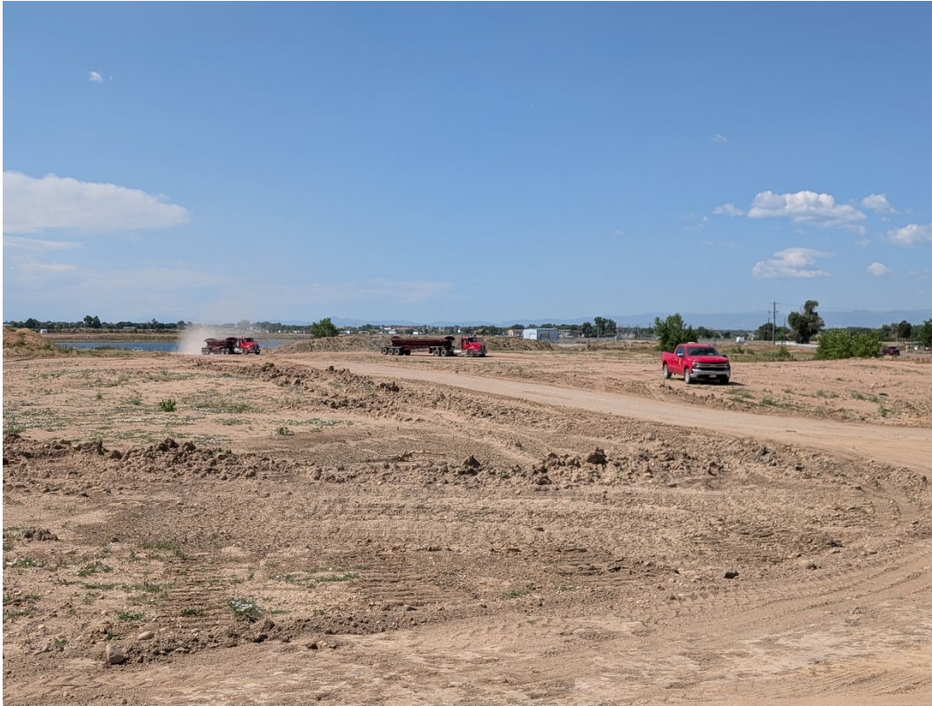
Photo 1: Looking south across Mining Area III. Haul trucks entering site.
