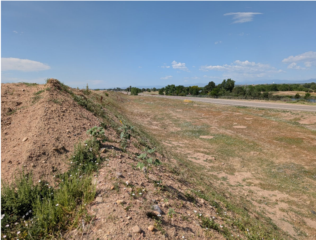
Photo 9: Looking south down the west side of the stockpile. Brighton Rd is on the right (red arrow).
