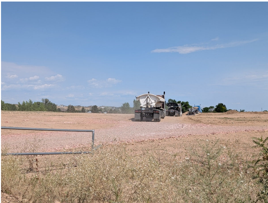
Photo 14: Standing at the entrance to the site. Multiple haul trucks entering the site during the inspection.
