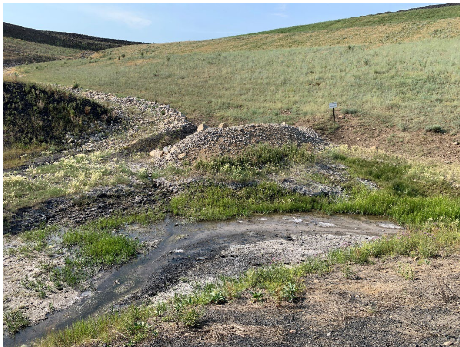
Photo 2- Waste Pile underdrain discharging to Pond D
