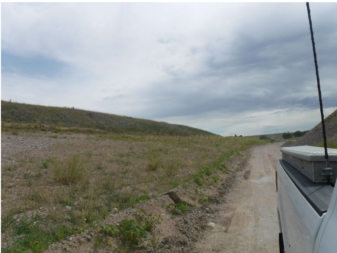
Photo 2: Regraded northern pit area slope (4H:1V) and vegetate topsoil stockpile
