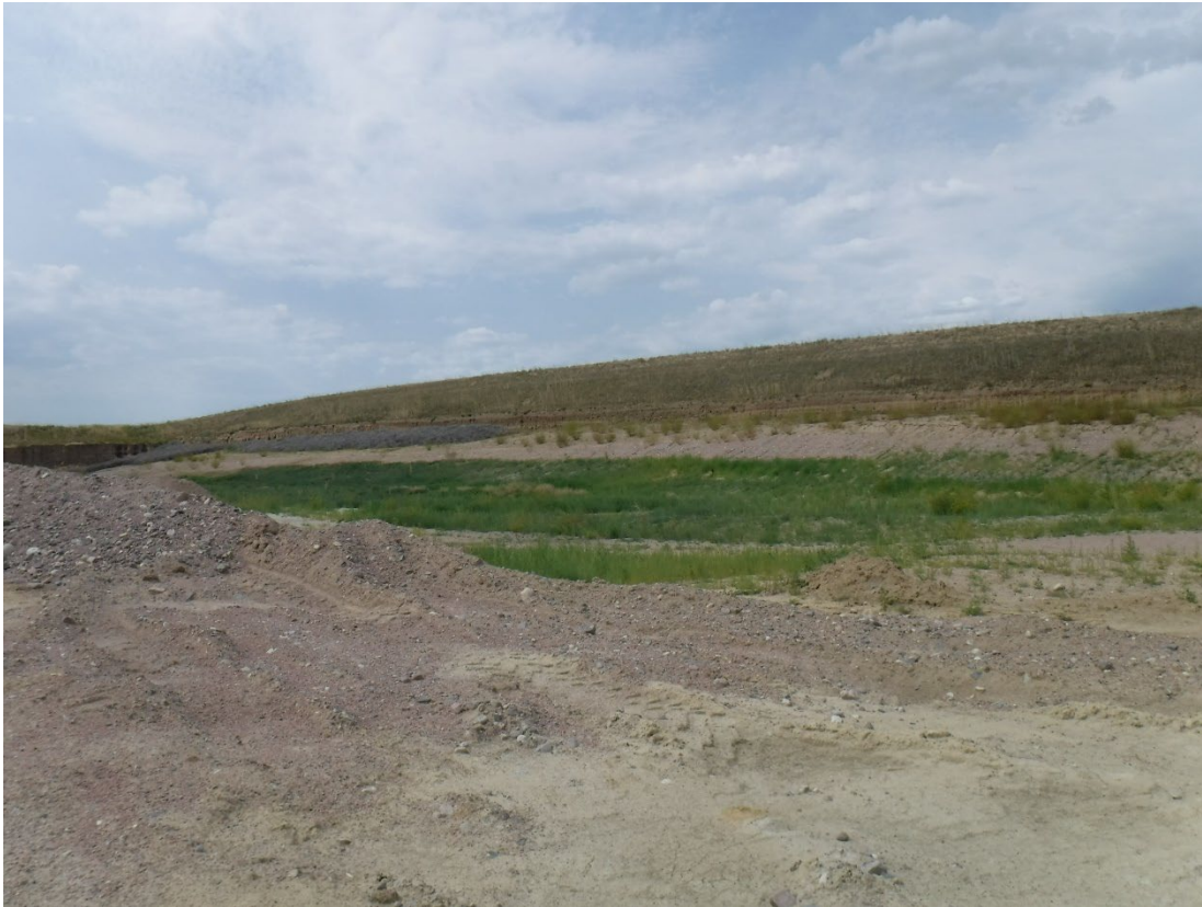
Photo 3: Regraded northwestern pit area slope (4H:1V) and vegetate topsoil stockpile
