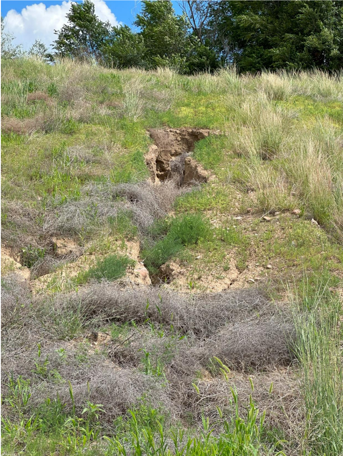
Photo 22. Erosion gully in buttress
