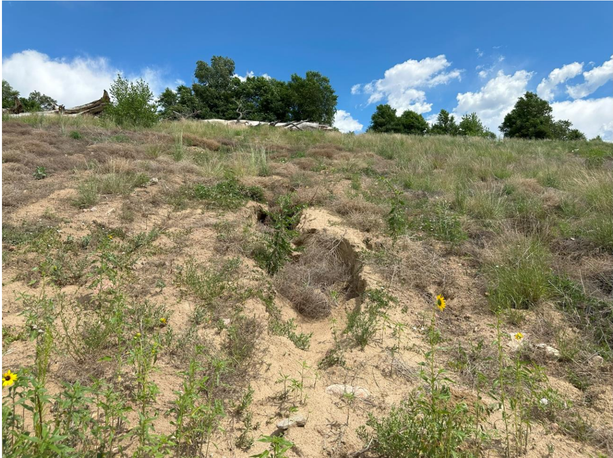
Photo 21. Erosion gullies in buttress
