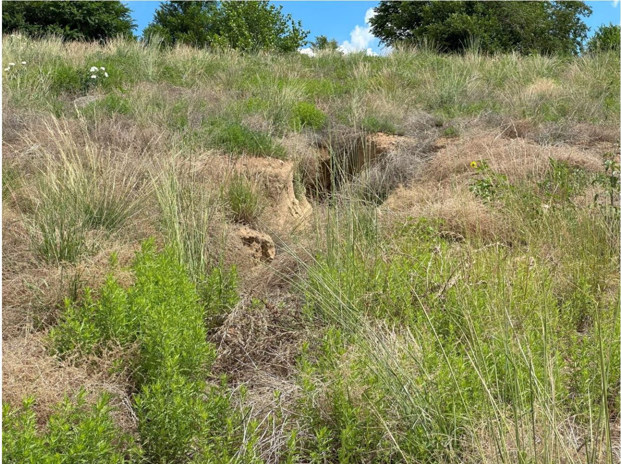
Photo 13. Erosion gully in buttress
