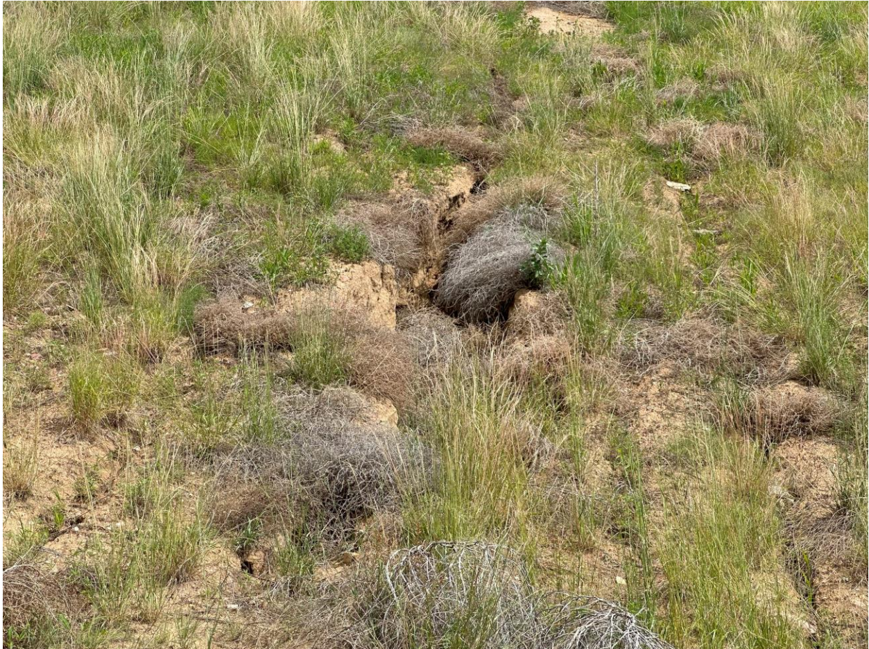
Photo 17. Erosion gully in buttress
