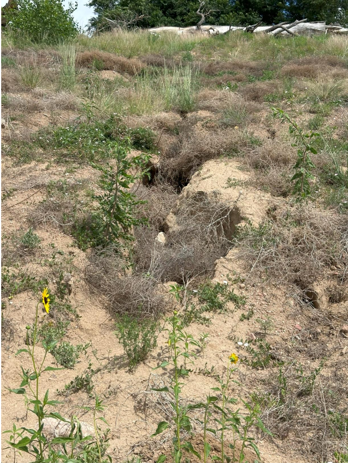
Photo 12. Erosion gullies in buttress
