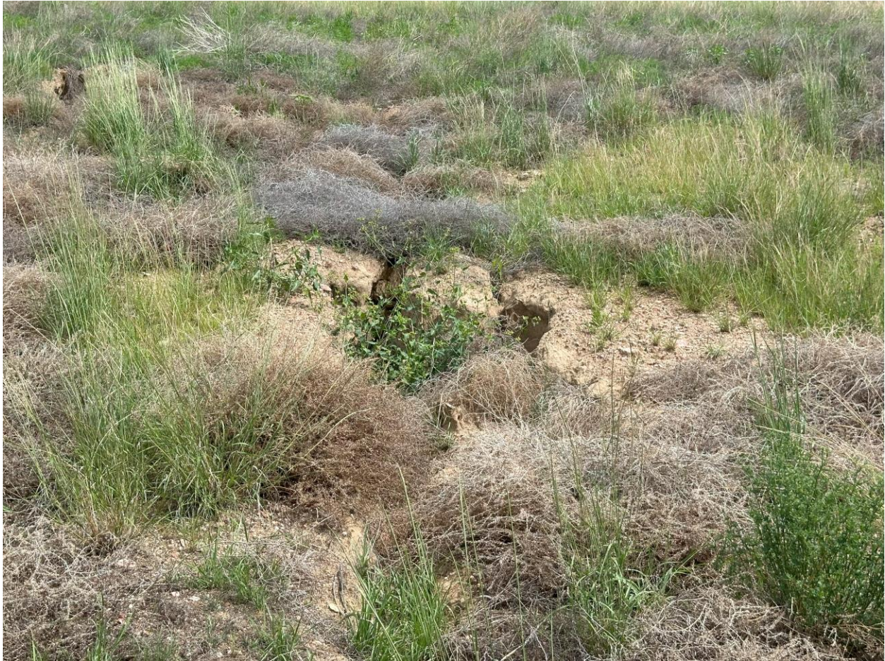
Photo 16. Erosion gully in buttress
