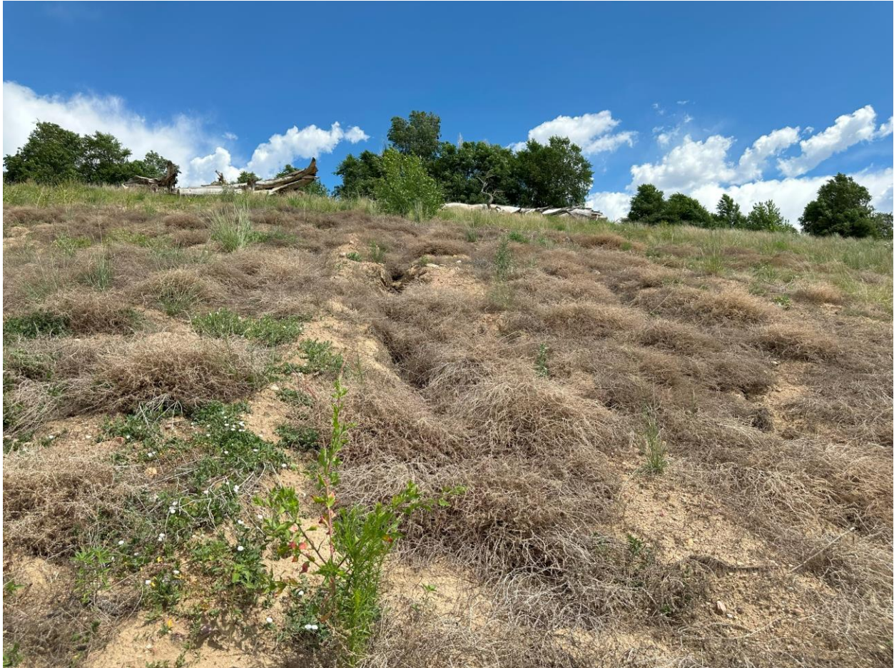
Photo 11. Erosion gullies in buttress
