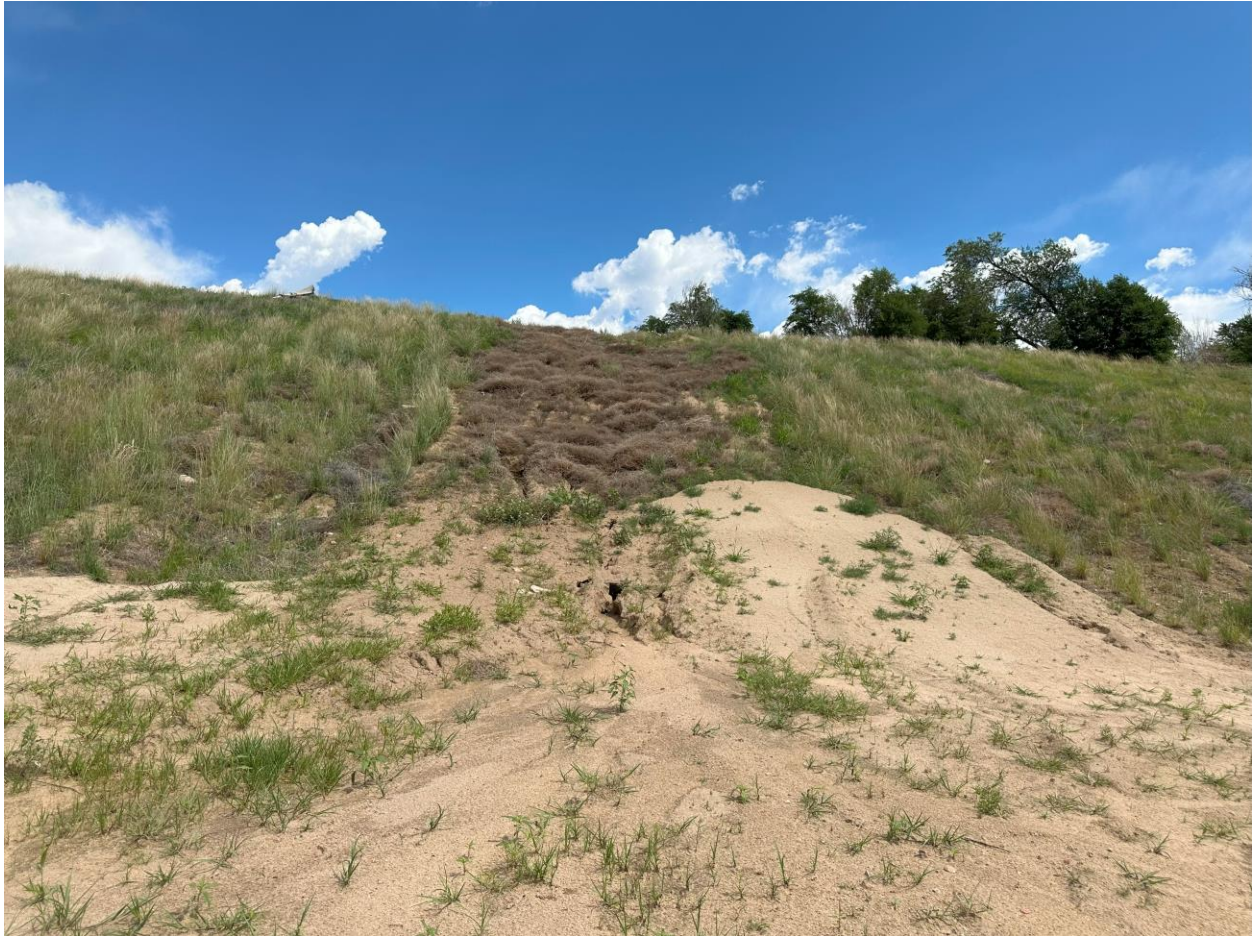
Photo 14. Erosion gullies in buttress
