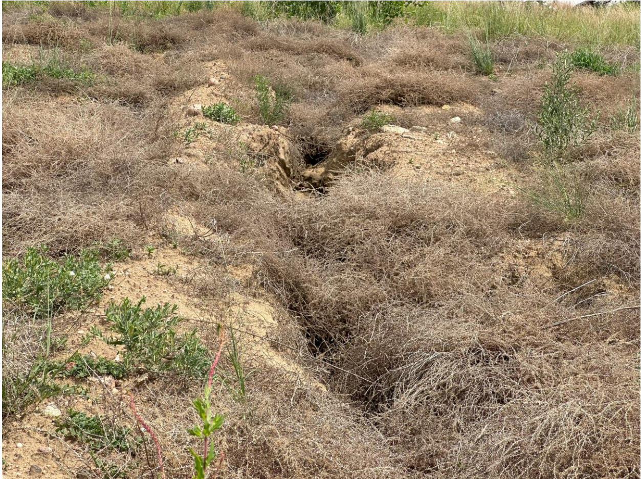
Photo 20. Erosion gully in buttress
