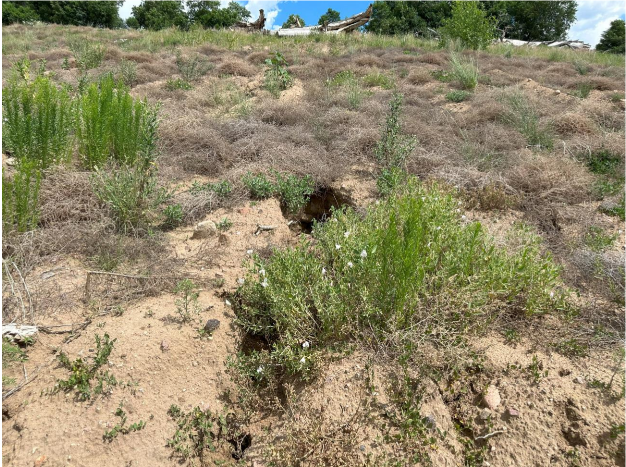
Photo 19. Erosion gully in buttress
