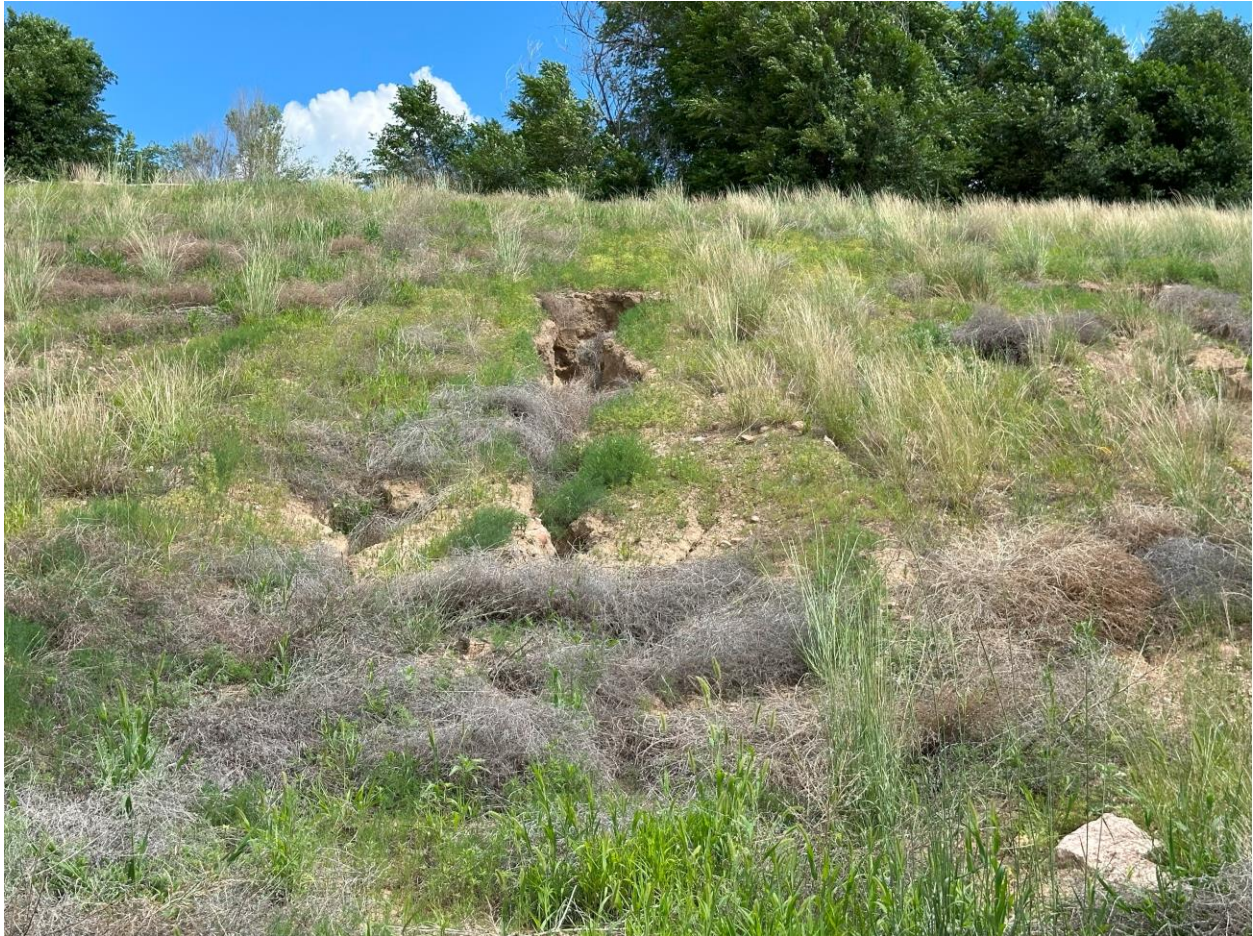
Photo 10. Erosion gullies in buttress
