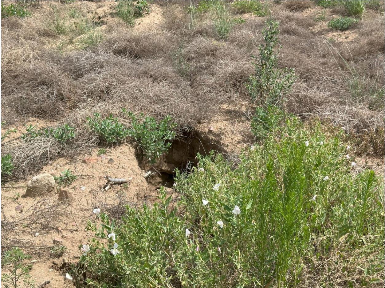
Photo 9. Erosion gully in buttress
