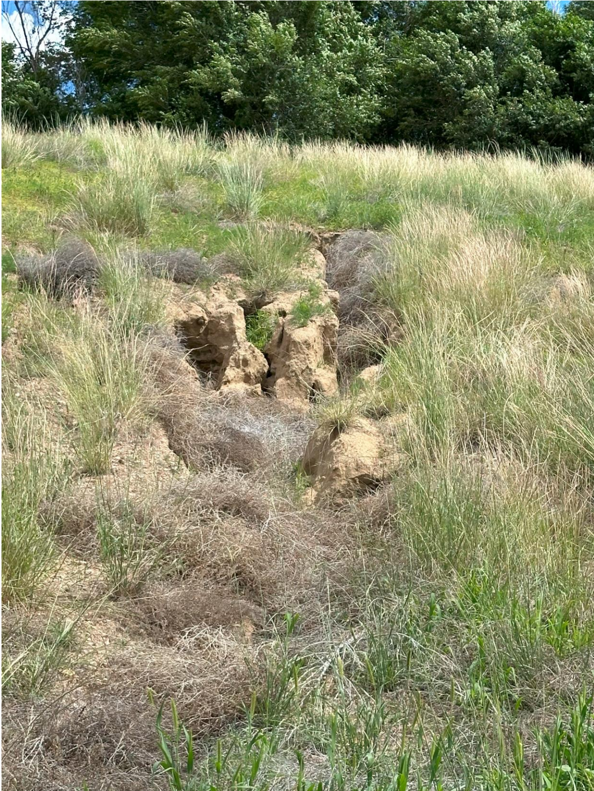
Photo 4. Erosion gullies in buttress
