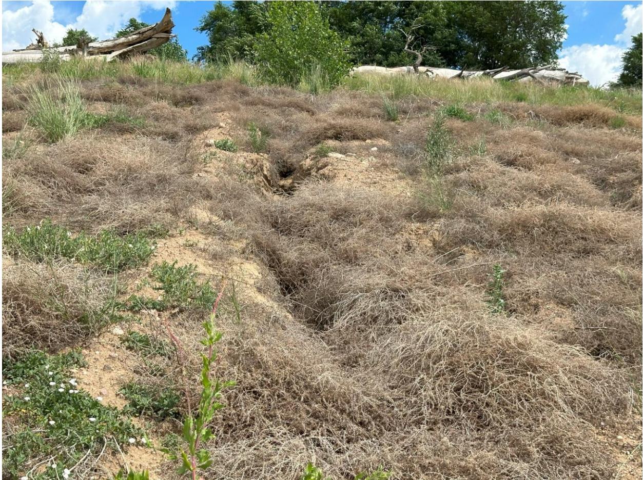
Photo 8. Erosion gullies in buttress
