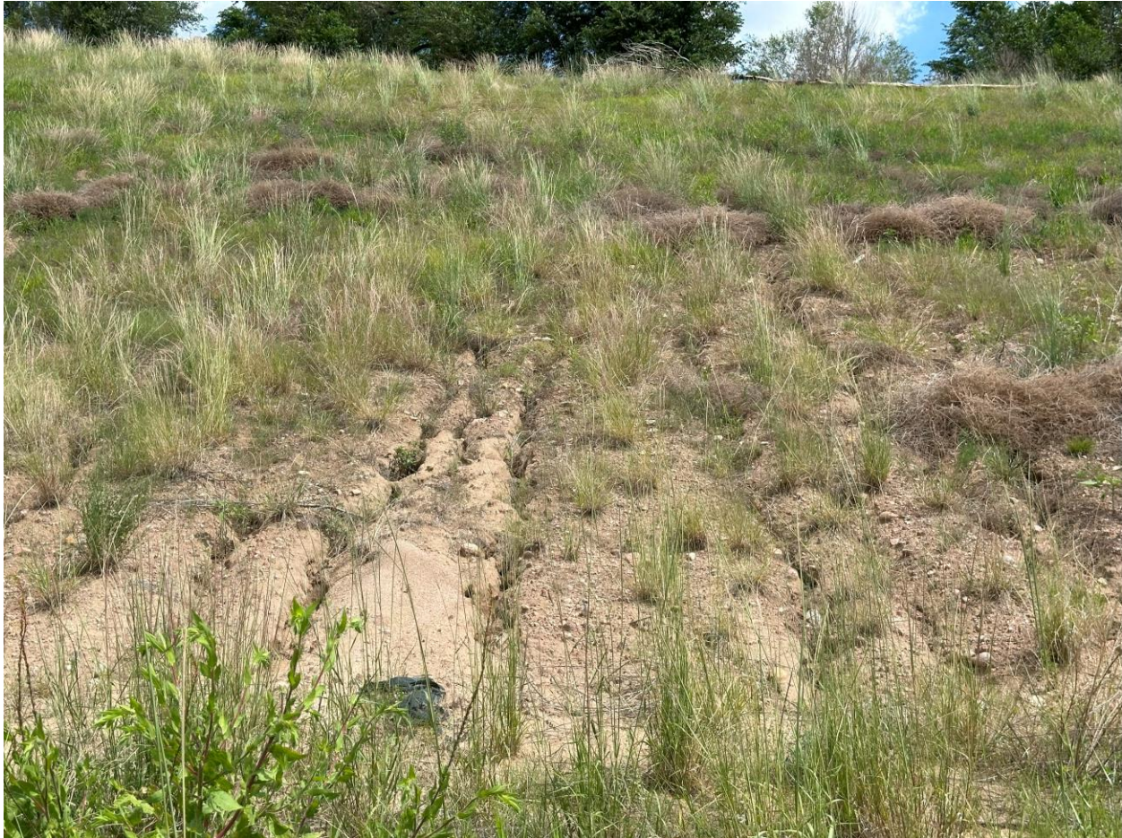
Photo 15. Erosion gullies in buttress
