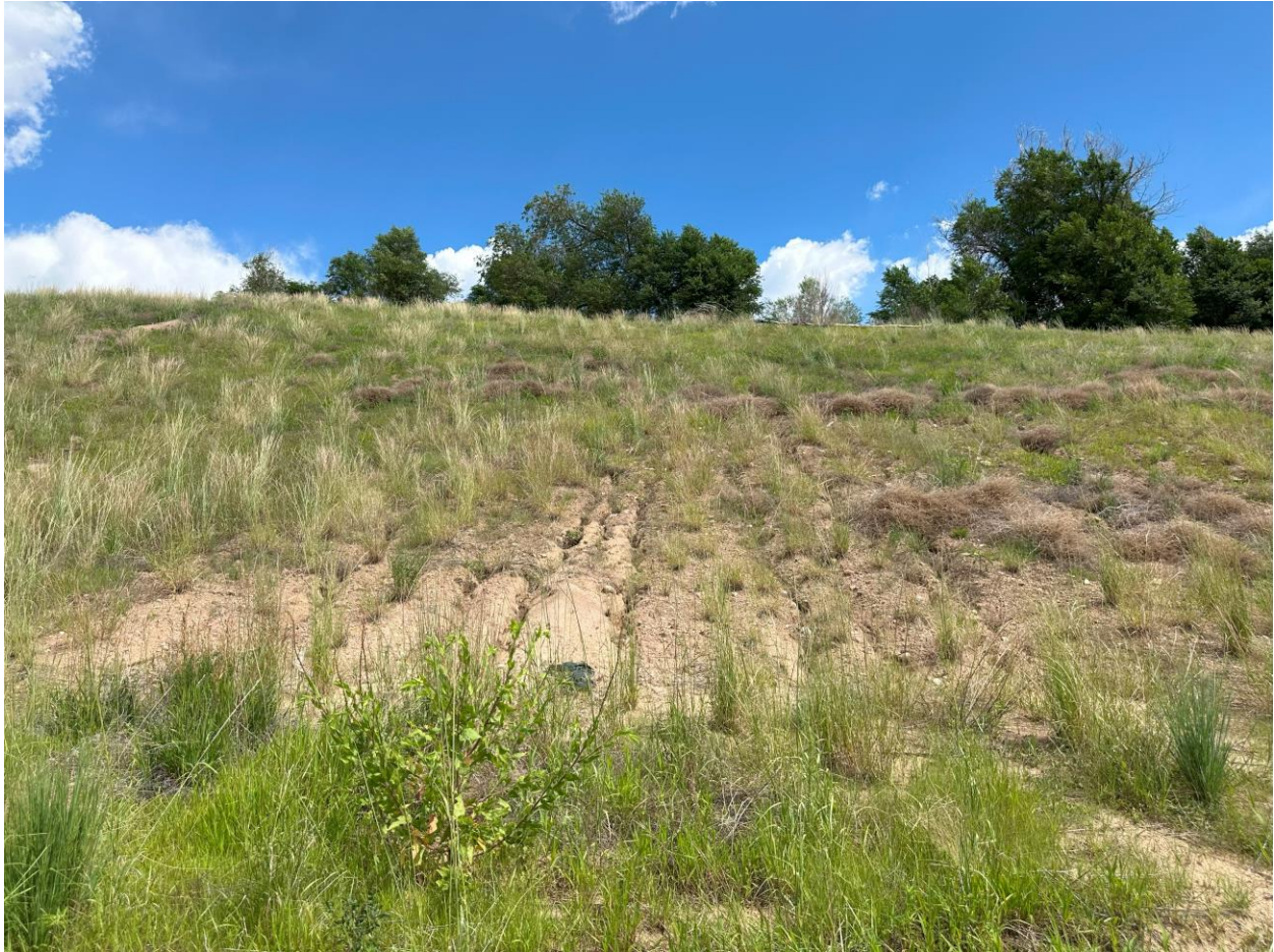
Photo 18. Erosion gullies in buttress
