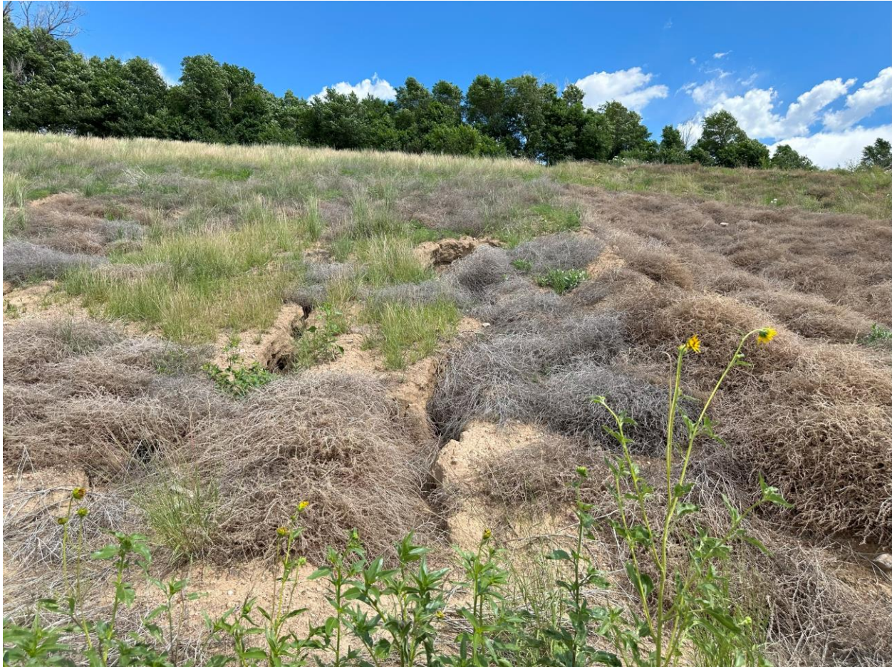
Photo 7. Erosion gullies in buttress
