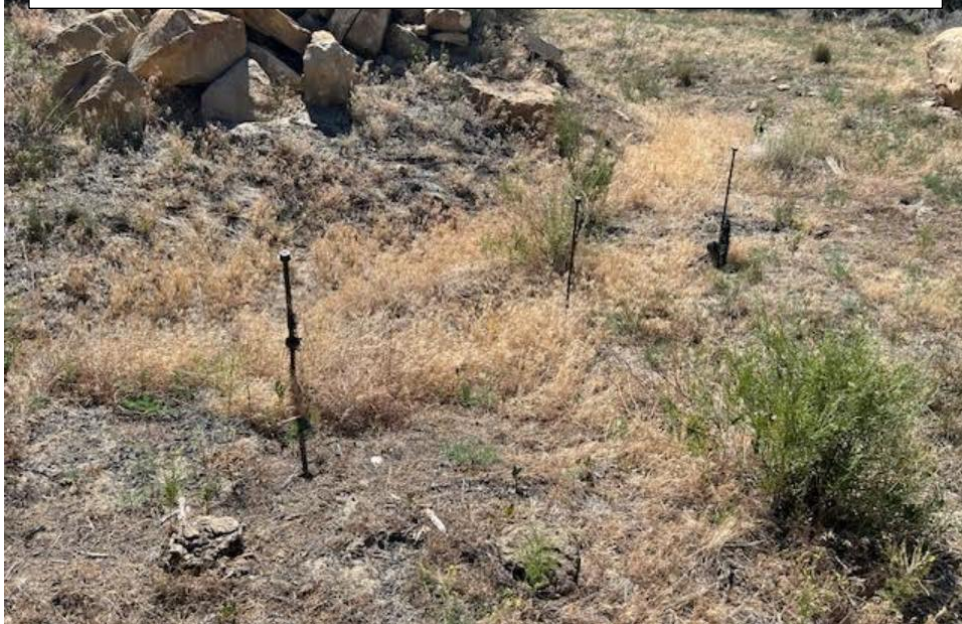
Photo 16: The torn and missing silt fence at the subsoil stockpile sump.
