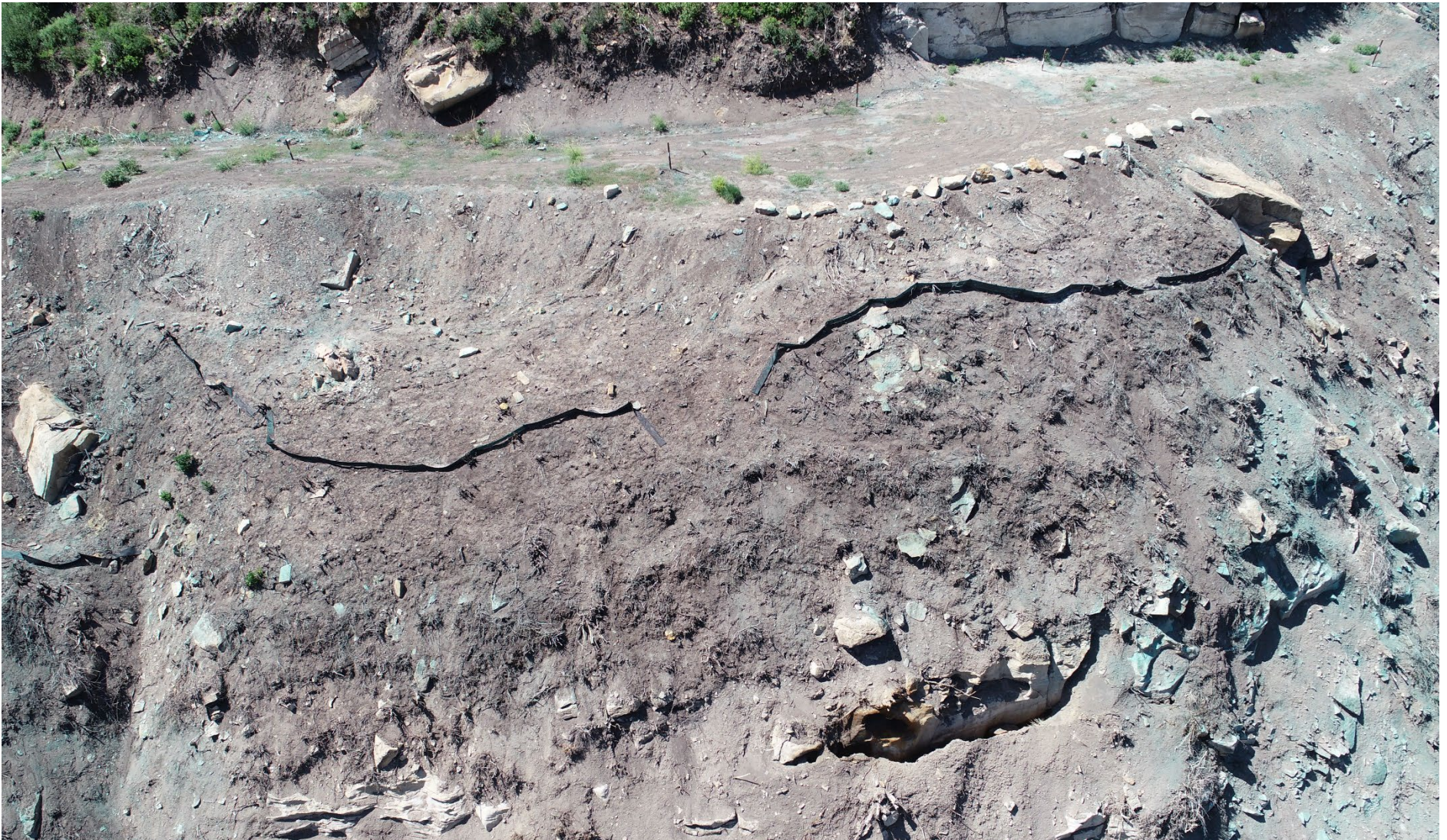
Figure 11: Bench and silt fence
