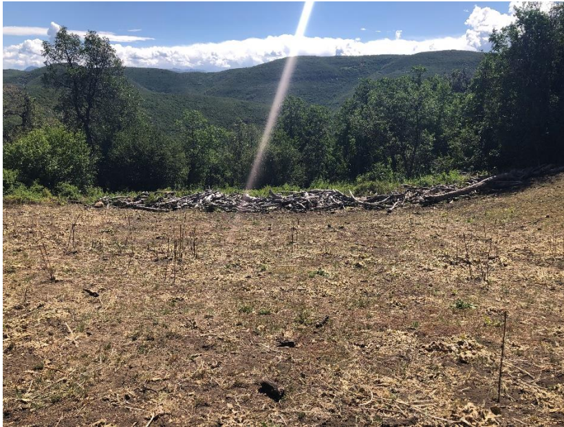
Pad for GVB-B17C – well graded, branches for erosion control, poor vegetation
