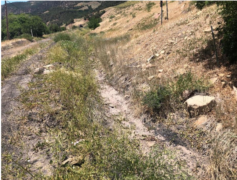
Ditch F-7, along toe of Gob Pile #2 – erodible channel does not meet the current spec, but is stable
