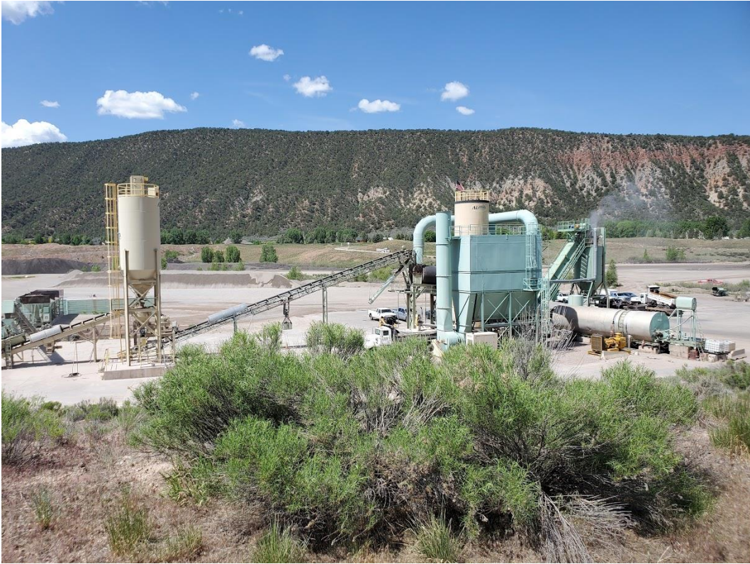
Photo 4: View to the west of hot plant on site.
