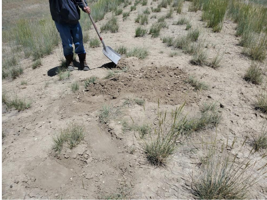
Photo 9: View to the east of filled animal burrow on embankment of RP-4 Pond
