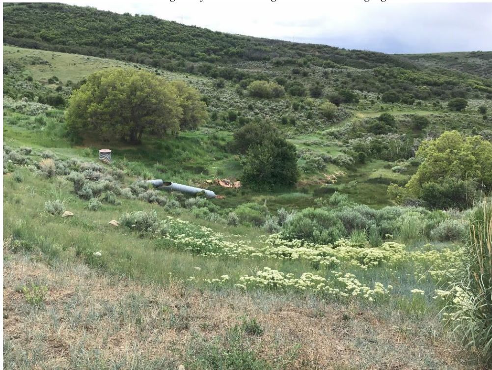
Photo 8: Pond 6 drainage way and discharge culvert discharging clear water.
