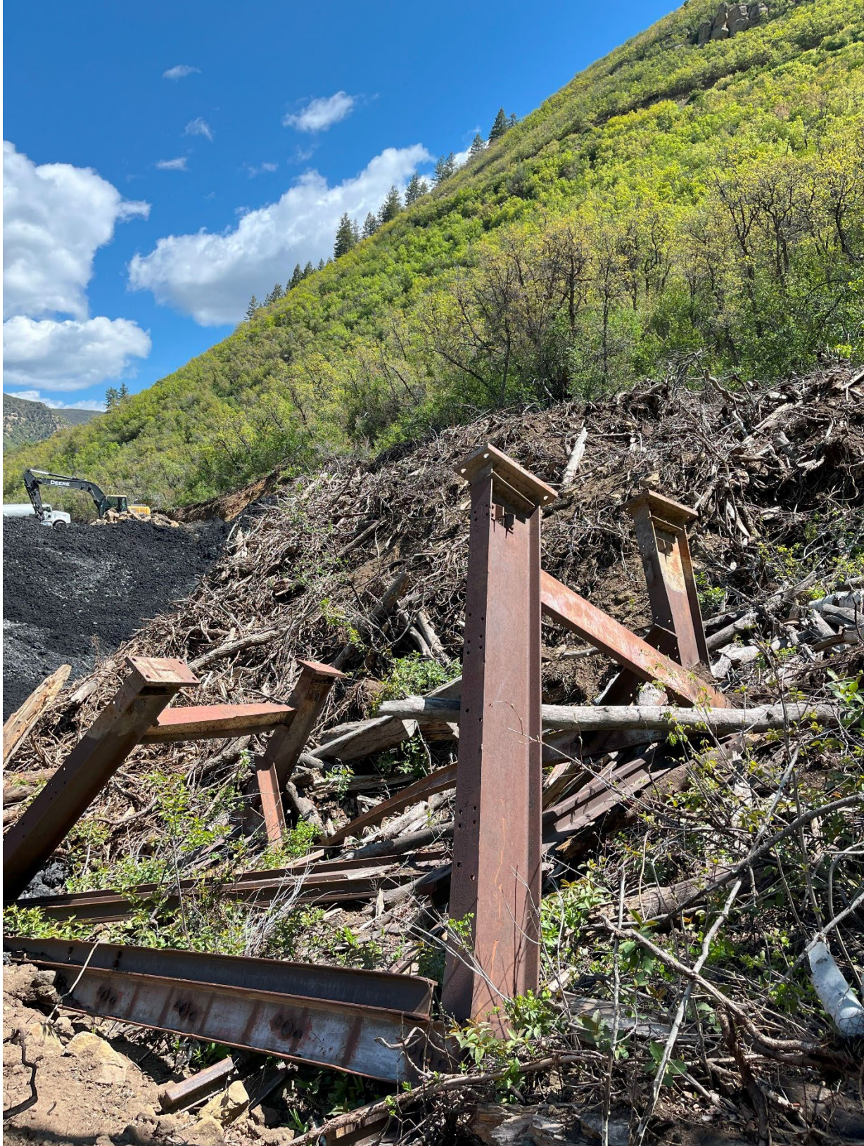
Figure 4 - Active coal refuse work encroaching on a slash pile and I-Beam metal on RPEE. These should be removed before they are buried.
