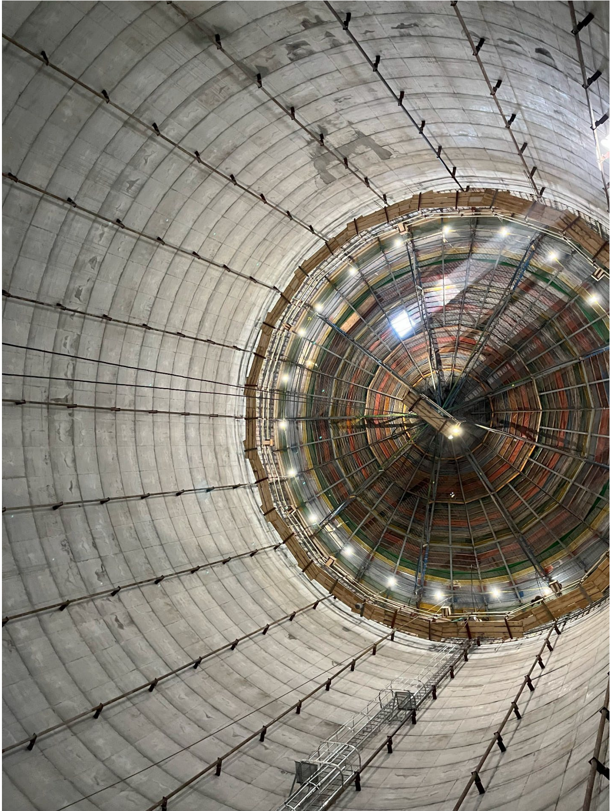
Figure 2 - A silo being repaired.
