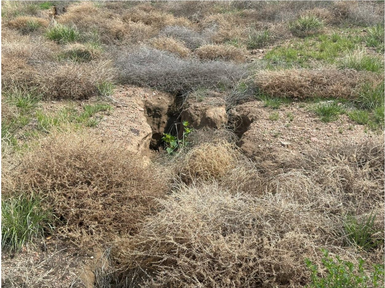
Photo 17. Erosion gully in buttress
