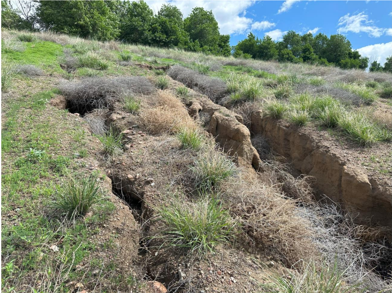
Photo 14. Erosion gully in buttress
