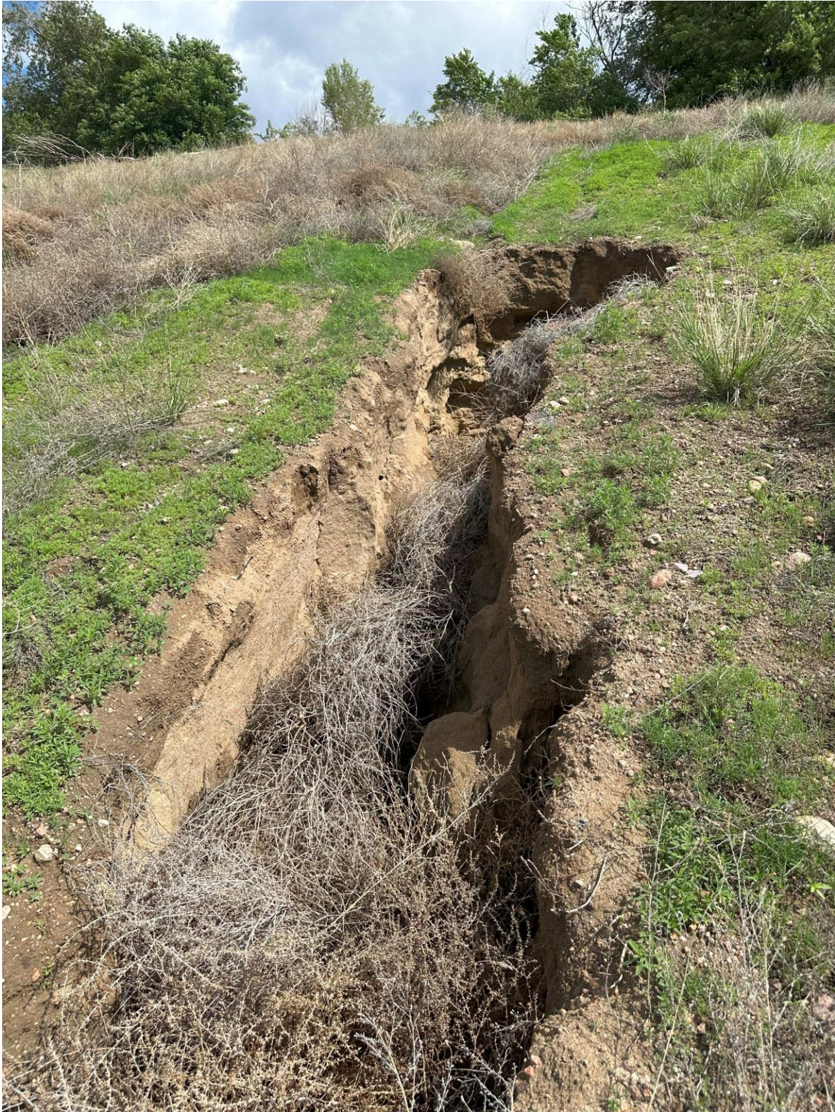
Photo 23. Erosion gully in buttress
