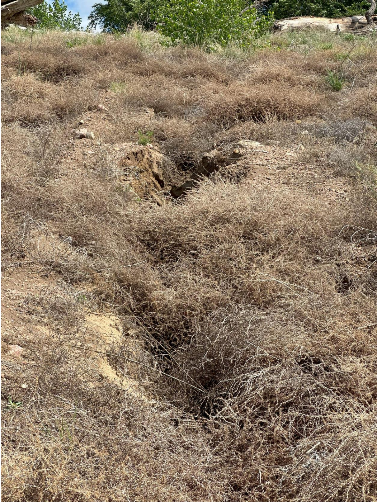
Photo 19. Erosion gully in buttress
