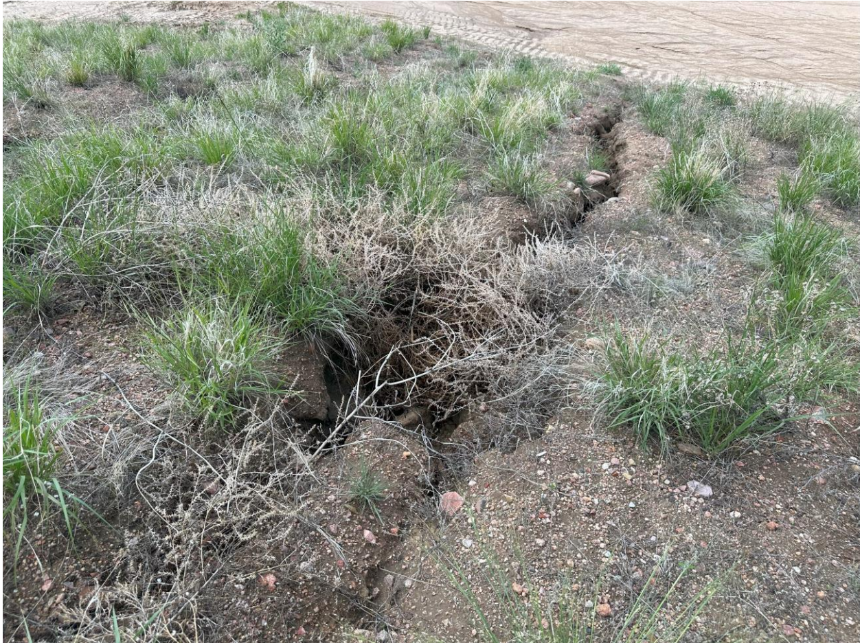
Photo 8. Erosion gully in buttress
