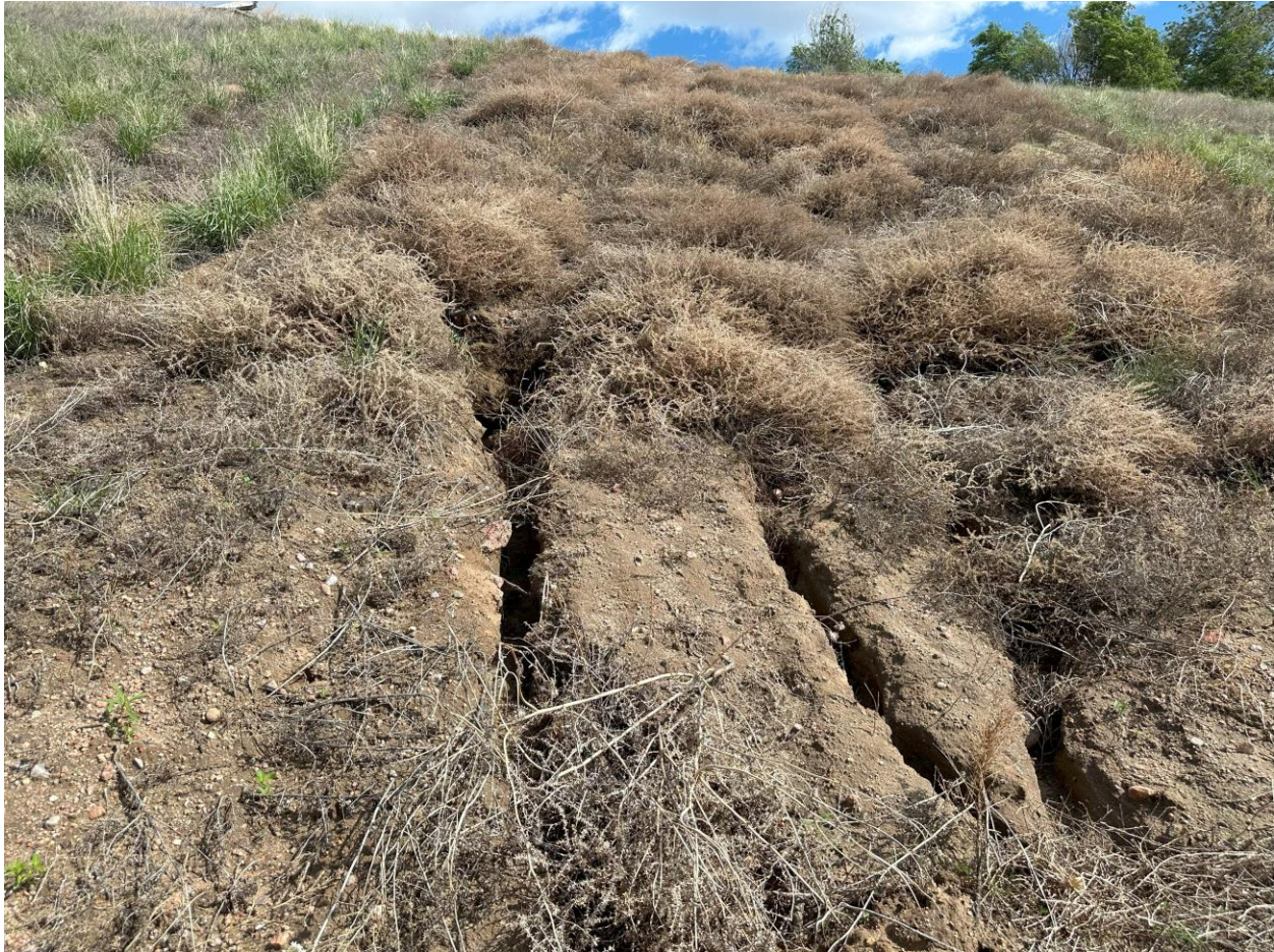
Photo 10. Erosion gully in buttress
