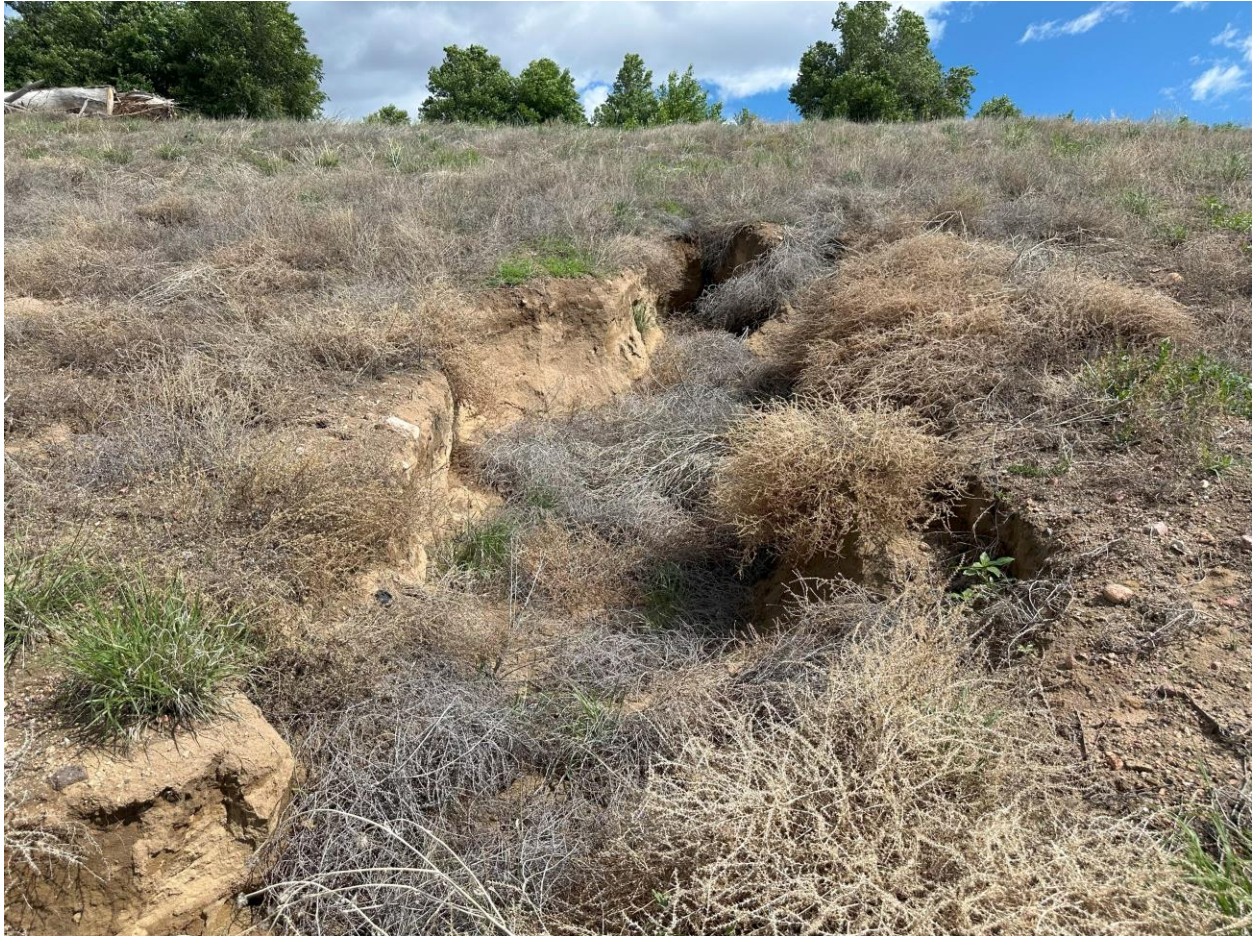
Photo 21. Erosion gully in buttress
