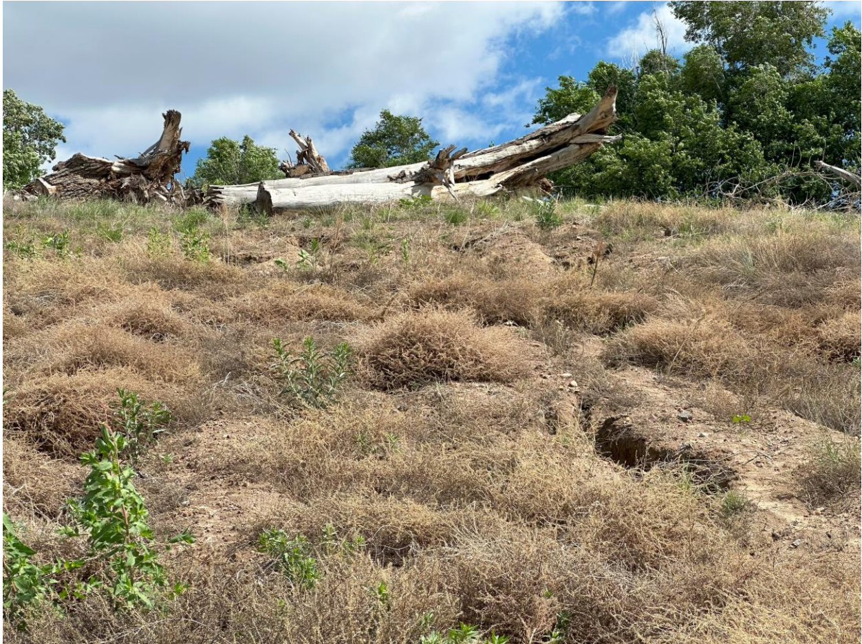
Photo 18. Erosion gully in buttress
