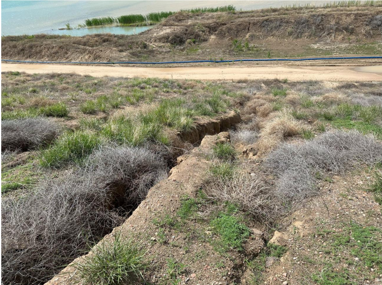
Photo 4. Erosion gullies in buttress
