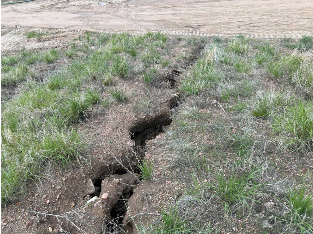
Photo 9. Erosion gully in buttress
