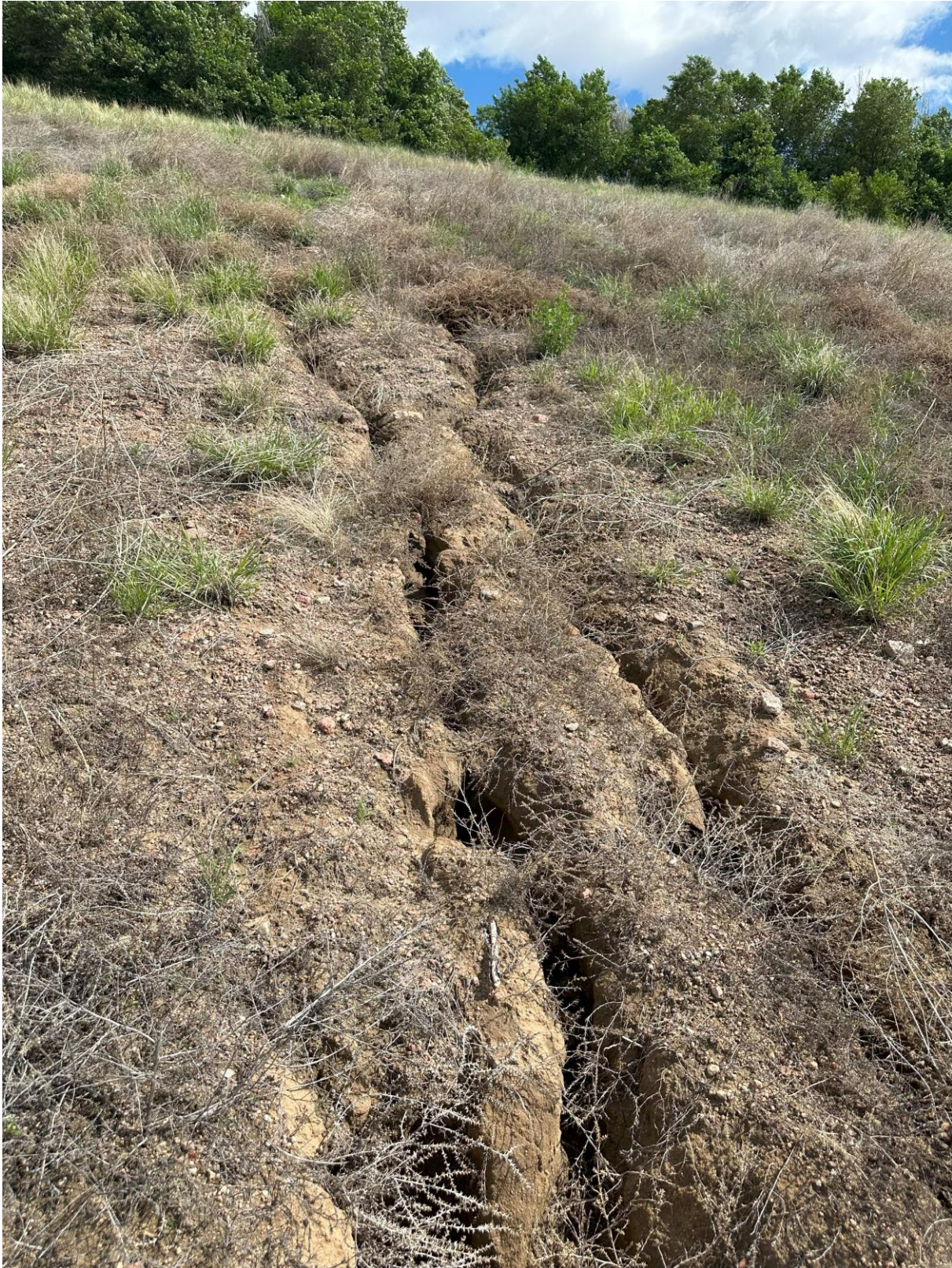
Photo 15. Erosion gullies in buttress
