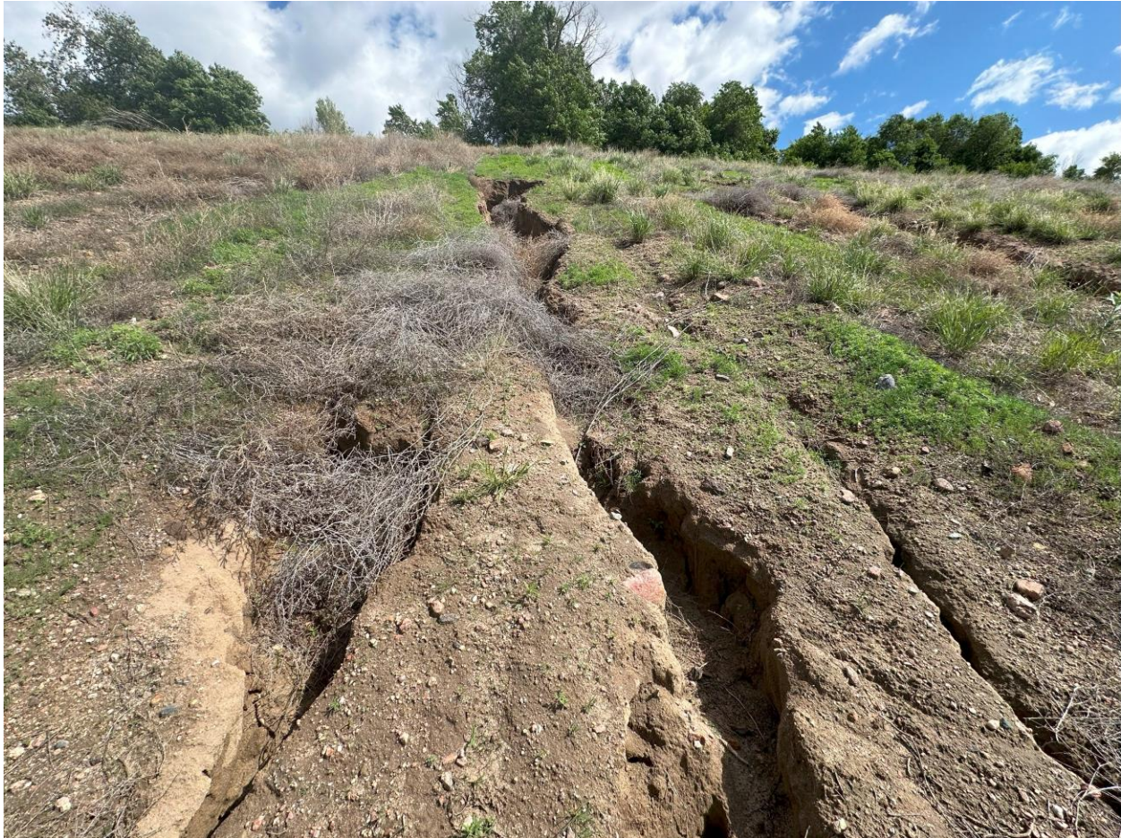
Photo 13. Erosion gully in buttress
