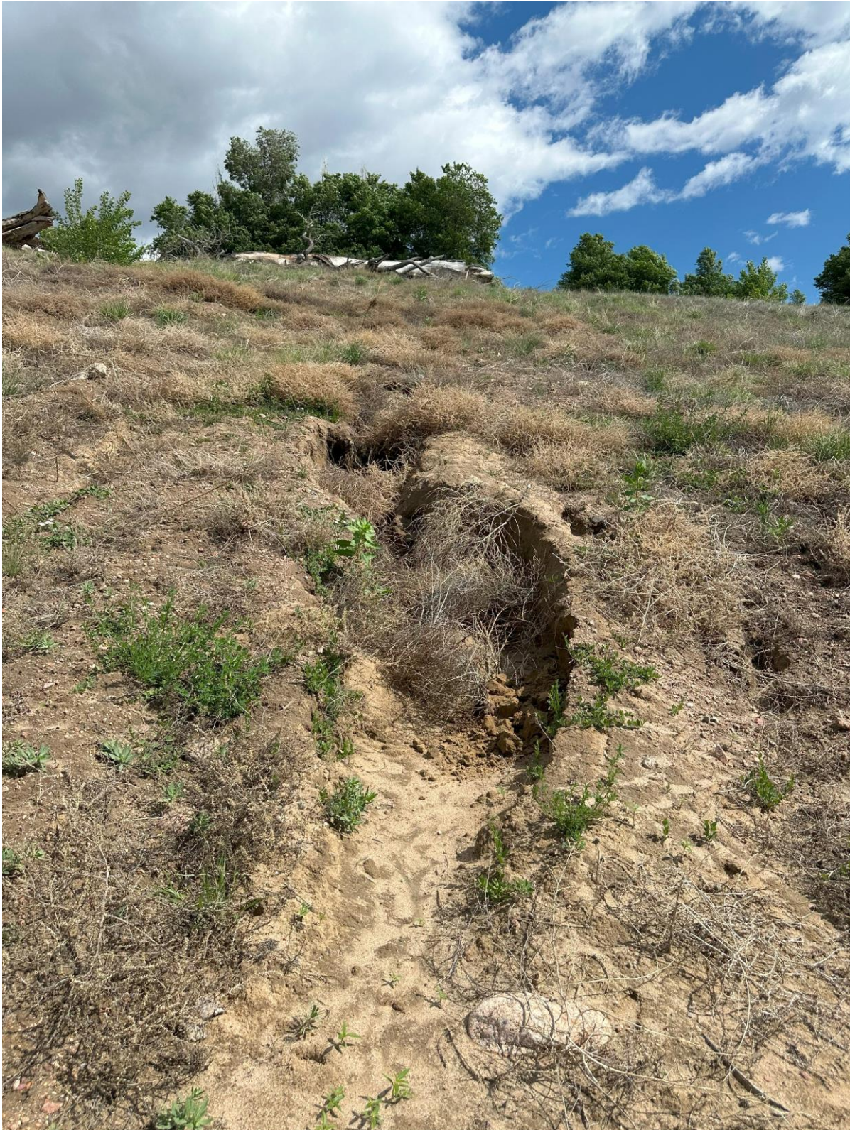
Photo 20. Erosion gully in buttress
