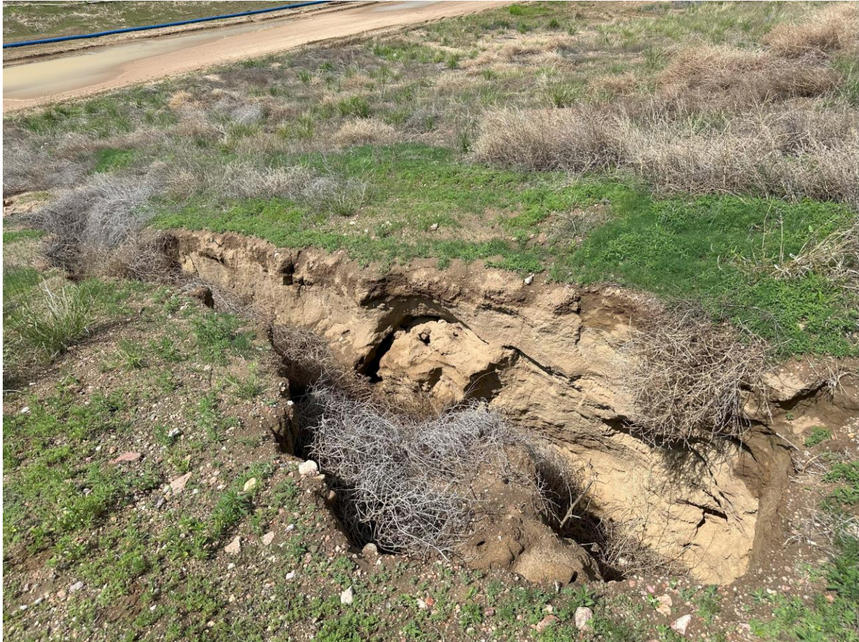
Photo 22. Erosion gully in buttress
