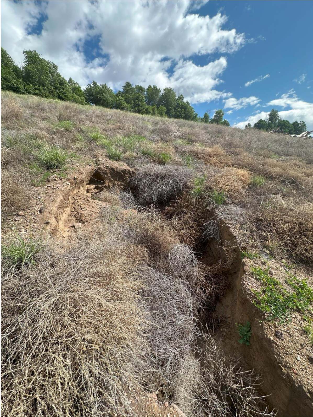
Photo 16. Erosion gully in buttress
