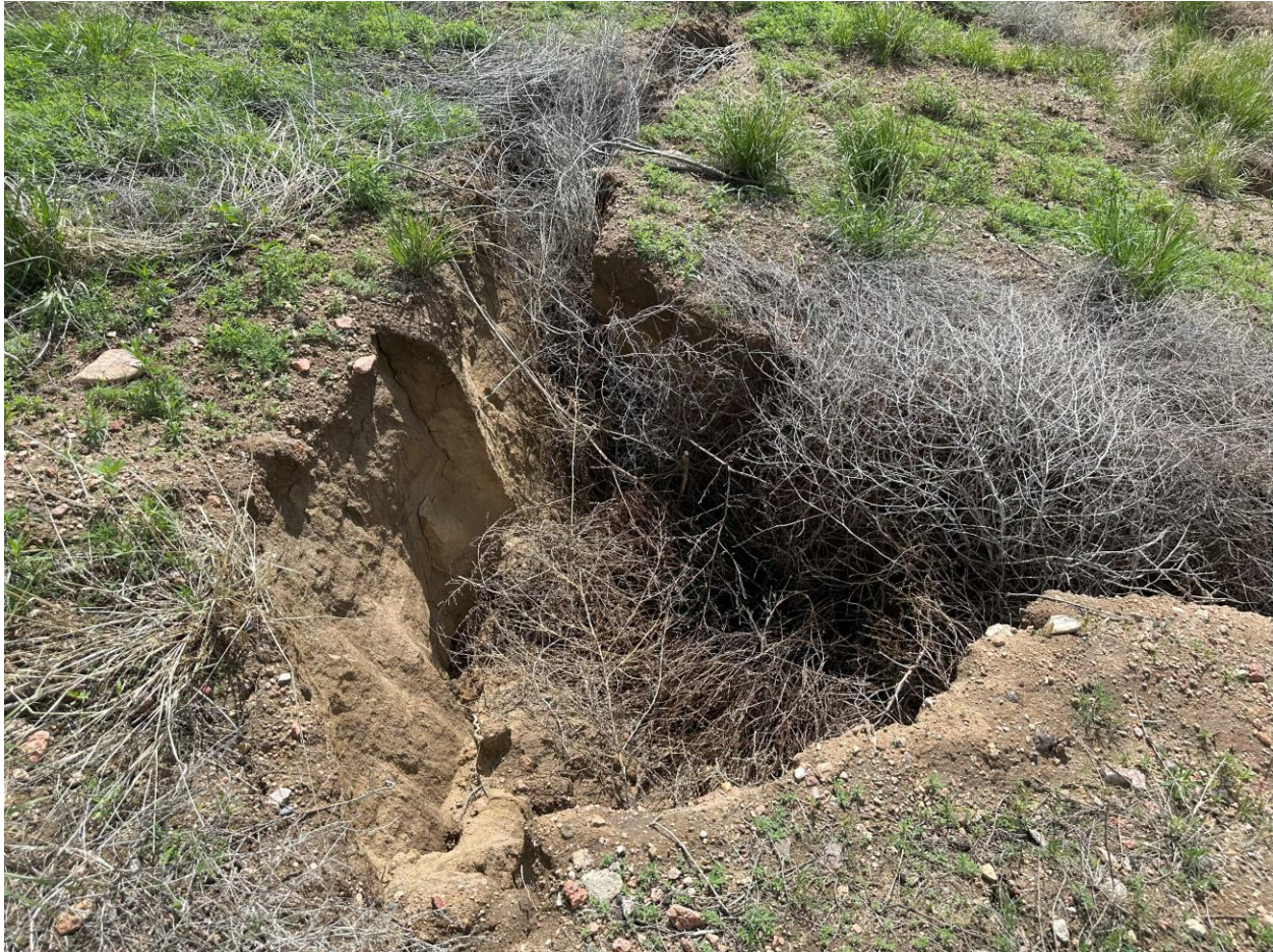
Photo 3. Erosion gully in buttress
