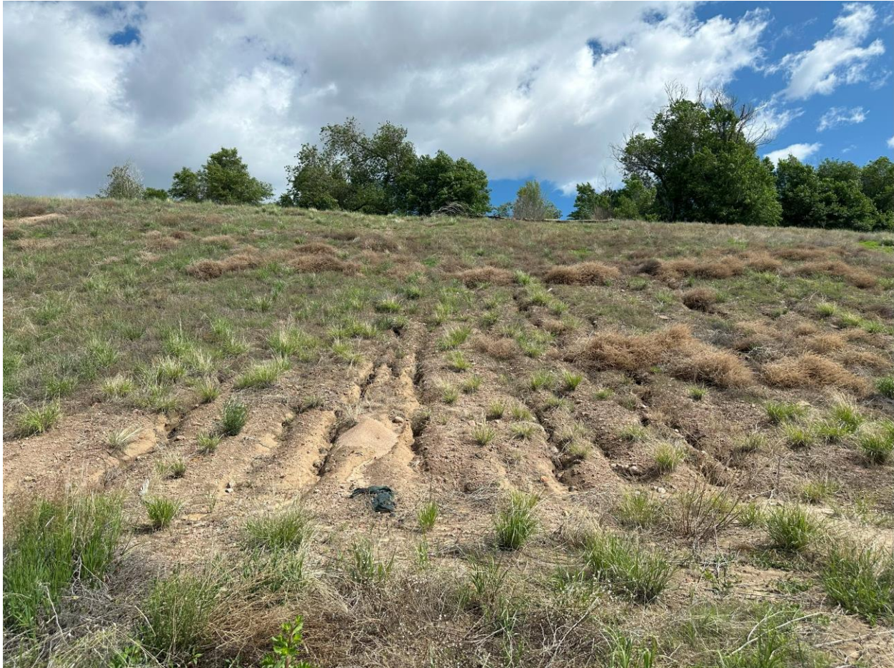
Photo 12. Erosion gullies in buttress
