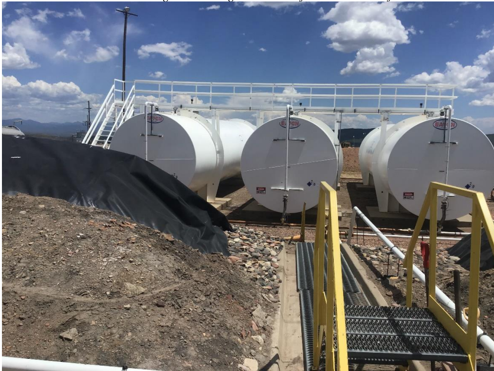
Photo 4: Fuel tank storage containment adequately maintained.
