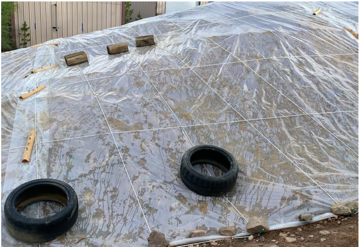
Tails – Close Up View Showing Cover Placement Method (Ropes & Ballast Materials)
