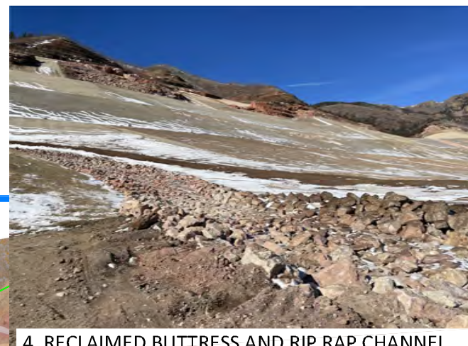
4. RECLAIMED BUTTRESS AND RIP RAP CHANNEL.
