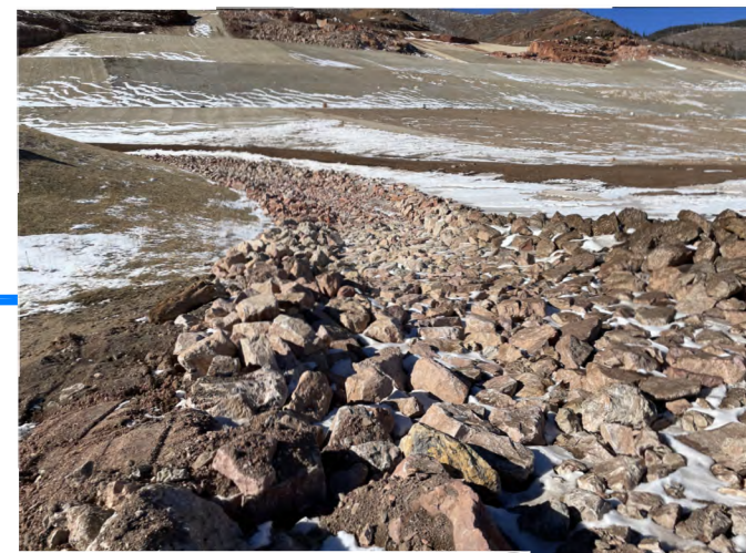
3. RIP RAP LINED MAIN CHANNEL.
