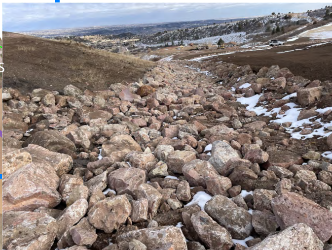
2. RIP RAP LINED MAIN CHANNEL.
