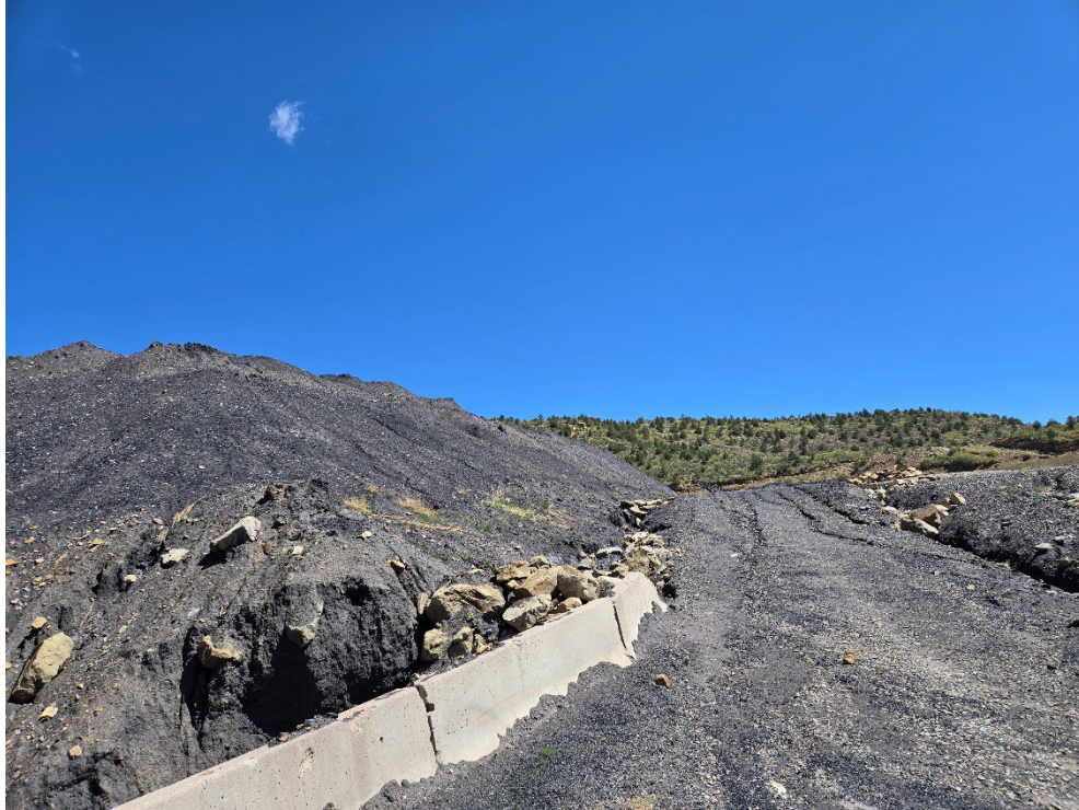
Photo 8: Erosion from the un-reclaimed slope has filled the check dams along the road.
