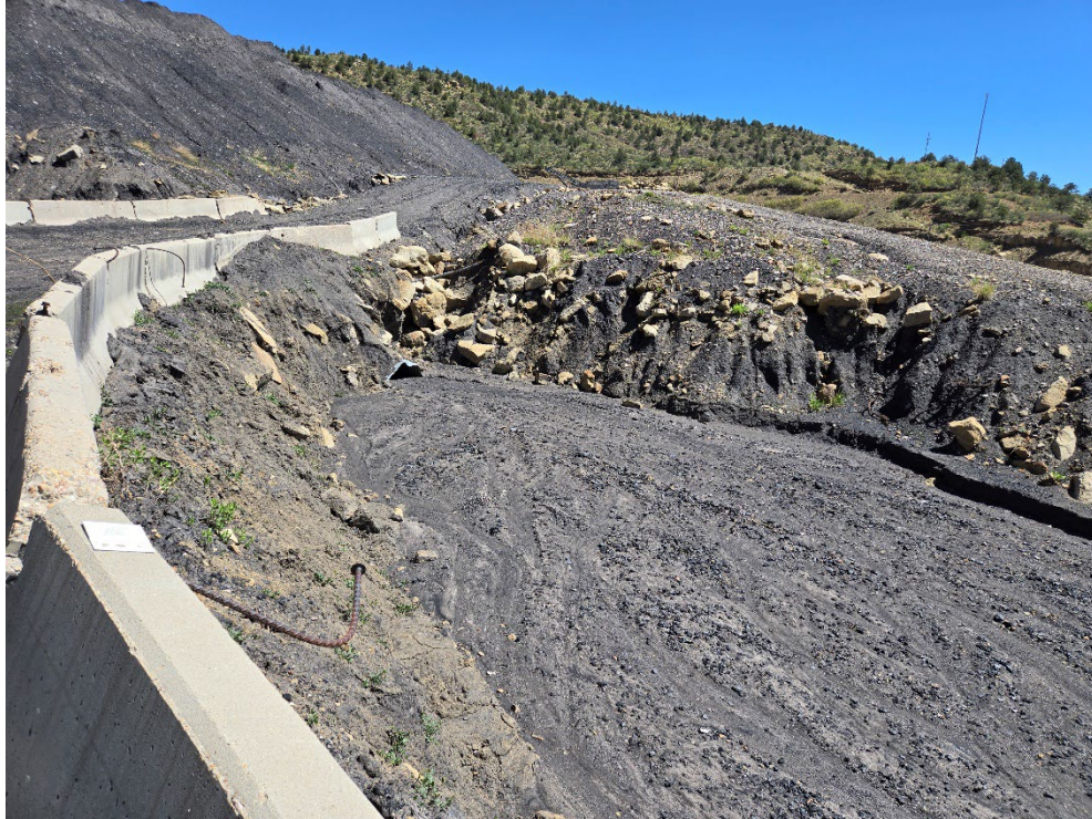
Photo 7: Sediment accumulation at the outlet of culvert C81
