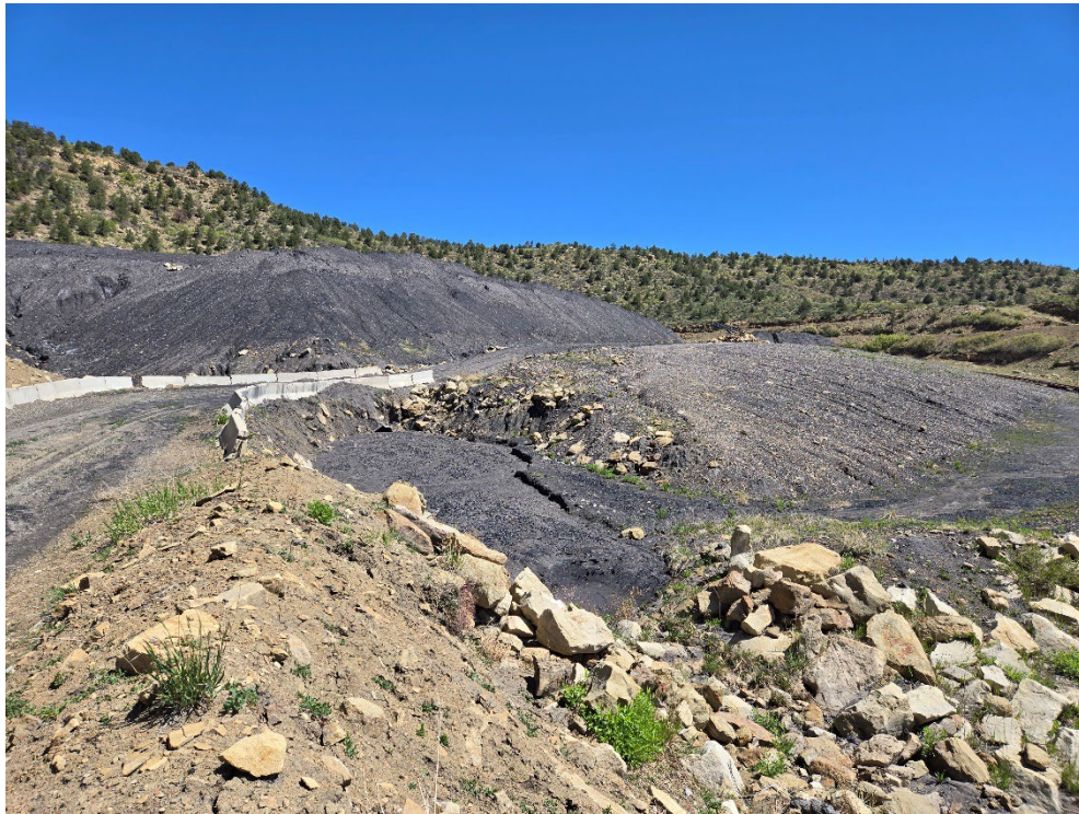
Photo 6: Sediment accumulating at the outlet of C81 from the un-reclaimed portion of the RDA and the ditches on the sides of the haul road.
