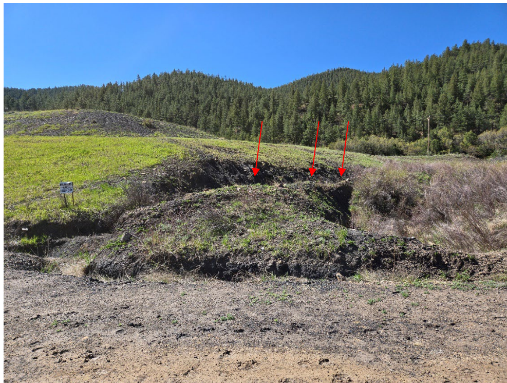
Photo 1: The arrow points to the eroding embankment separating the affected land drainage from the adjacent clear water ditch (D7).
