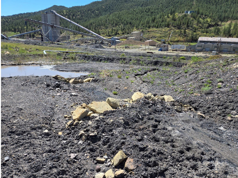
Photo 4: Check dams on the north side of DWDA #2 leading to the sediment basin.
