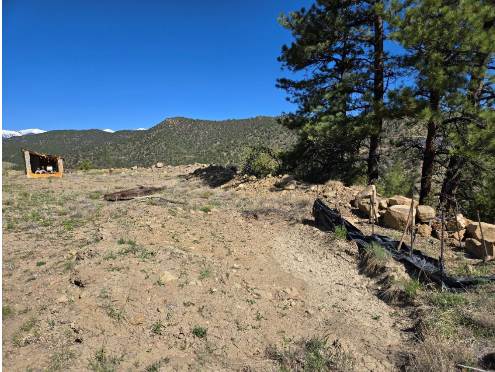
Photo 3: Silt fence within S.A.E on the south side of the permit and the damaged water valve structure in Maintenance item #10 below.
