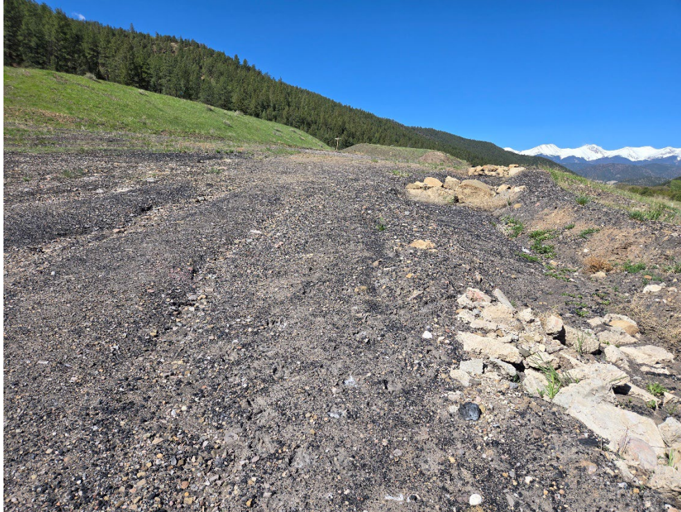
Photo 5: Check dams along the north side of the soil storage area.
