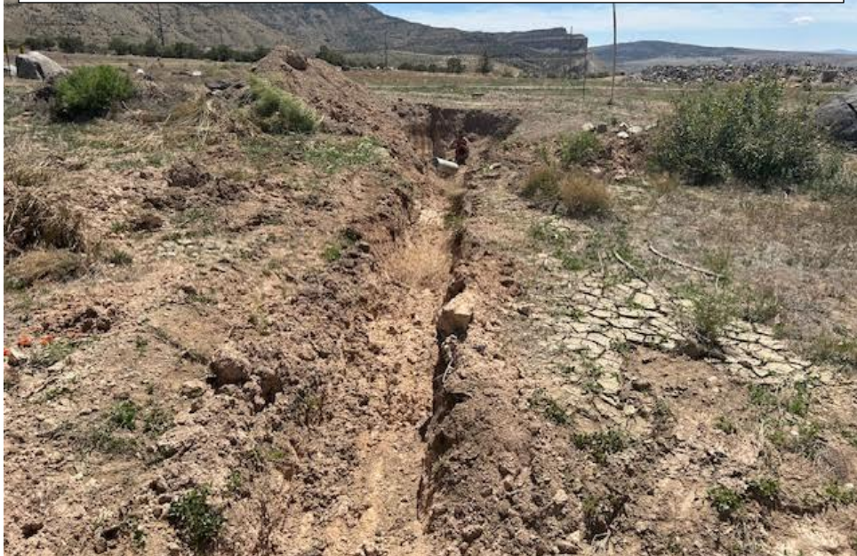
Photo 2: The trench connecting the Carey Pit to the landowner's buried pipeline.
