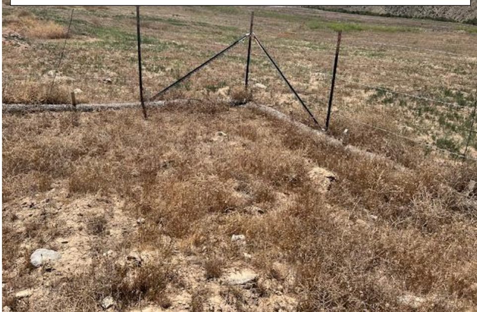
Photo 6. The connection of the southern and western straw waddles at the TR-69 Repair Area disturbed area boundary.
