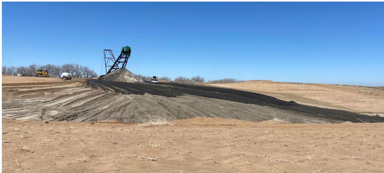
Figure 4.2: Stockpile Development Constructed from Cyclone Underflow
