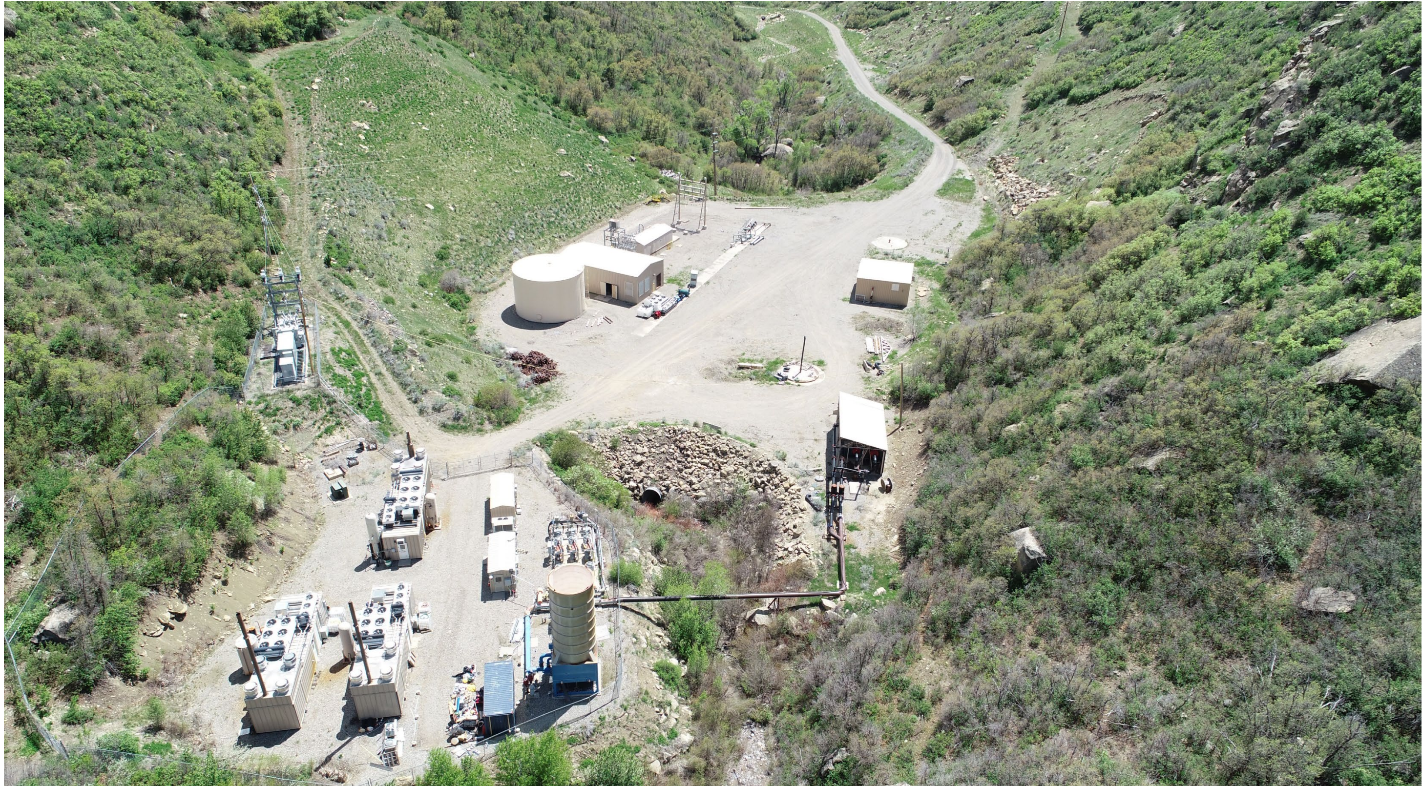
Figure 7: Upper facilities pad
