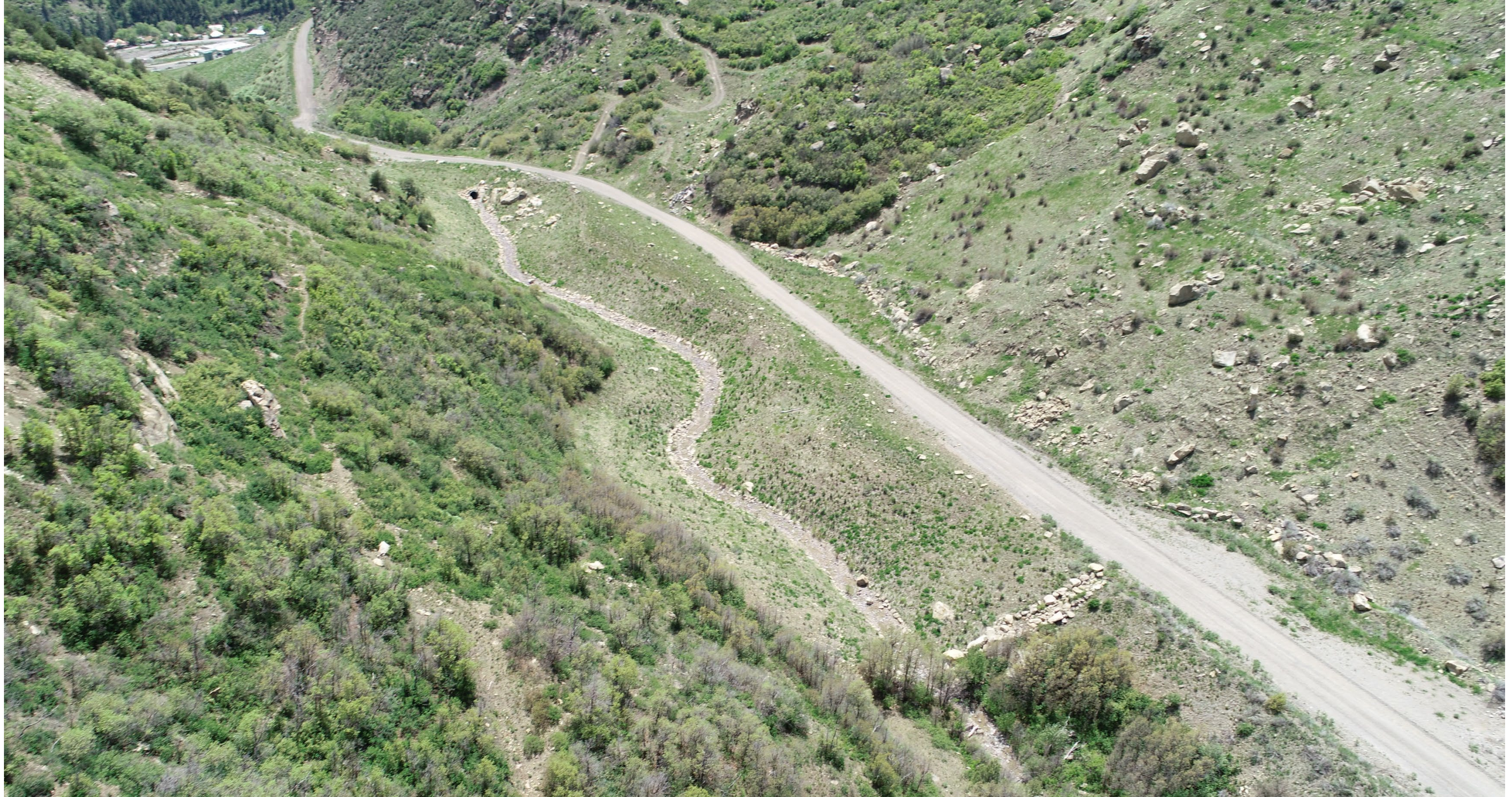
Figure 8: (Reclaimed) middle facilities pad, with reconstructed Elk Creek channel
