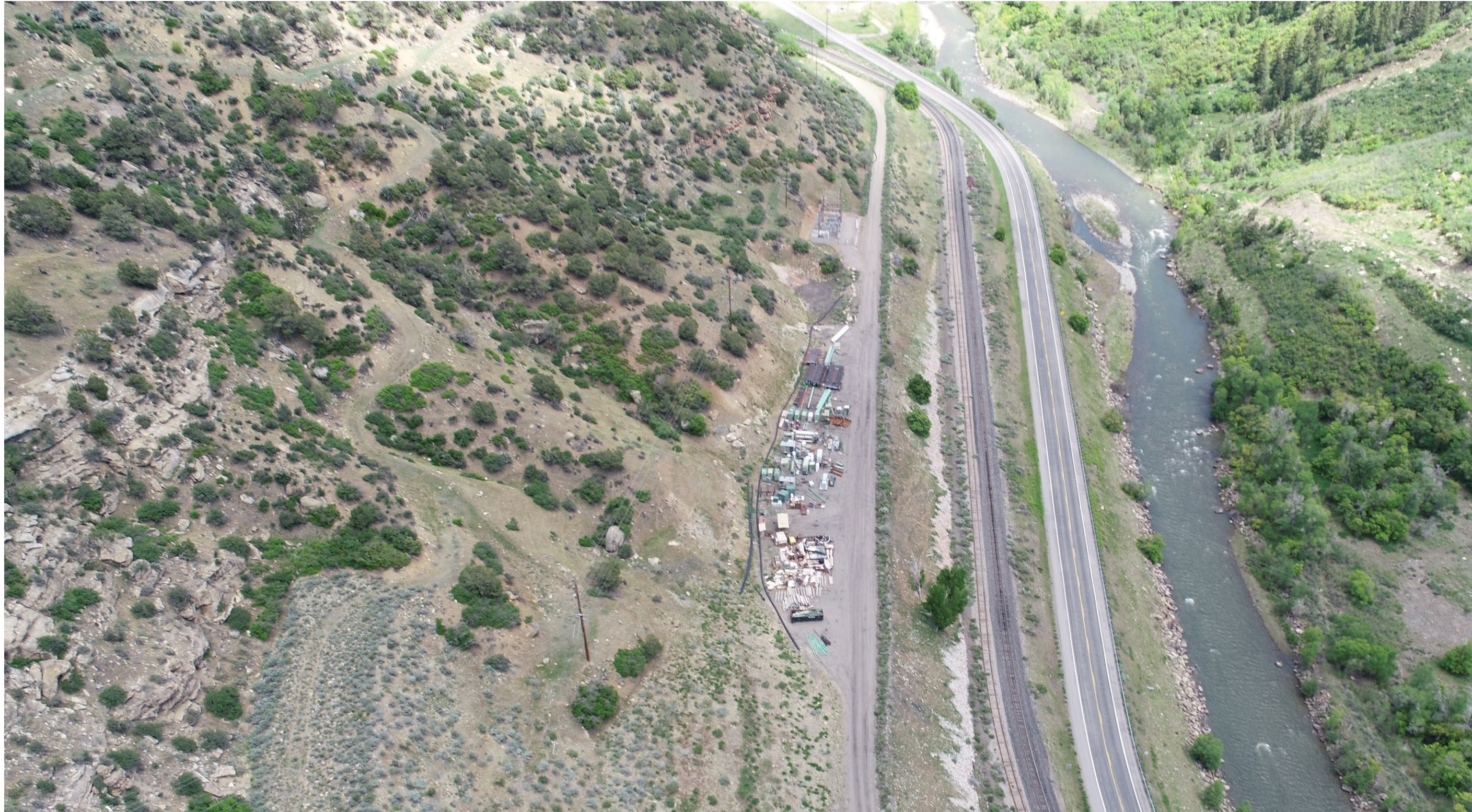
Figure 12: Equipment belonging to Gunnison Energy stored at East Yard
