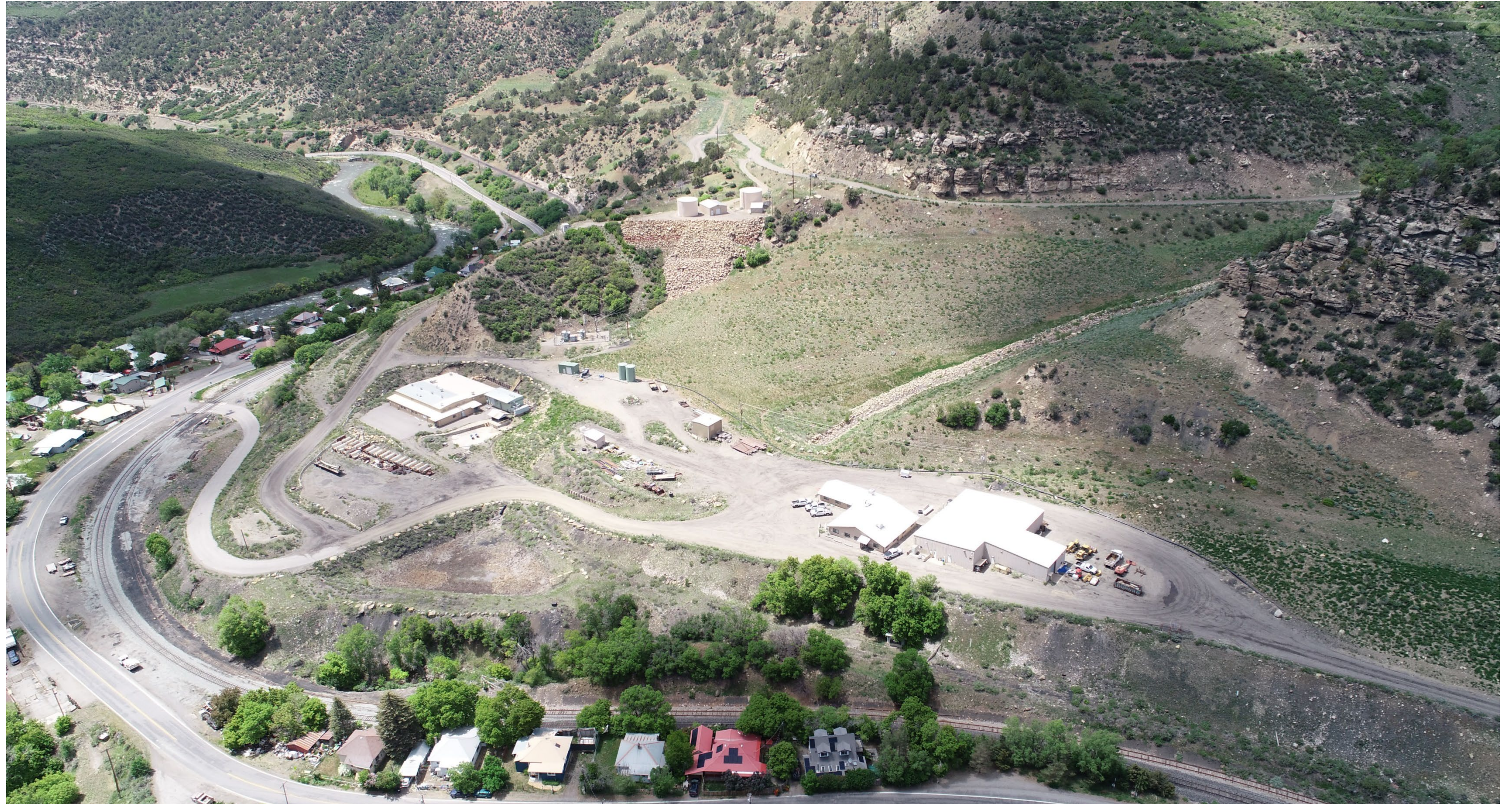
Figure 6: Lower facilities area
