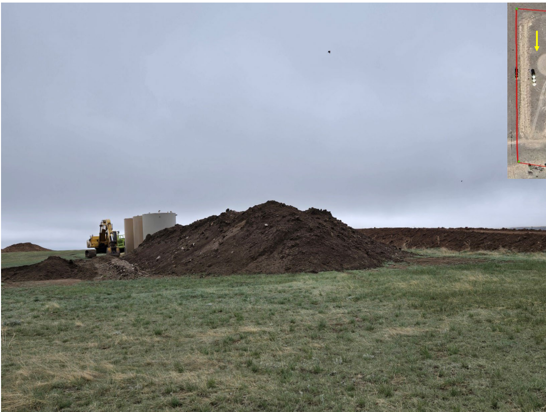
Photo 10: New topsoil pile east of the stabilized pile. The Operator shall ensure this pile is stabilized and seeded if not used for reclamation within one growing season.
