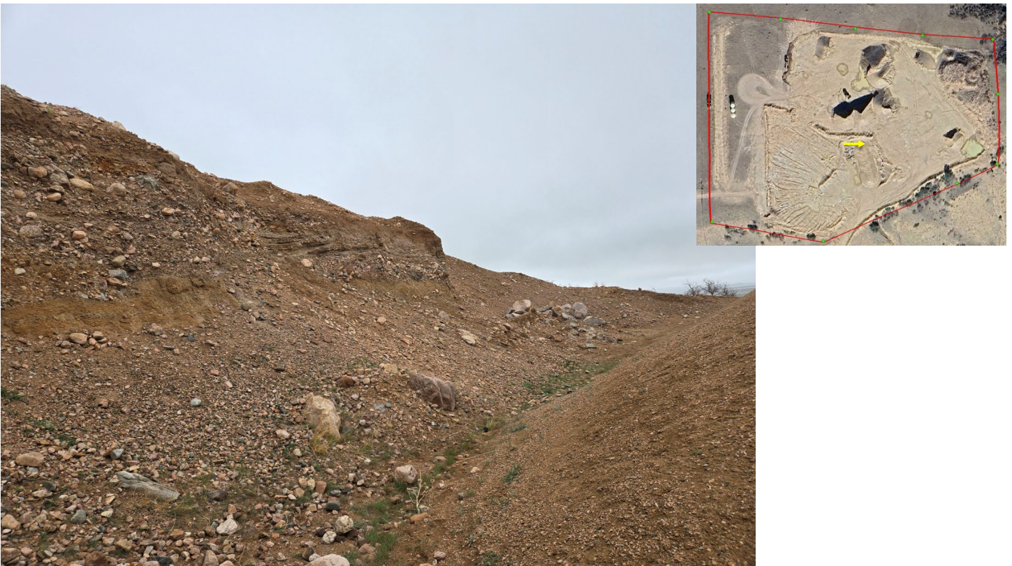
Photo 14: Looking south along the section of highwall within the pit area.
