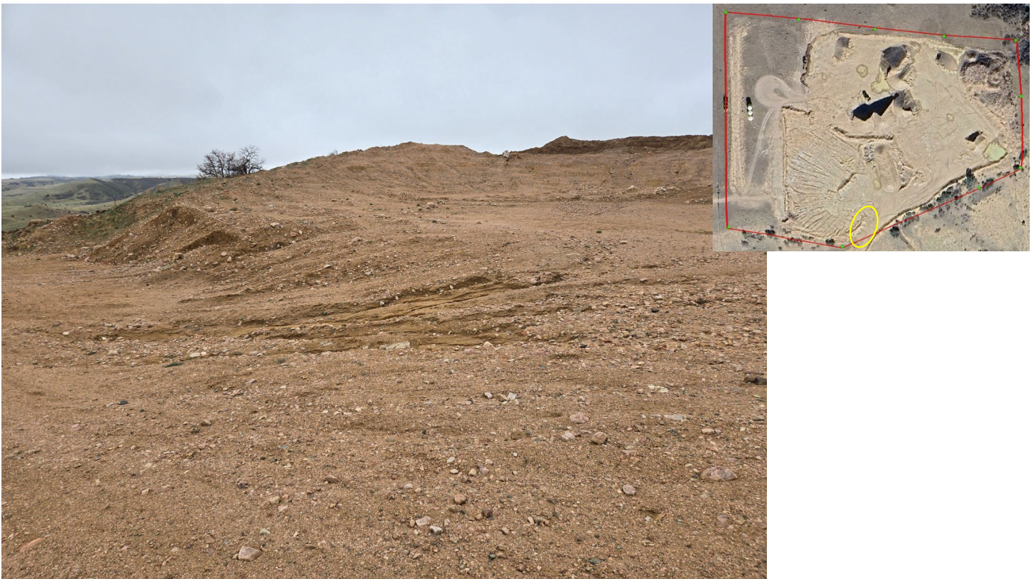
Photo 16: Looking west at the small area near the entrance to the stie where some erosion has begun to form that the Operator shall stabilize.
