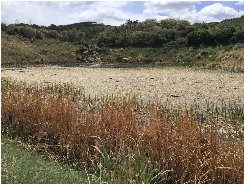
Photo 4: Cattail crop covering East Middle Flume #1 Pond. Inflow channel requires stabilization.
